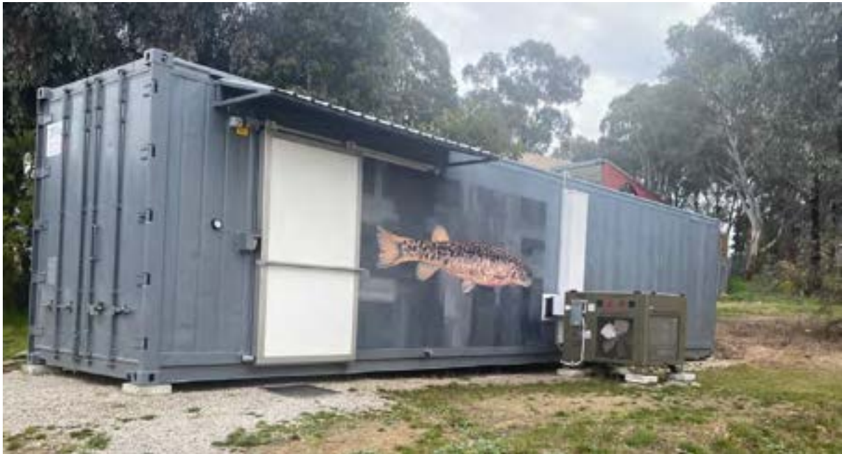
Figure 1. The refrigerated shipping container that the Stocky galaxiids are housed within at Charles Sturt University. The ambient air temperature within the container can be controlled via two sources, the internal refrigeration unit and an external cooler, and can be maintained at temperatures between 2-30° C. The container is also equipped with a backup generator that can run the external cooler and run air into the container.
