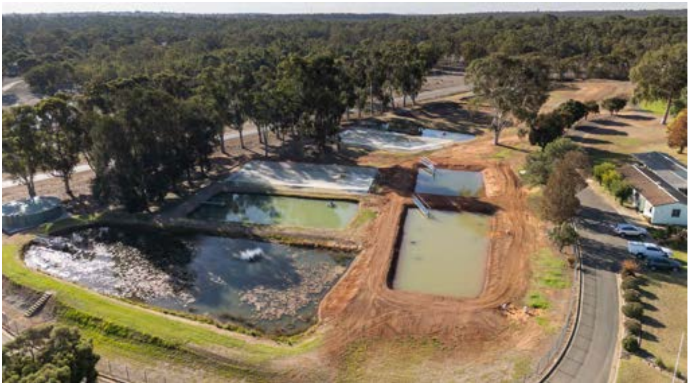
Figure 8. Two newly constructed Office Ponds
