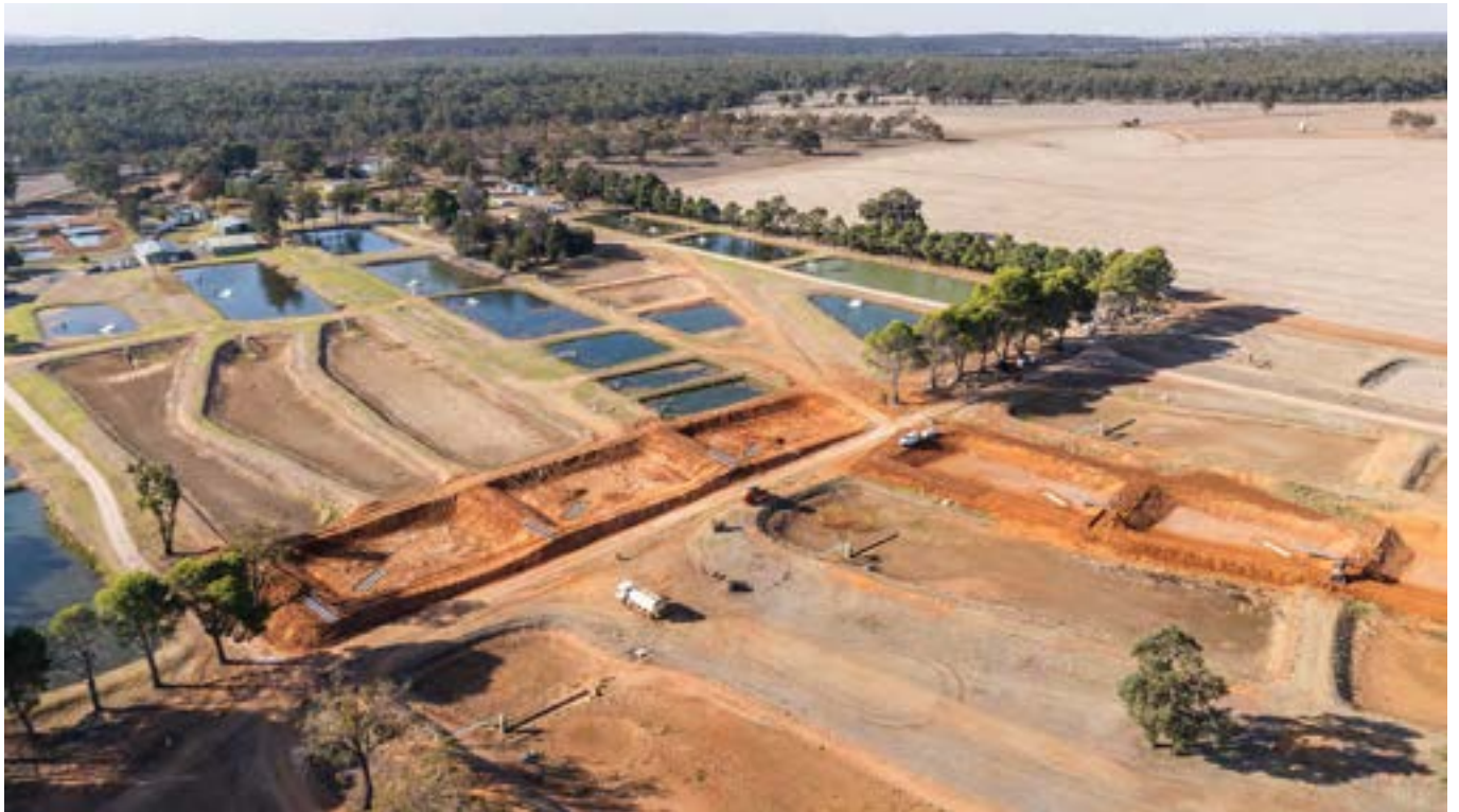
Figure 9. Pond construction on Middle Pines and Between 36-37 nearing completion in the foreground. The completed Office ponds can be seen full in the background.
