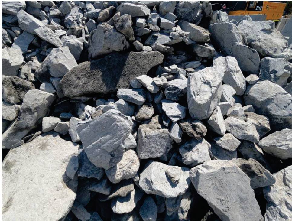
Figure 2-5 Rockfill Material for in Reservoir Placement
