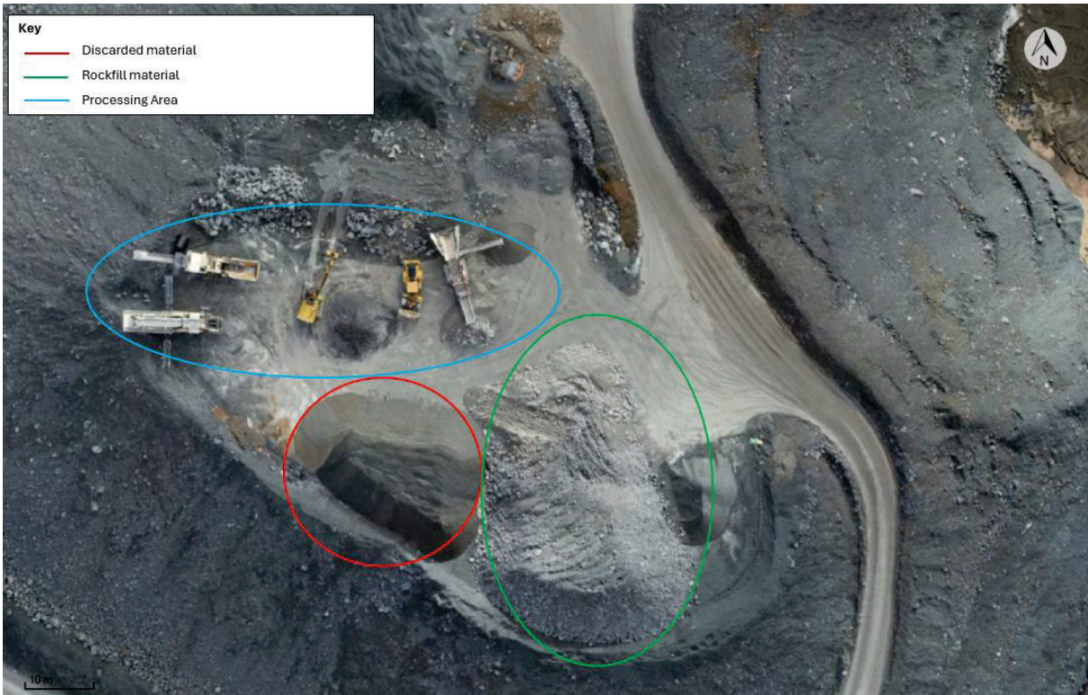
Figure 2-1 Rockfill Processing Area
