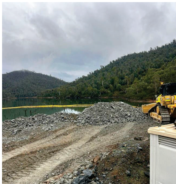
Figure 2-7 Northern Talbingo Rock Platform Work Area
