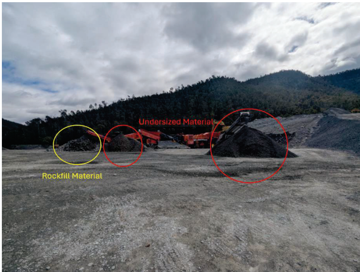
Figure 2-3 Screen and Crusher Setup Showing Removal of Undersized Material
