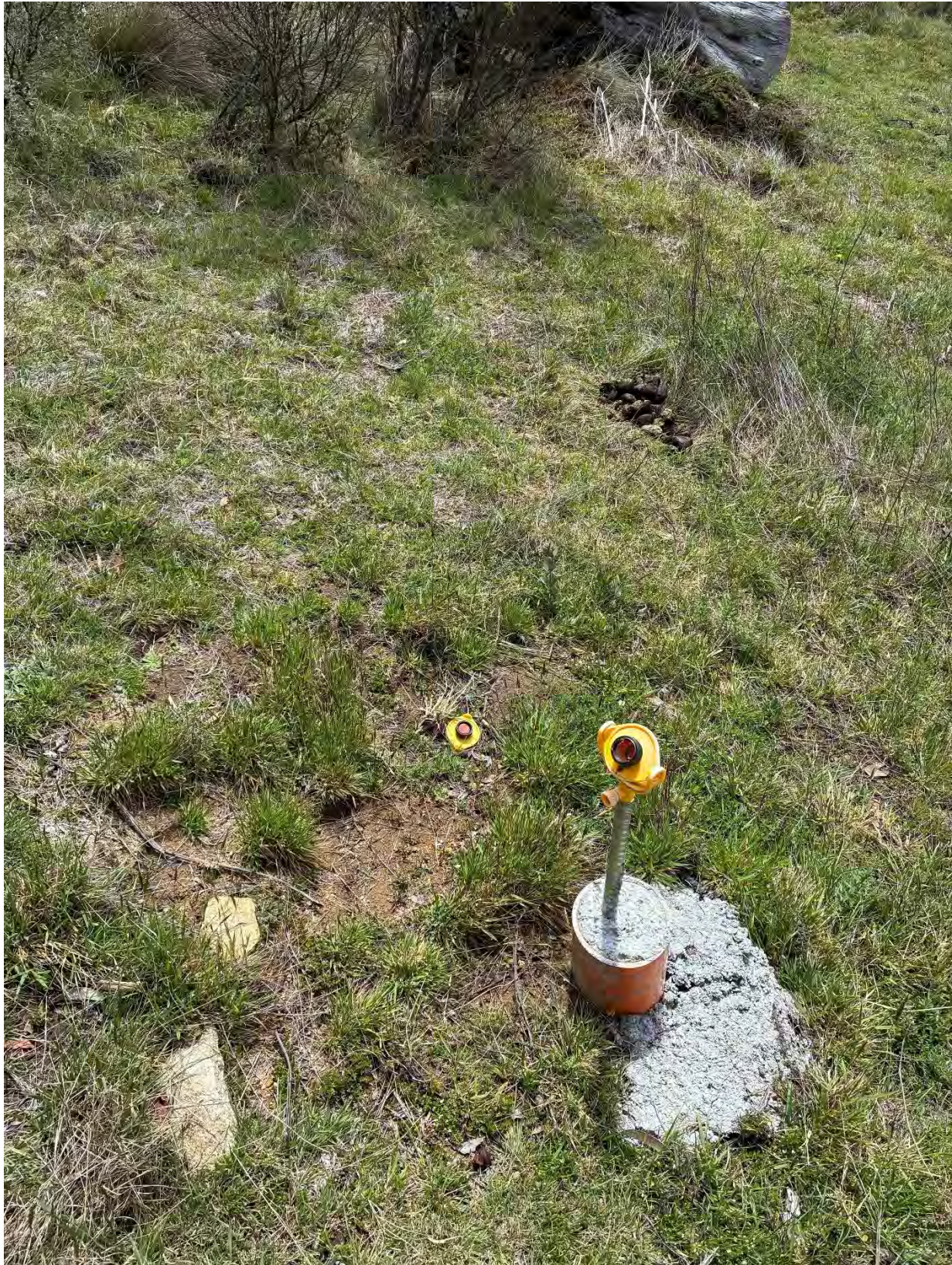
Photograph 7 – Survey Monitoring Point. Note damaged Prism on ground
