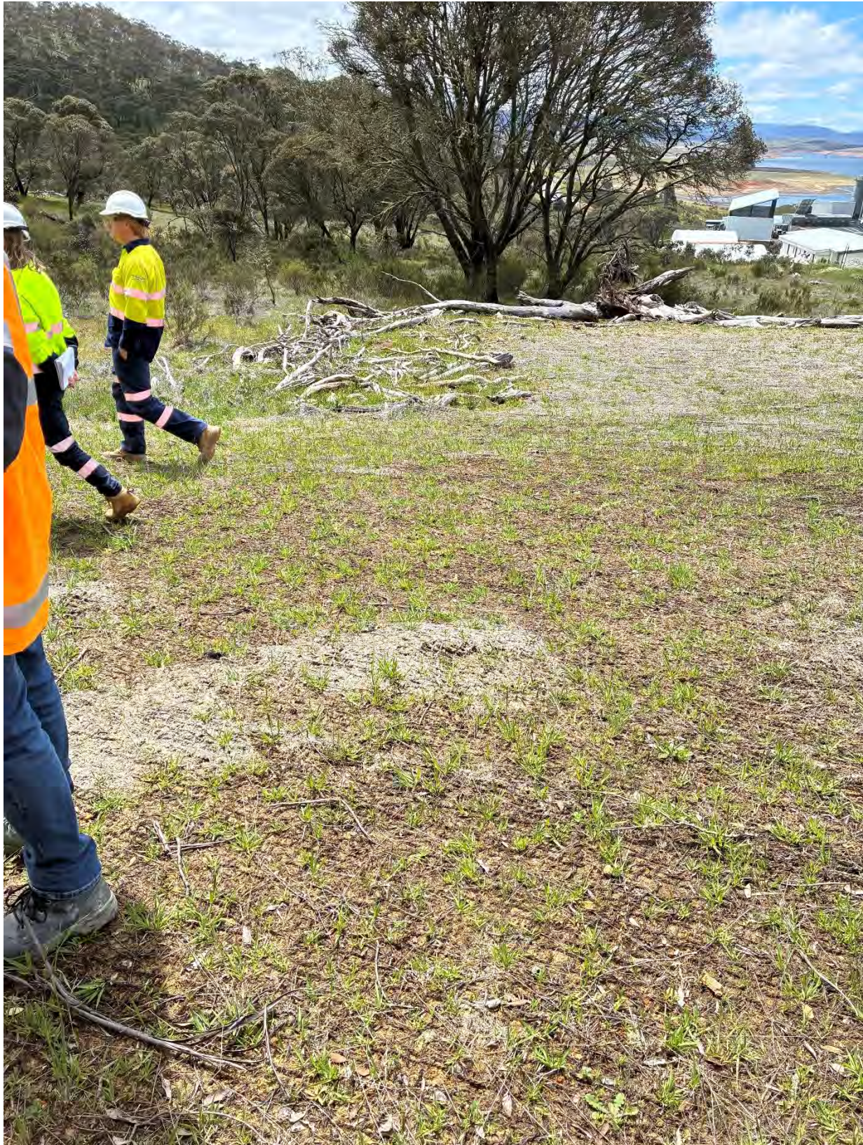
Photograph 2 -Grasses growing on remediated sinkhole. Note ground covered in jute matting as erosion protection
