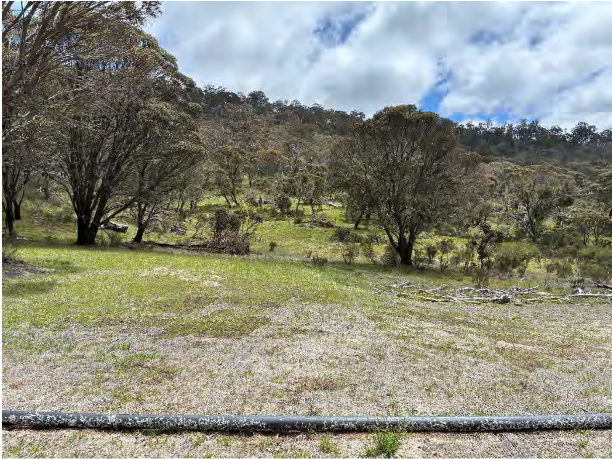
Photo 1 – General view of the former sinkhole looking west along the approximate line of the tunnel. Footprint of remediated sinkhole in foreground covered with jute matting
