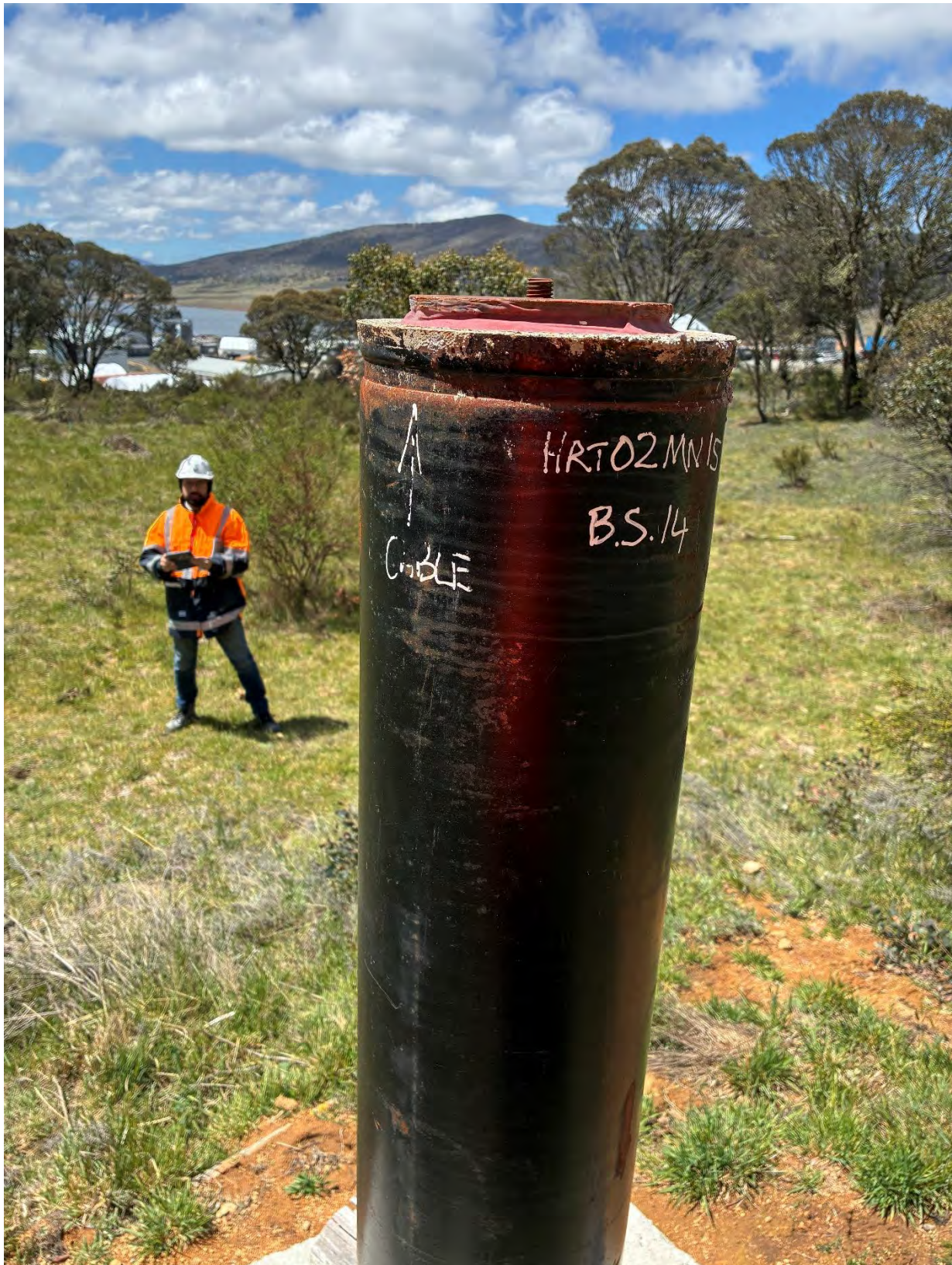
Photograph 9 – Survey Station detail
