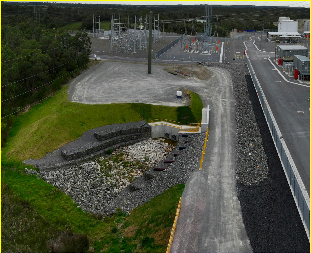
Figure 6.2b: Location of KKPS penstock valve and stormwater discharge outlet
