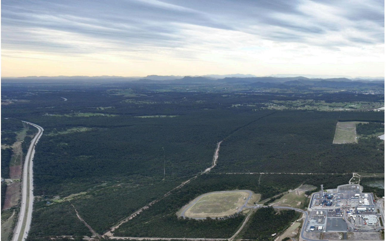
Figure 4.3: KKPS proximity to bushland
