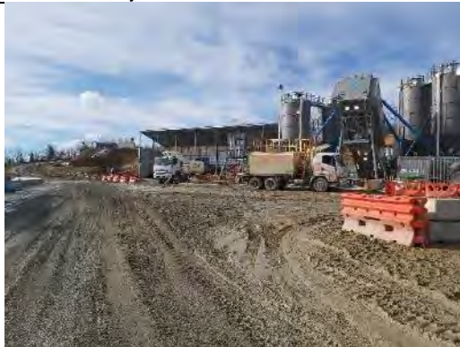
MC32: MC233: Marica Surge shaft – aggregate bins – materials used at the concrete batching plant
