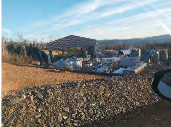
MC28: Marica Surge Shaft building
