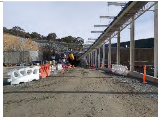
TT24: 3 Tantangara Adit Portal
