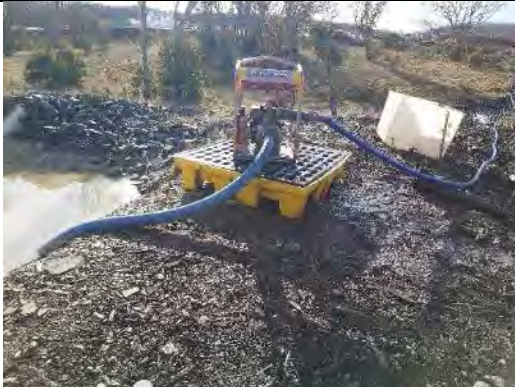
MC24: Dewatering operations at MC03 near Marica Camp. Water was leaking from a hose fitting and overtopping the bund. Dewatering permit was one day out of date (OBS)
