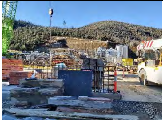
LH 36: Talbingo Adit TBM location
