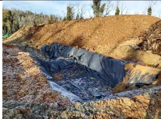
MC19: Concrete washout area – Marica West trail
