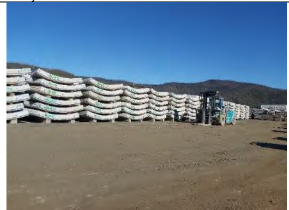
LH 9: Storage tunnel segments on Pad 50 at Main Yard
