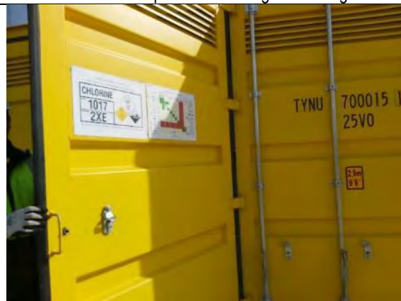
TT31: Container – chlorine storage.
