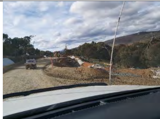
TT41: Sediment sumps along Spoil Road
