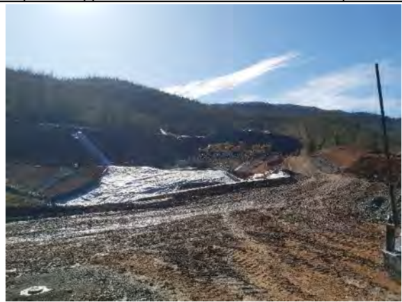
LH 28: View to GF01 – leachate basin in foreground, spoil stockpile on left, diversion drain / access track on right.
