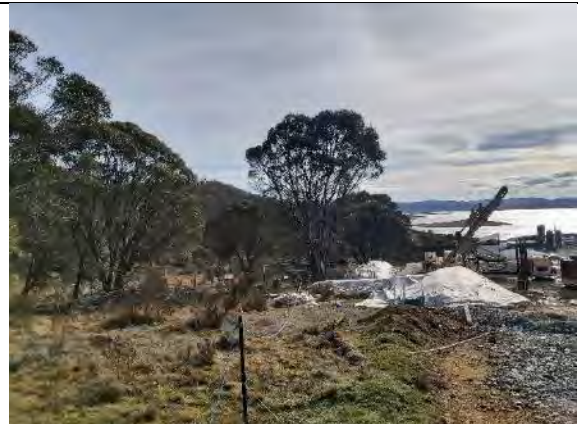
TT21: Sink hole work site. Behind fenced area is outside EIS boundary (no entry sign on fence). Drilling / grouting works to stabilise area around the sinkhole.
