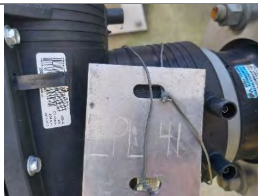
LH 42: EPL point correctly labelled on apparatus
