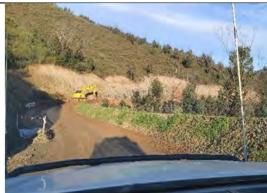
LH 44: Berms stabilised and seeded LHRR North, drain protected
