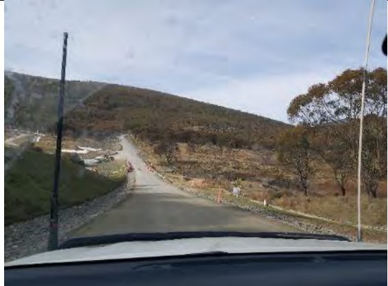
TT12: Stabilised verges, road surface sheeted with crushed rock / DGB20
