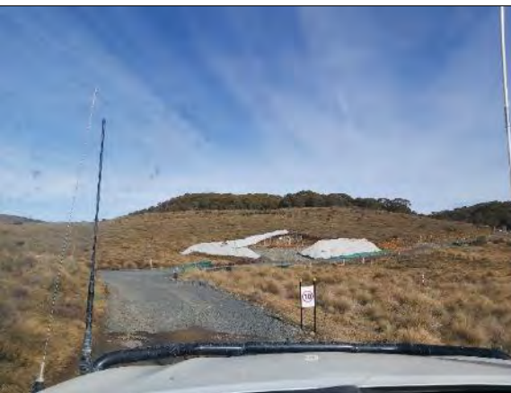
GTS17: Covered stockpiles and stabilised drilling pad area
