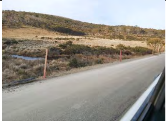
TT3 TT4: Tantangara Creek - Nungar Creek crossing – road in the vicinity has been sealed to prevent / minimise unsealed road runoff / diffuse water pollution as response to EPA regulatory actions
