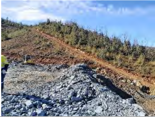
LH 25: GF01 showing water diversion/access trail around spoil area. Has since been upgraded to be a clean-water diversion drain – see next photo.
