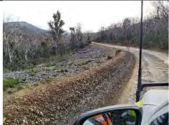
TT2: Tantangara – stabilised berm on road edge
