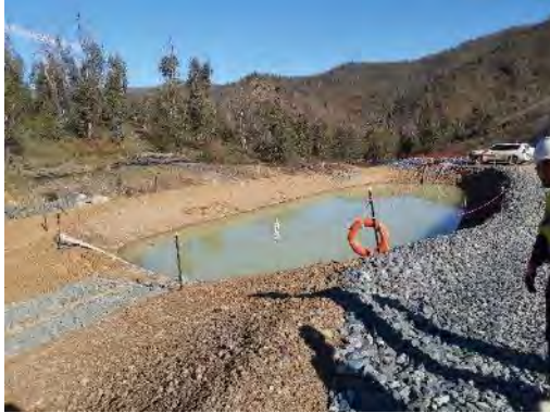
LH 33 Jute mesh and rock –upgraded basin – F10 on low side of GF01
