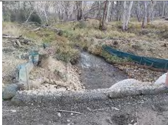
TT5: Unnamed creek feeding into Nungar Creek
