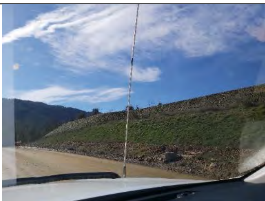
LH 23: Stabilised Batter Pad F
