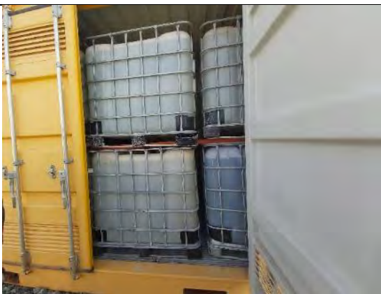
TT32: Chlorine storage inside container
