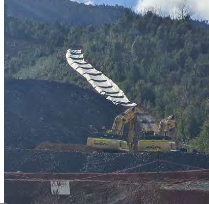
LH 26: Updated photo (31/07/23) of diversion drain. Following a joint agency meeting, a temporary clean water drain is being installed to replace the current access road, as per the approved erosion and sediment control plan
