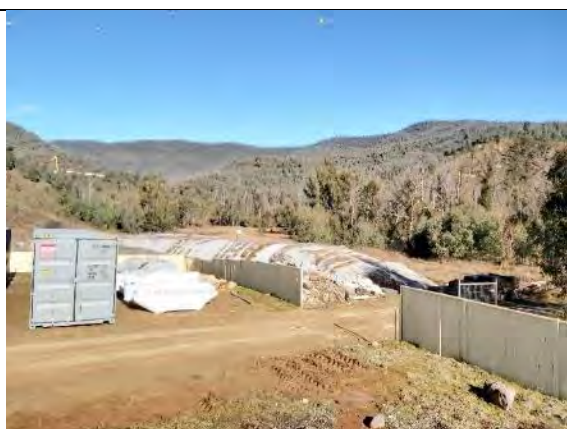
LH 15: Topsoil stockpile – covered, with signage – “Clean topsoil” at Pad 2
