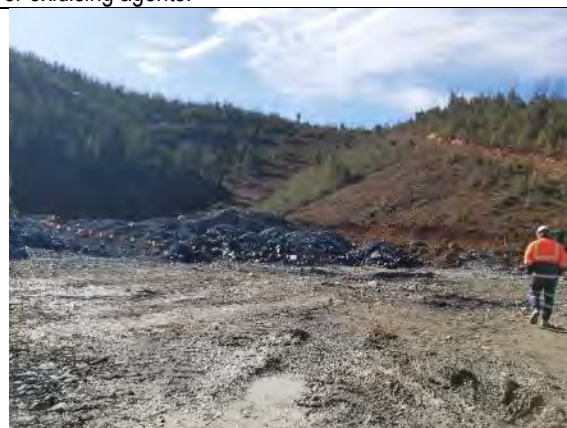
LH 24: Tunnel spoil – PAF storage area – awaiting validation testing prior to blending Sign says PAF UC PAF Spoil – GF01
