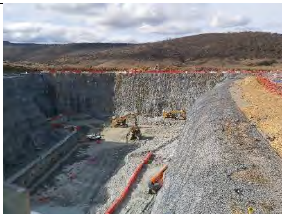
TT33: Tantangara Intake under construction
