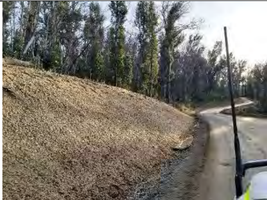
TT1: Tantangara road – Hydromulched batter
