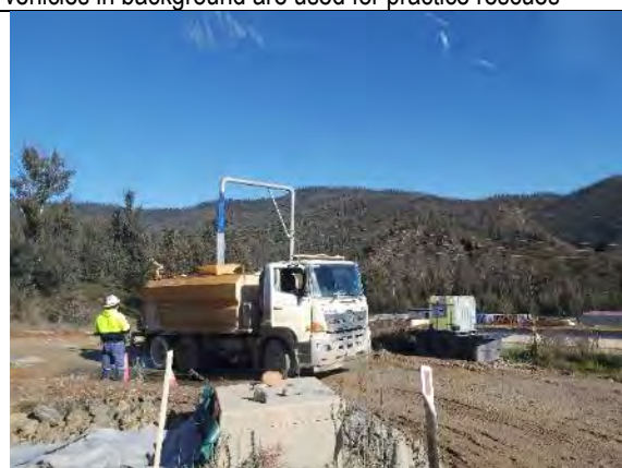
LH 16: Water cart refilling – for irrigation and haul road dust suppression – Pad 2 standpipe
