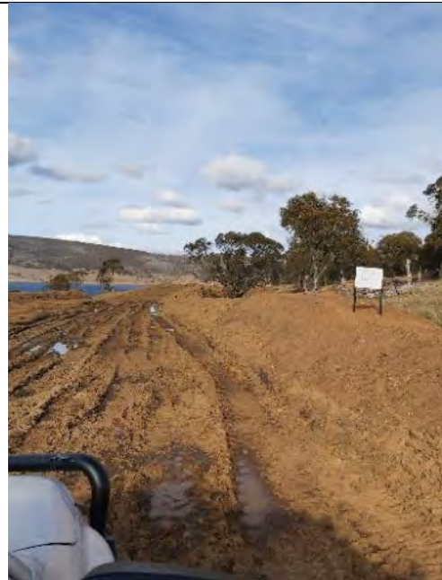
TT47: Topsoil stockpile – for later rehabilitation (recently placed – to be stabilised with stonewall and covered)
