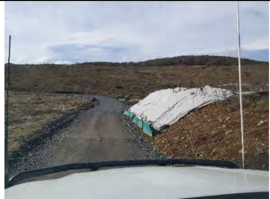
GTS8: Approaching Gooandra Creek – covered stockpile in foreground, road near crossing sheeted with DGB
