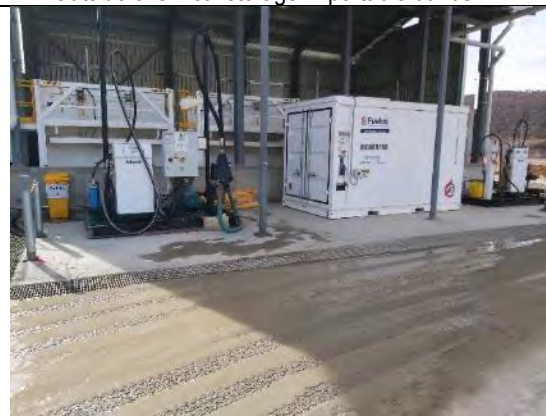
TT29: Fuel Farm. Sumps around storage and filling area
