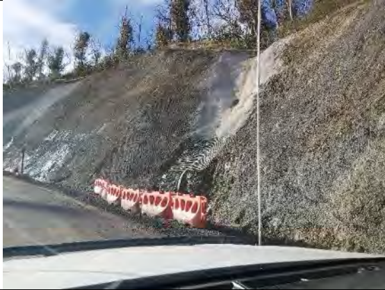
MC20: Marica Trail – “blind corner” stabilised batter
