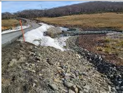
MC8: Eucumbene River crossing – gabion baskets being installed
