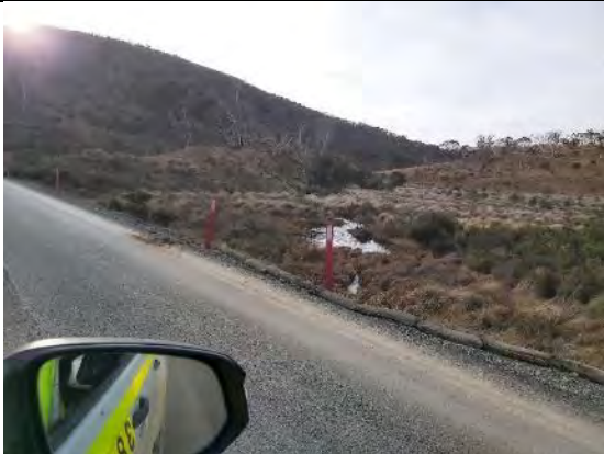
TT3 TT4: Tantangara Creek - Nungar Creek crossing – road in the vicinity has been sealed to prevent / minimise unsealed road runoff / diffuse water pollution as response to EPA regulatory actions
