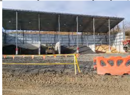
MC32: MC233: Marica Surge shaft – aggregate bins – materials used at the concrete batching plant
