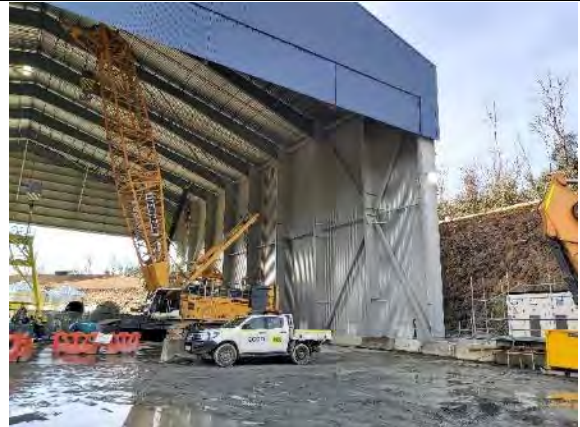
MC29: Marica Surge Shaft building
