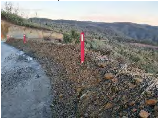
LRR 15: Roadside berms – treated with Stonewall
