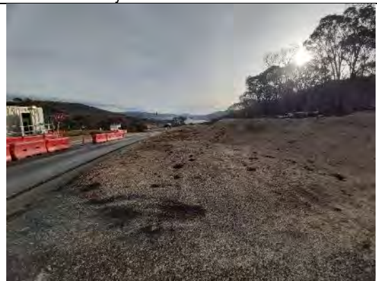
TT9: Berms and ground stabilised with hydromulch (recent damage by wild horses (widespread issue))
