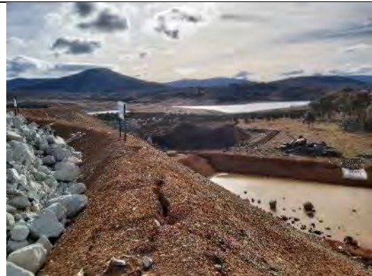
TT49: S1 spoil area – sediment basin
