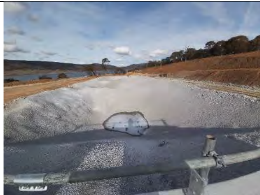
TT43: New shotcrete lined grout pits from sinkhole consolidation works under construction in spoil area – it is a waste management process to allow grout to be removed from water not suitable for the WTP to allow water to be reused on site.
