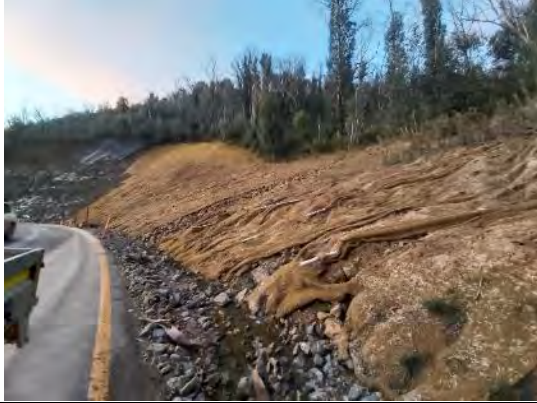
LRR 7: Further view of plastic mesh that requires replacement with a non-plastic, approved stabilisation material
