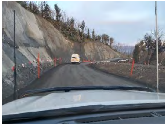
MC10: Marica trail – stabilised batters
