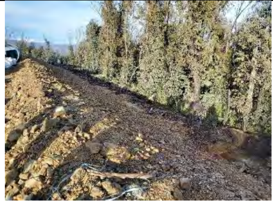
MC15: Batter at edge of the HDD pad – some washout of berm observed at base of batter – requires repair and maintenance (OBS)
