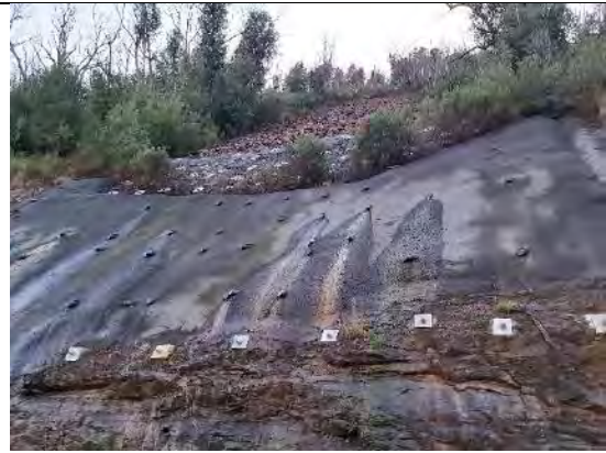
LRR 10: Stabilised / shotcreted rock face
