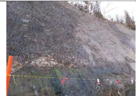
MC9: Batter stabilisation – wire mesh
