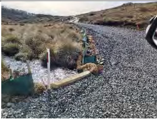
GTS9: Gooandra Creek crossing – sheeted with DGB
