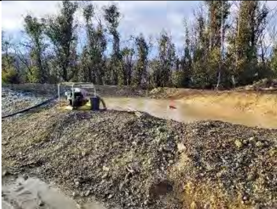
MC14: HDD Pad, pump used for dewatering (placed on "plant nappy"). Permits required for dewatering
