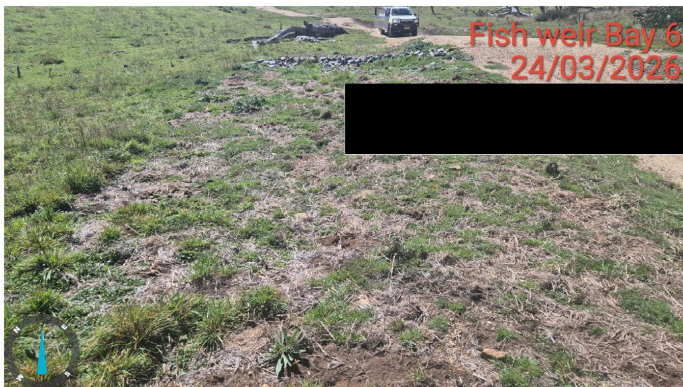
Figure 2. Fish Weir Passing Bay 6, 24 March 2026; excellent groundcover from straw mulch and direct seeding
