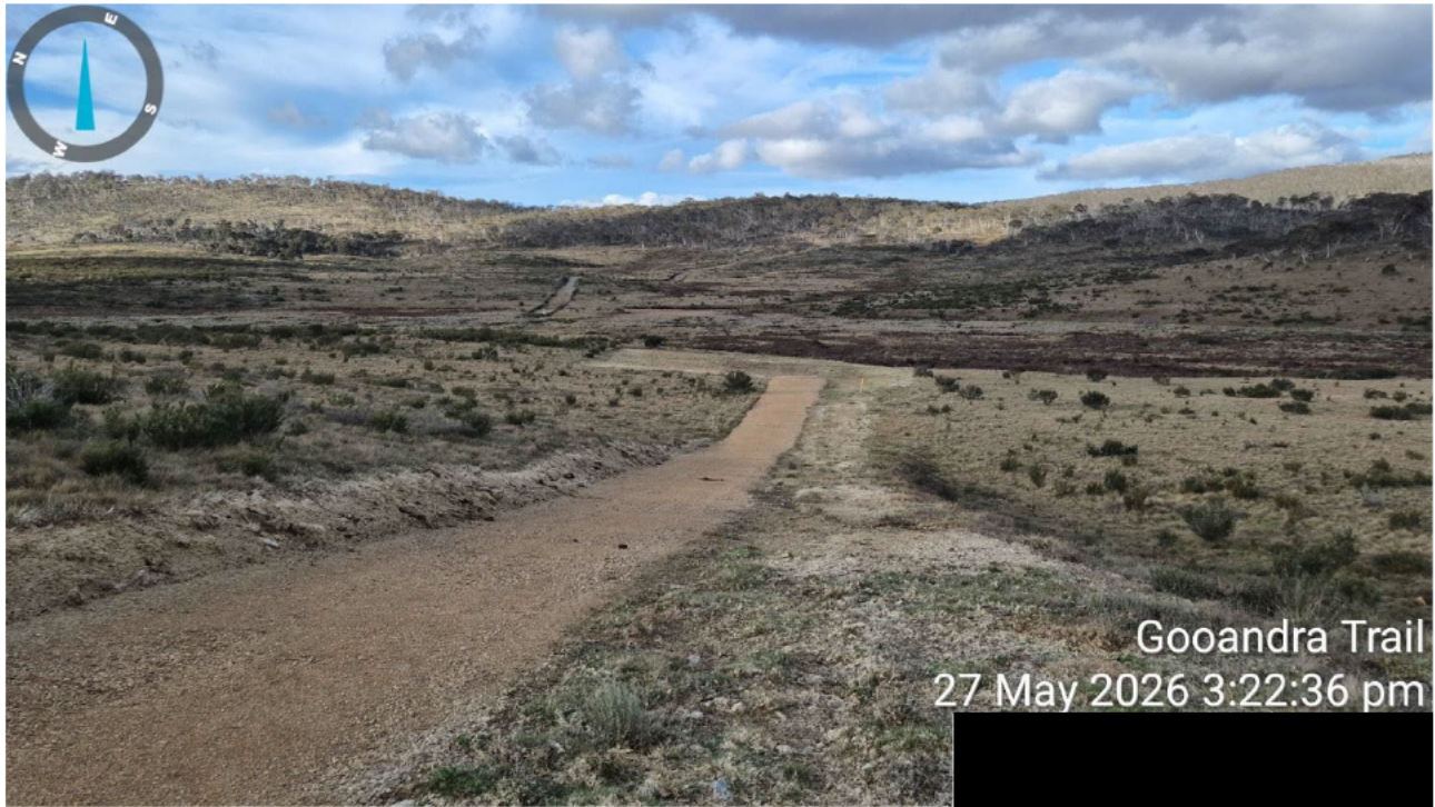
Figure 10. Gooandra Trail, 27 May 2026; hydromulching of trenchline and HDD pad complete
