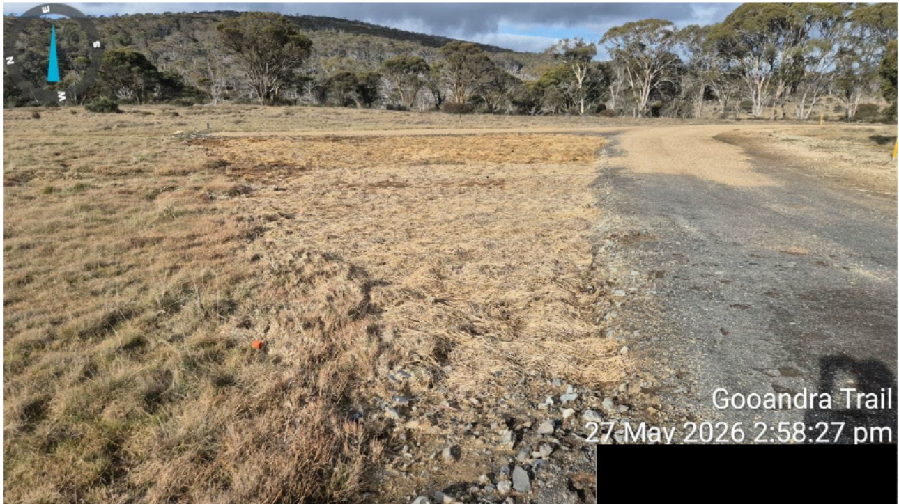
Figure 12. Gooandra Trail, 27 May 2026; former laydown pad with hydromulch and straw applied
