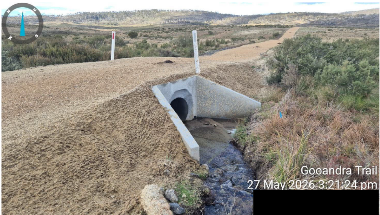
Figure 11. Gooandra Trail, 27 May 2026; all black plastic culverts have been replaced with concrete culverts, jute mesh and hydromulch applied
