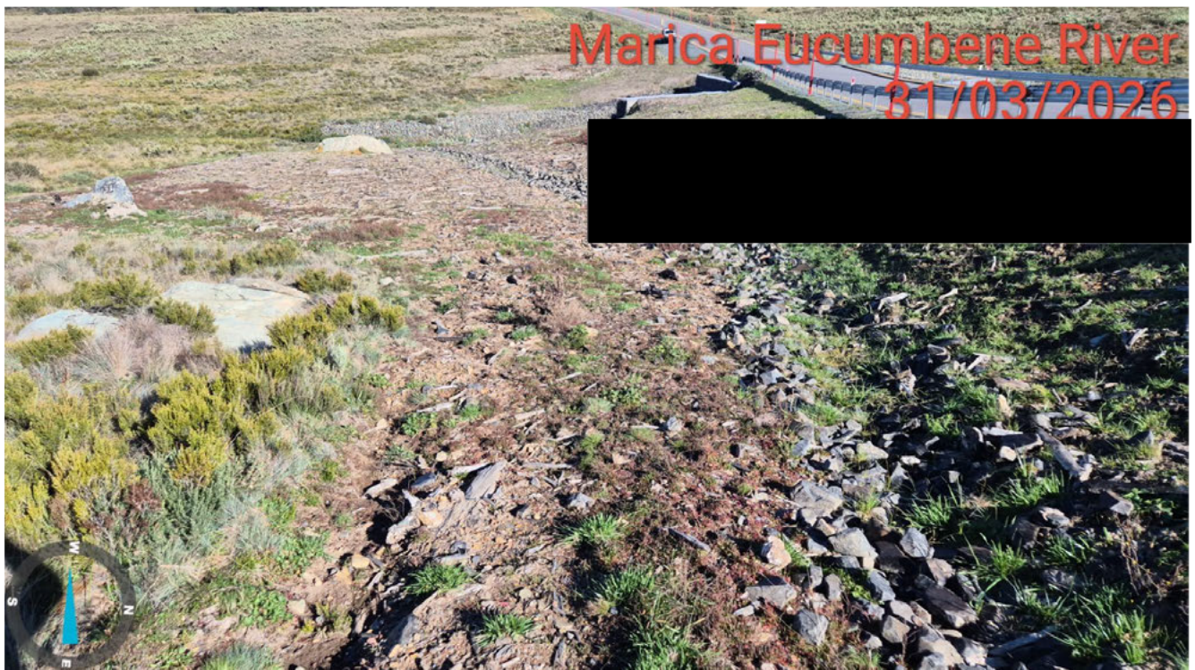
Figure 25. Marica Main Access Road, Eucumbene River Crossing, 31 March 2026; ground cover progressing
