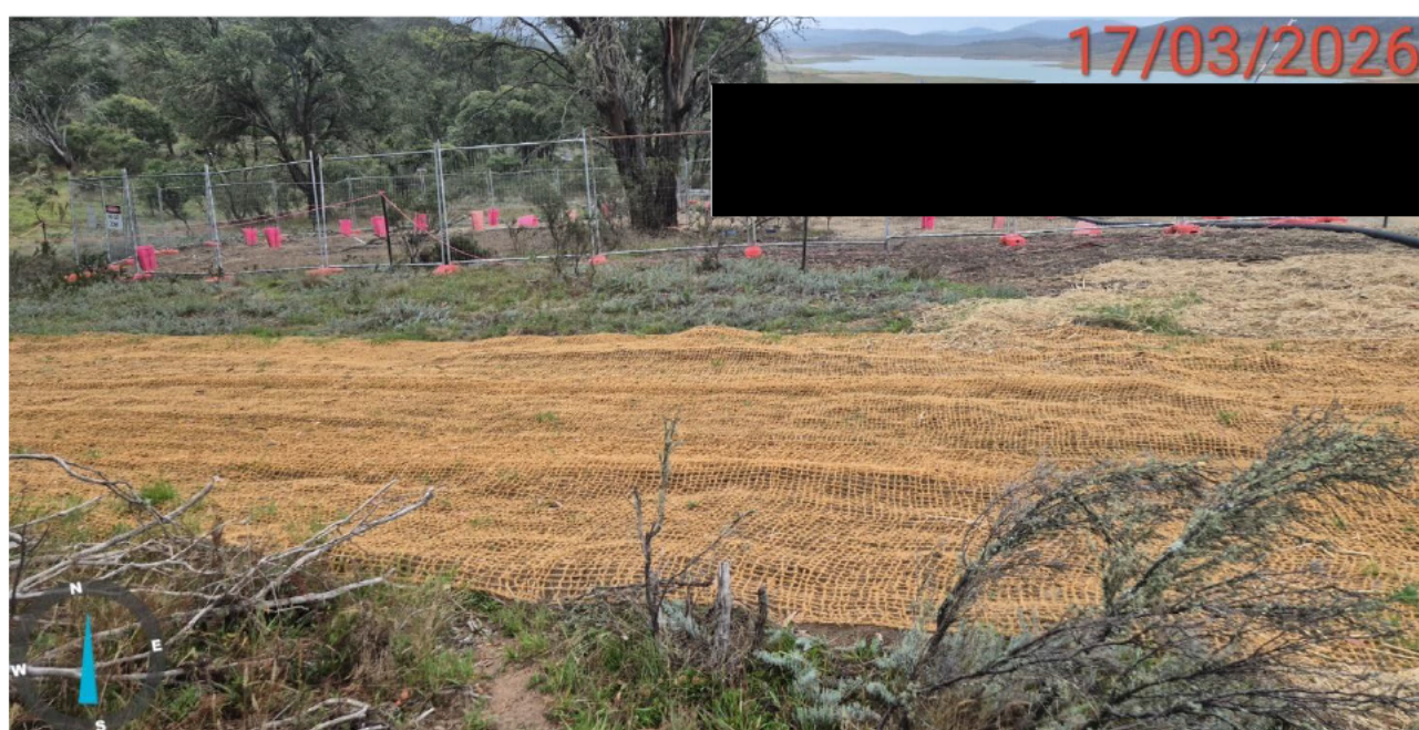
Figure 8. Rehabilitation of erosion and sediment control area of Tintangara Surface Depression 17 March 2026; survey controls removed, jute mesh and straw mulch applied, fencing in place and some tubestock planting
