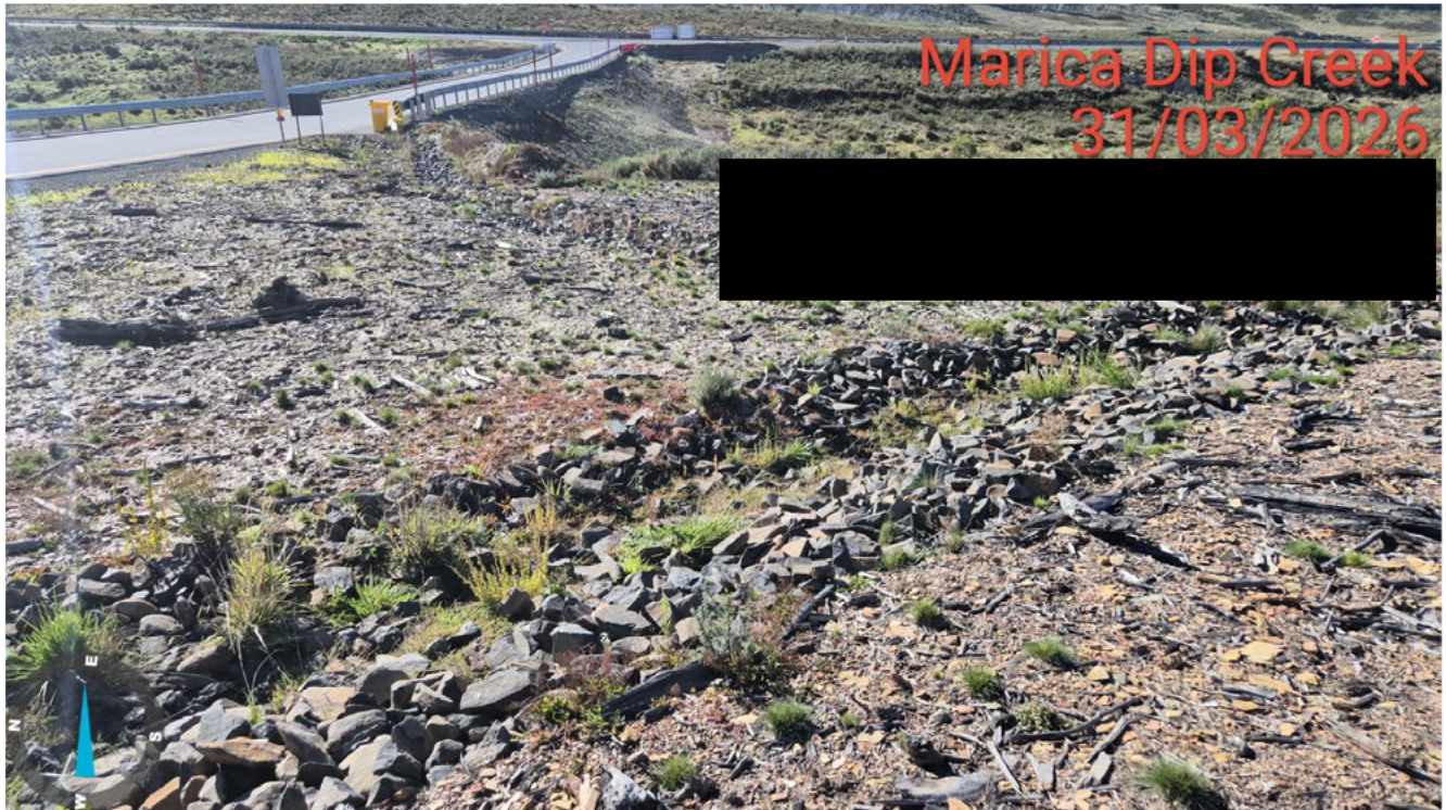
Figure 26. Marica Main Access Road, Dip Creek Crossing, 31 March 2026; ground cover progressing.
