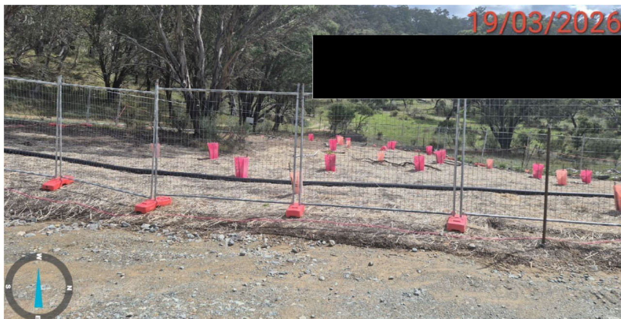
Figure 7. Tintangara Surface Depression, 19 March 2026; fencing in place, straw mulch and thatch applied and some tubestock planting
