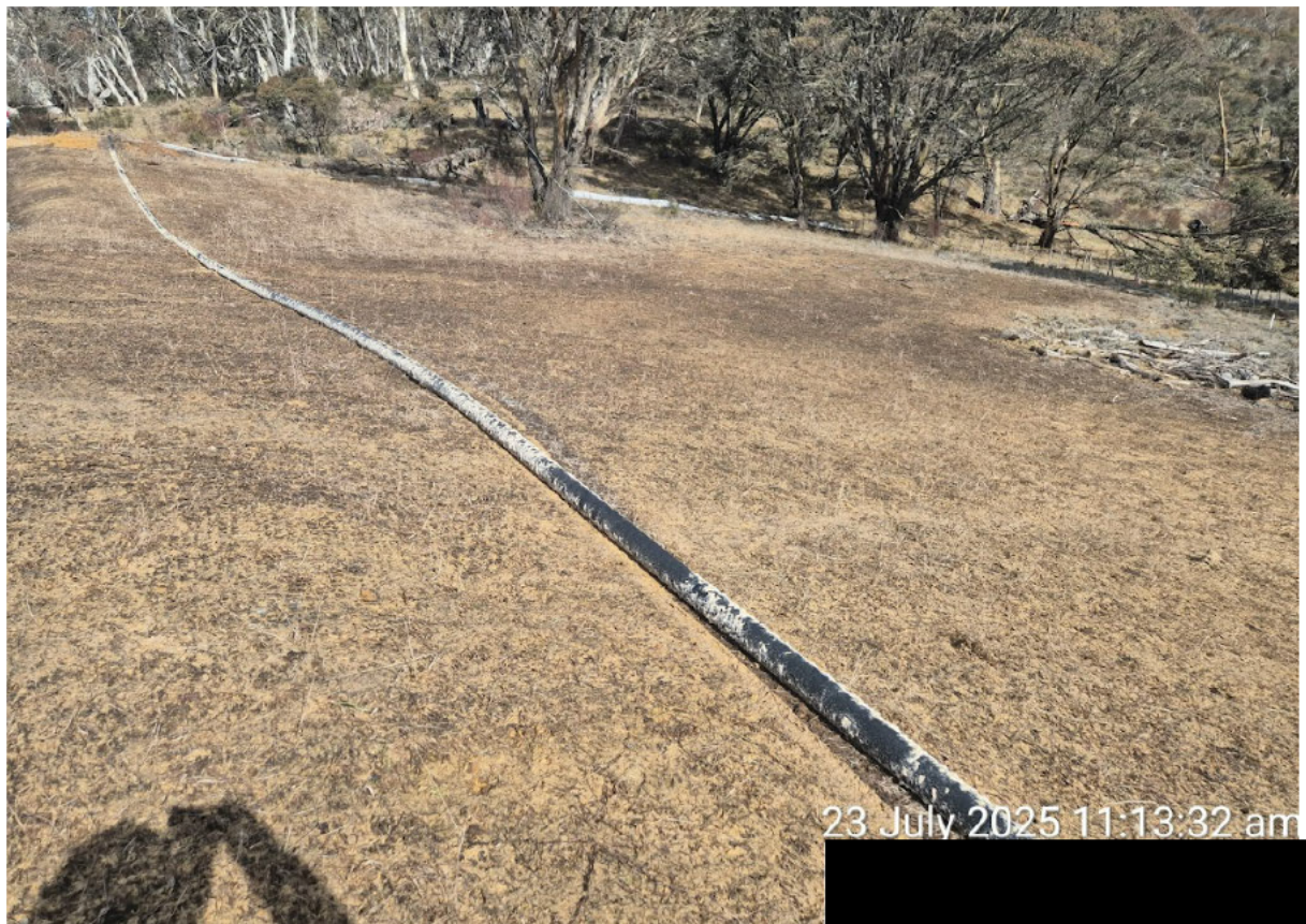
Figure 5: Tantangara Surface Depression following hydromulch application Date- 230725
