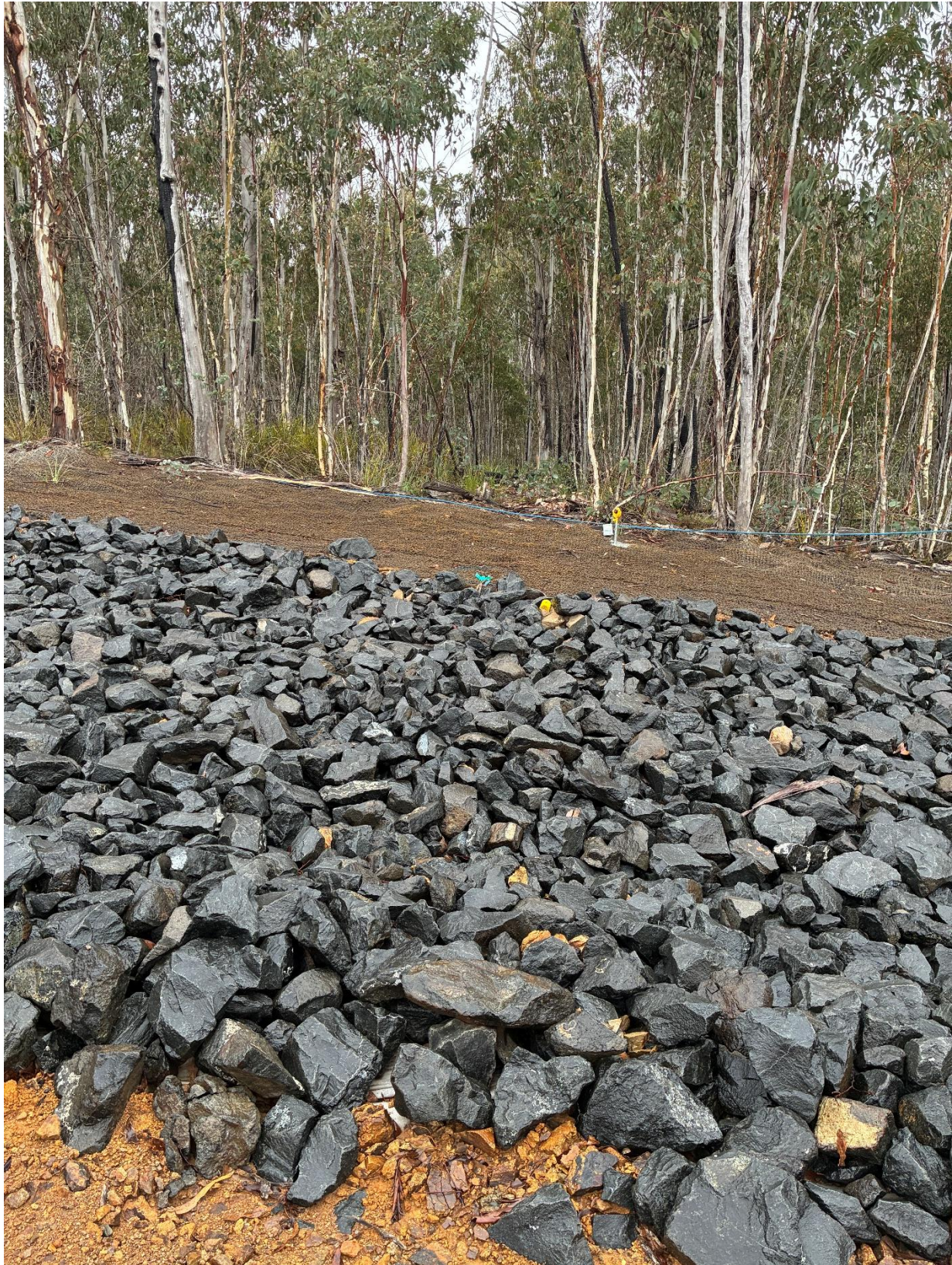
Photograph 3 – Foot track along line of tiltmeters over tunnel centreline. Note tiltmeter at CH10m near tree line.
