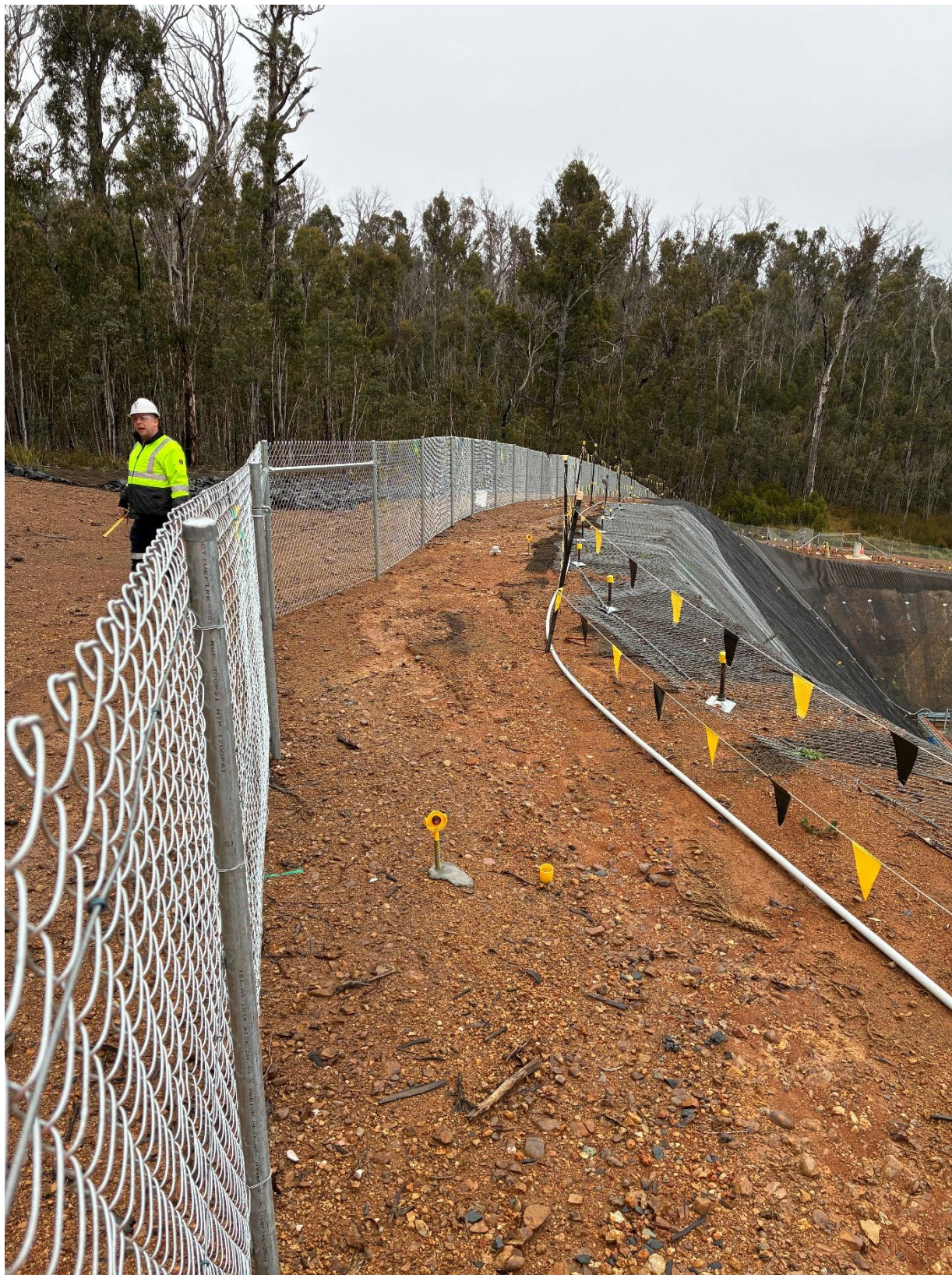
Photograph 1 – General view of the crest of the Portal Cut showing prisims located at crest of cutting
