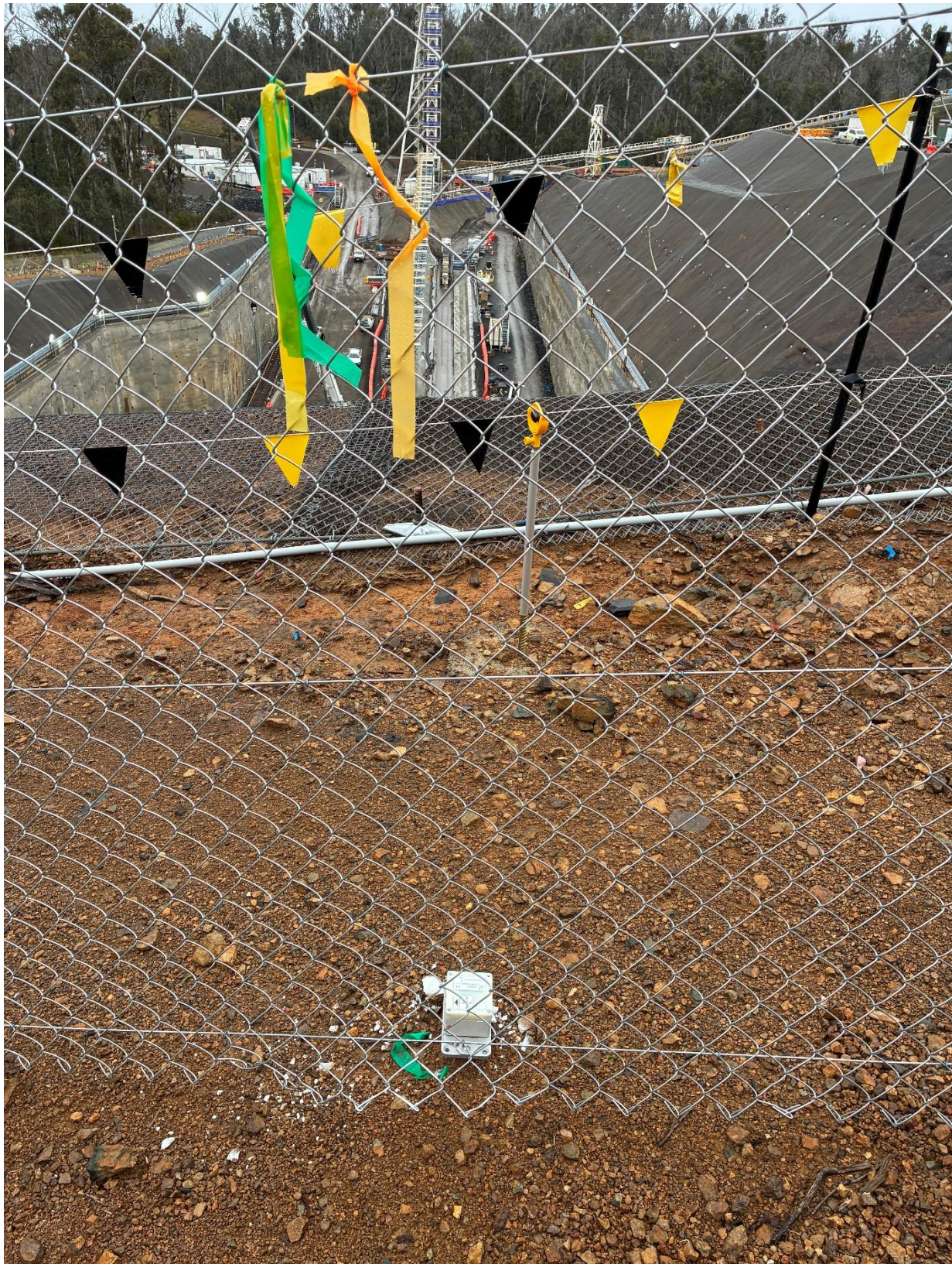
Photograph 2 - Prism and tiltmeter located on centreline of tunnel at the crest of the portal
