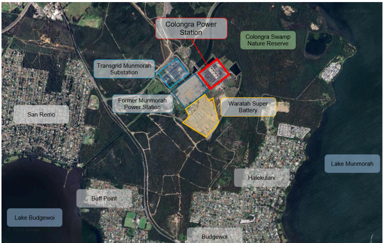
Figure 2.1: Colongra Power Station Location Aerial View
