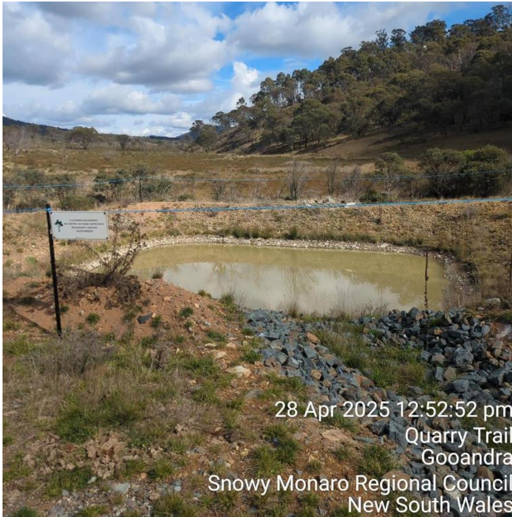
Figure 6.10: Exclusion zone established around sediment basin CH805.
