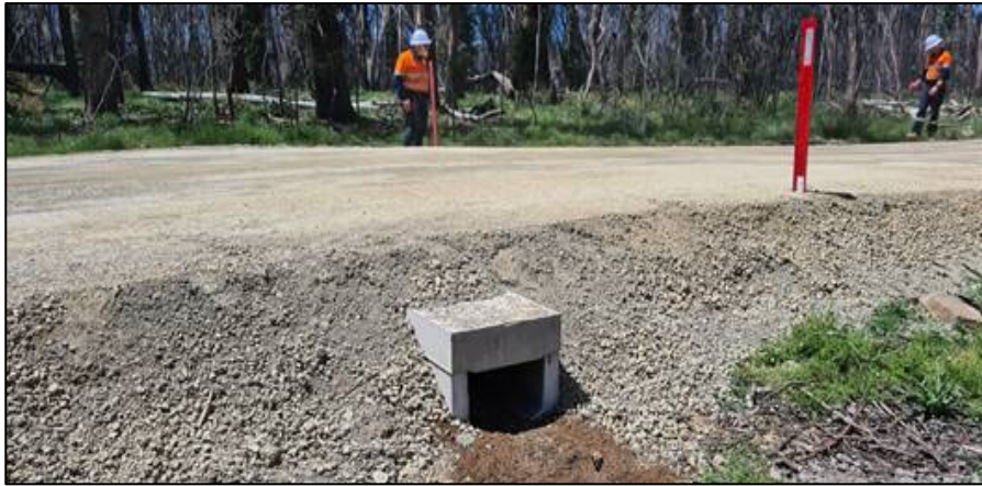
Photograph 5 - showing smaller culvert and 'ramp' over
