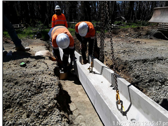
Photograph 3 - Installation of trial underpass
