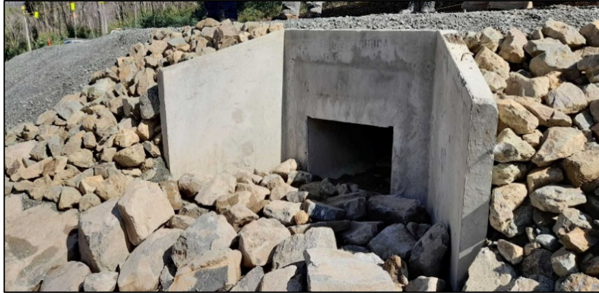
Photograph 9: Installed headwall and rip rap
