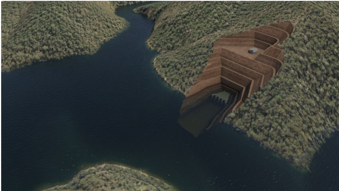
Figure 4: Surface View of Talbingo intake and intake gate structure, an example of how the BIM system could look at the end of the Project
