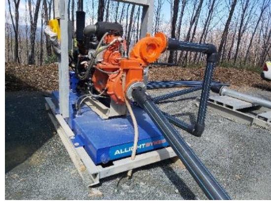
MC24: Pump installed at water tank. It requires bunding to contain any spills / leaks.
