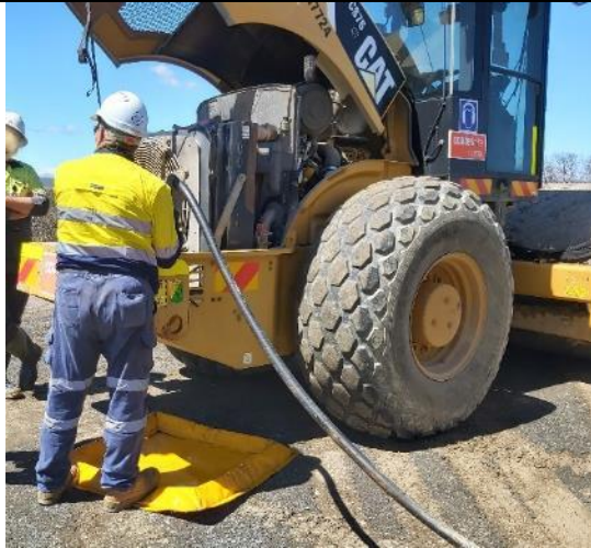
MC28 and MC29: Refuelling of plant in progress. Portable bund / plant nappy used to contain potential spills. Spill materials were on hand nearby in refuelling truck
