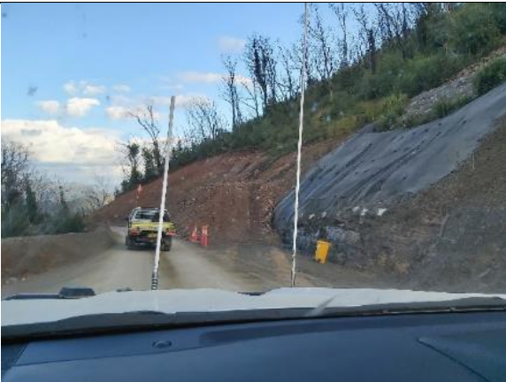
LHRR11: Stabilisation of batter and ongoing road widening activities along Lobs Hole Ravine Road
