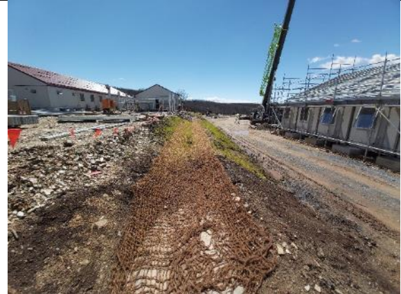
MC27: Marica Camp – under construction – seeding / revegetation of batters appears to be successful to date
