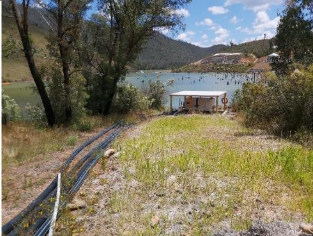
LH29: Old / backup water intake pump area – now has permanent bunding. Audit#1 identified inadequate bunding – now fixed. Intake was operating on the day of the audit
