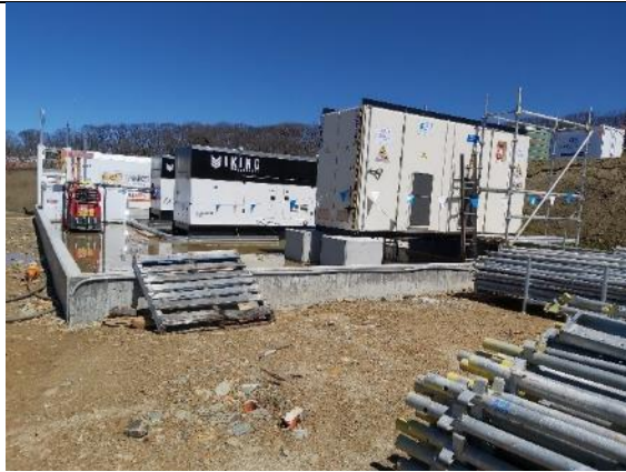
MC30: Bunded pad for generators and fuel storage – Marica Camp
