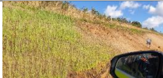
TT26: Stabilisation of batter, hydromulched
