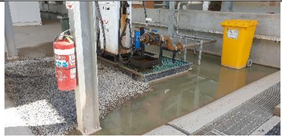
LH1 and LH2: Fuel Farm. Noted ingress of water – roofing is not sufficient to prevent ingress of water during heavy rain
