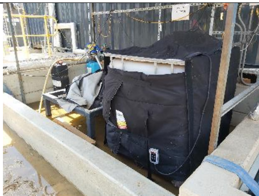
LH13, and LH24: Sodium Hydroxide stored in a bund with acids (incompatible) at the STP. This was identified as an issue at the previous audit (see NC)
