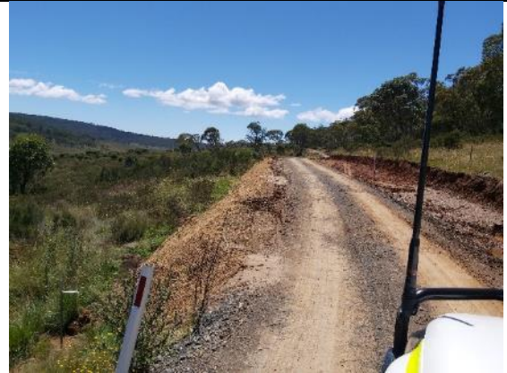
TS10: Jute mesh stabilising batter, recent clearing works on RHS of Gooandra Trail
