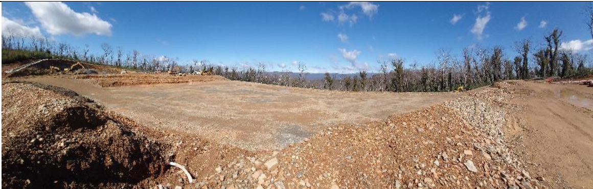
MC22: View of Marica Surge Shaft pad under construction. The area will first be filled, then the surge shaft will be excavated through to the tunnel.
