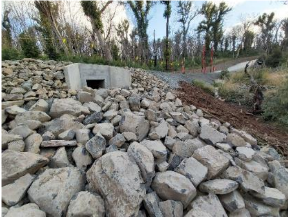
LHRR7 : Recently completed wildlife underpass (low side) (one of 6 being constructed)
