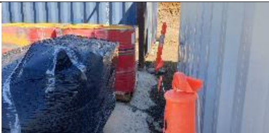
TT23: Chemical storage at receiving area, not bunded
