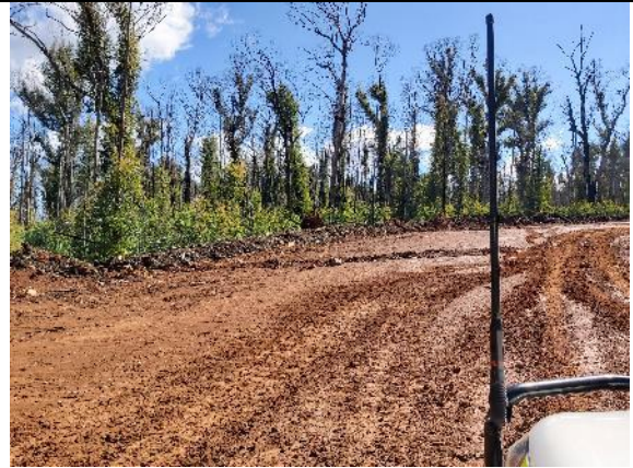
MC20: HDD track – cross drain diverting water off the roadway to small sediment basins
