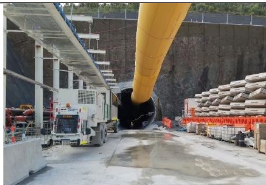
LH8: MAT Portal – length was approximately 1km at the time of the audit. Segments for installation in the tunnel
