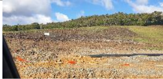
TT20: Clean top soil stockpile, clearly marked (signposted), hydromulched
