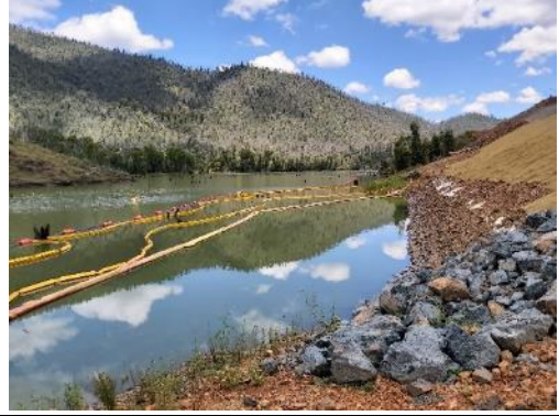
LH28: Silt curtains in place near the Talbingo intake area
