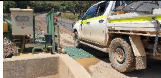
TT40: Tintangara wash down station; not operational at the time of the site inspection due to water pump malfunction and had they also run out of water.
