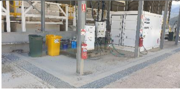
LH1 and LH2: Fuel Farm. Noted ingress of water – roofing is not sufficient to prevent ingress of water during heavy rain
