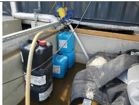
LH13, and LH24: Sodium Hydroxide stored in a bund with acids (incompatible) at the STP. This was identified as an issue at the previous audit (see NC)
