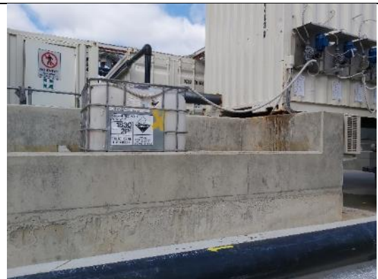
LH6: IBC of sulphuric acid within bund at water treatment plant
