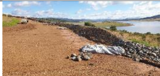
TT28: Spoil Road to Peninsula Emplacement Area, sediment controls, dam side
