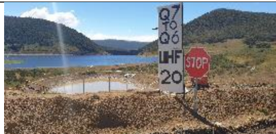
TT24: One of various sediment basins near Tantangara Reservoir (each were numbered)
