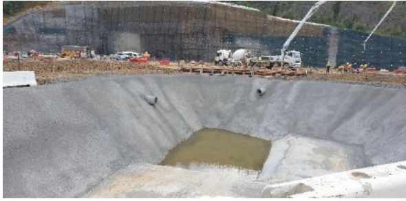
LH27: Talbingo Adit area – laying foundations and basin
