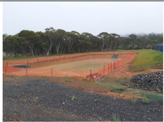
RF9: Sediment basin on the Rock Forest site. It was noted that there had been heavy rain events over the days prior to the site visit.
