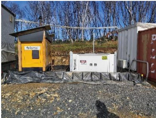
MC9: Marica Office Pad with generator set up in a bunded area
