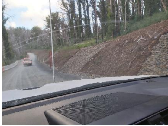
LHRR9: Stabilised batters
