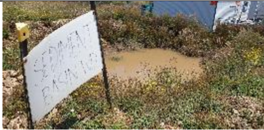
TT39: Sediment basin, water used for wash down station
