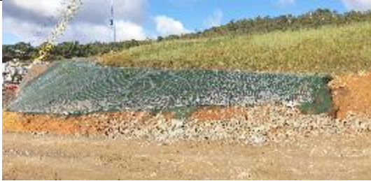
TT19: Stabilisation of batter
