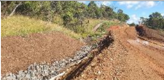
TT25: 3 Spoil Road to Peninsula Emplacement Area, clean water diversion, sediment controls in place
