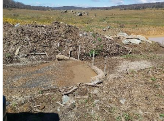
MC8: Basin and sediment controls near Marica Trunk services work – coir log working but requires maintenance.
