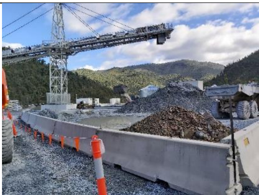
LH7: Tunnel spoil – excavated from Main Access Tunnel (MAT) Portal tunnel -
