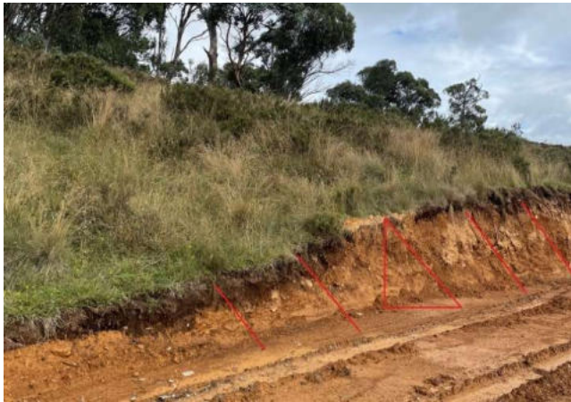
Figure 3: Proposed Batter reinstatement (as indicated by red)
