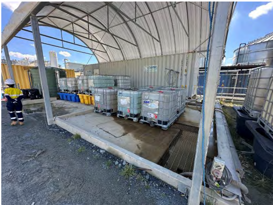
Photo 12 – Bulk hydrocarbon storage at Tantangara meting AS 1940.
