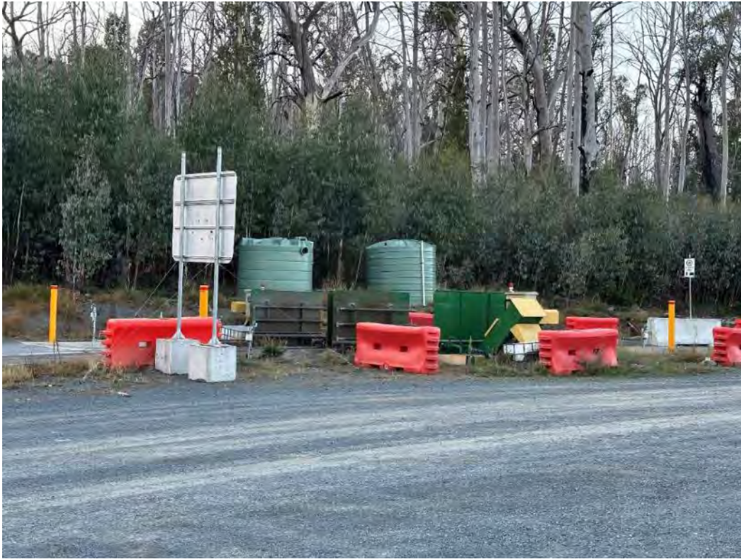
Photo 23 – Wheel wash station at Lobs Hole Gate House.
