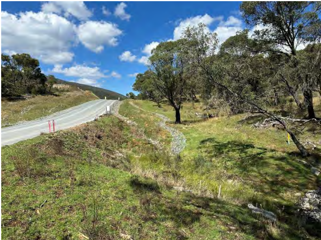
Photo 08 – Quarry Road diversion drains are stable with well vegetated areas.
