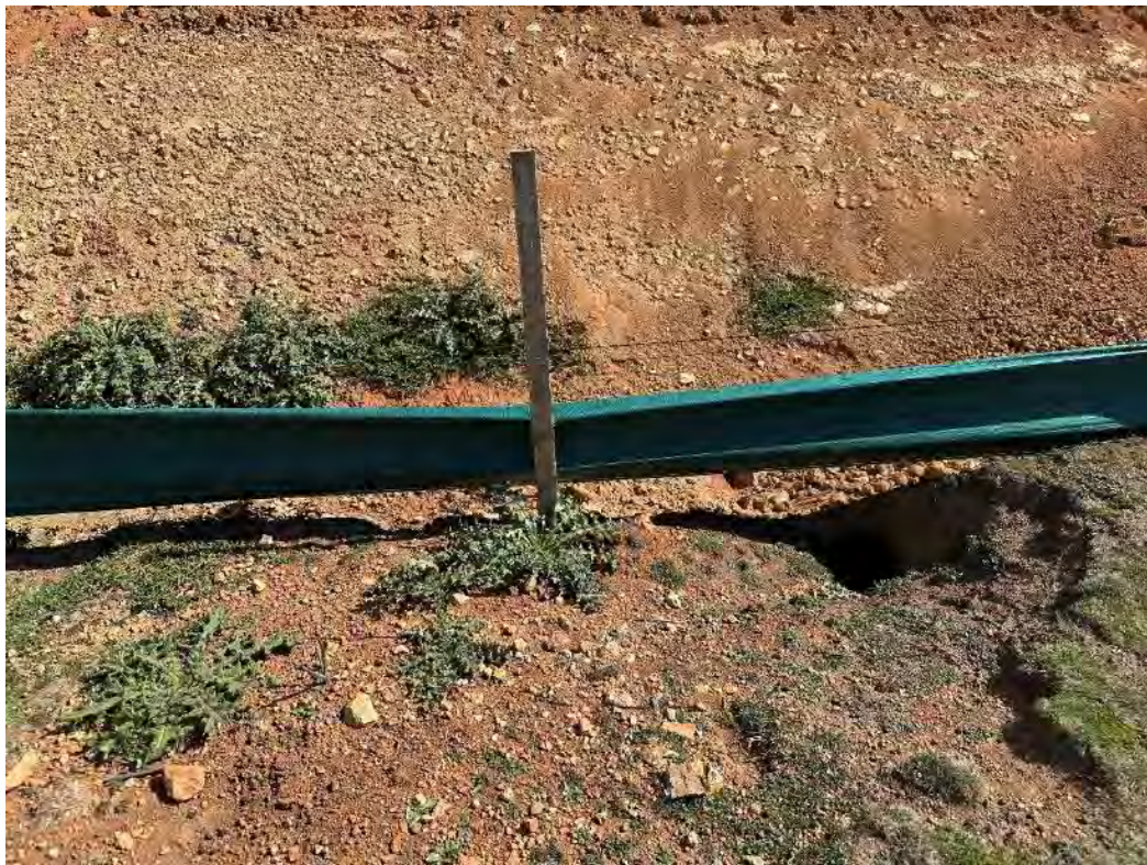
Photo 22 – Ineffective sediment fence and rabbit damage to permanent spoil laydown low point/project boundary. See IMP REC 17.
