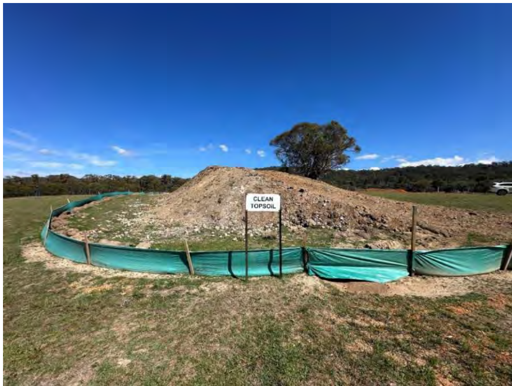
Photo 61 – Topsoil stockpile and effective sediment fencing (Rock Forest).
