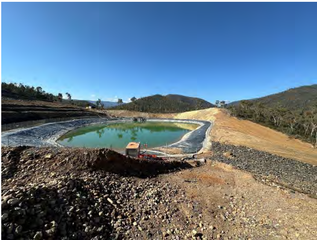
Photo 24 – Leachate basin (SB01) below the permanent spoil emplacement (Ravine Bay).
