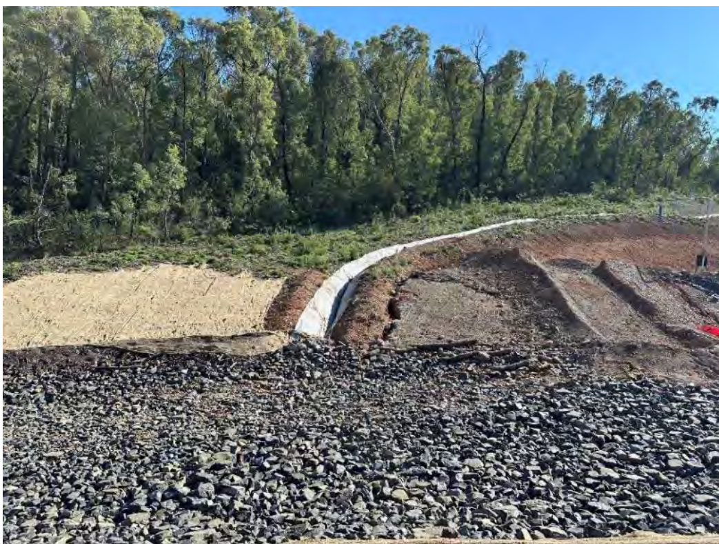
Photo 27 – Minor erosion along drain at Permanent Spoil Emplacement (Ravine Bay). See IMP REC 25.
