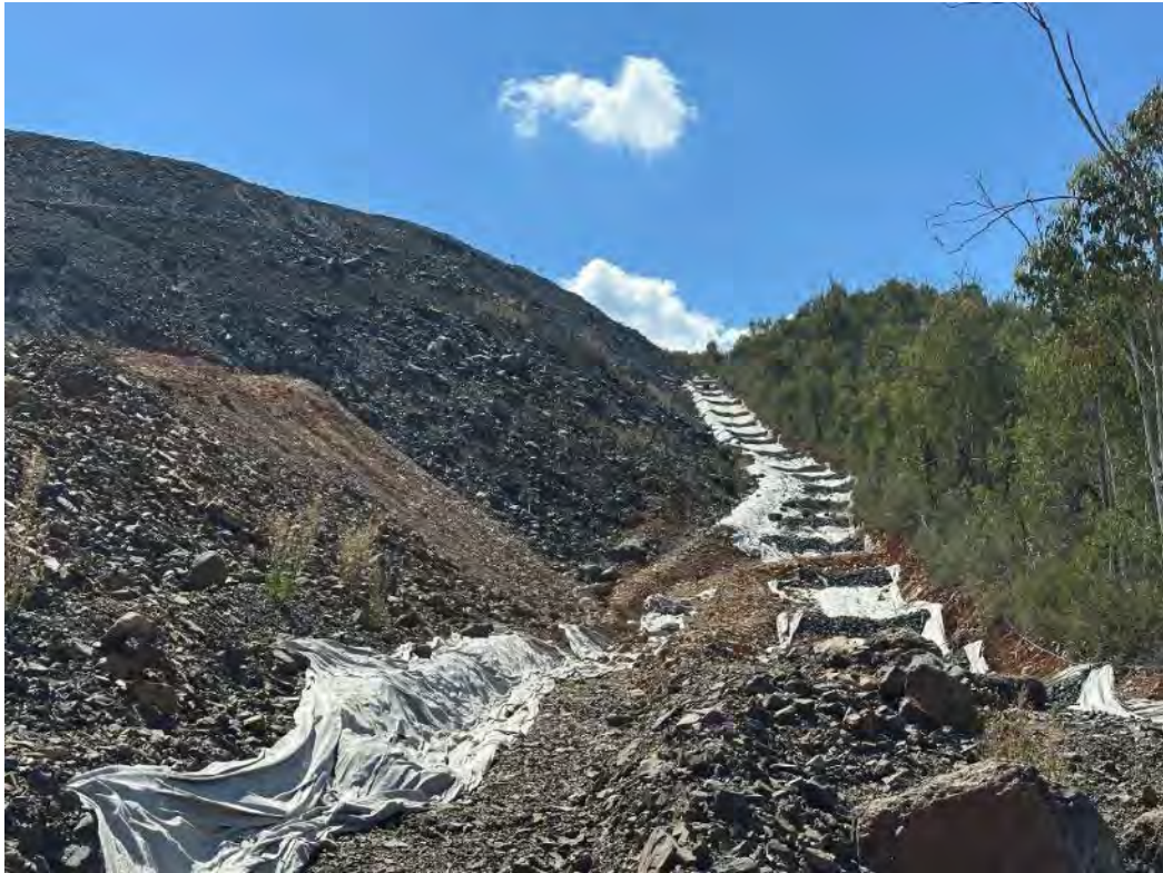
Photo 33 – GF01 clean/dirty diversion drain.
