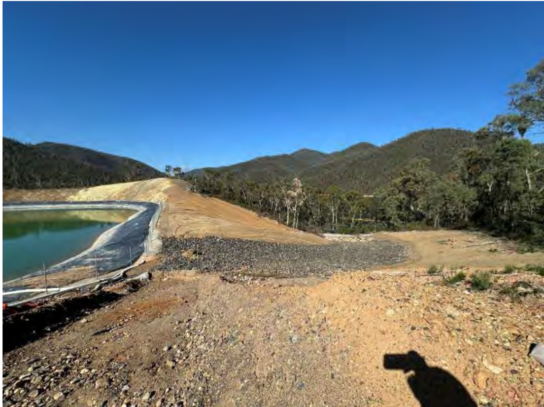
Photo 25 - Leachate basin (SB01) spill way.
