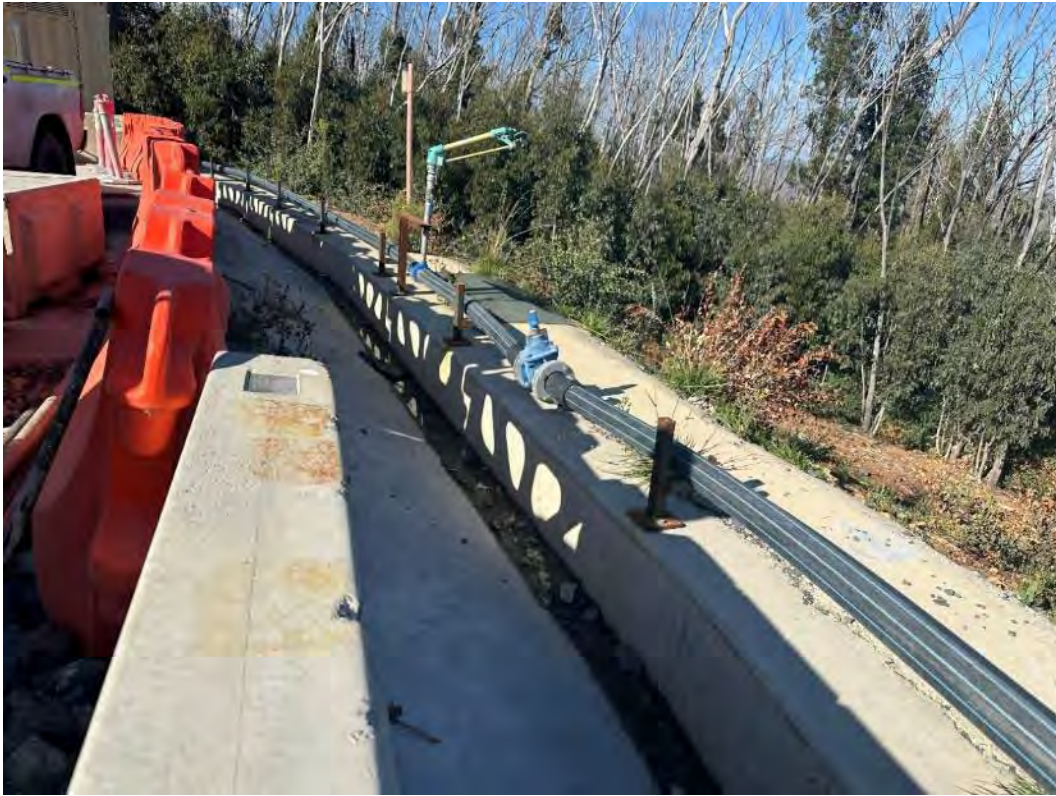
Photo 51 – Boundary drain around the Marica Surge Shaft with sprinkler system fitted.
