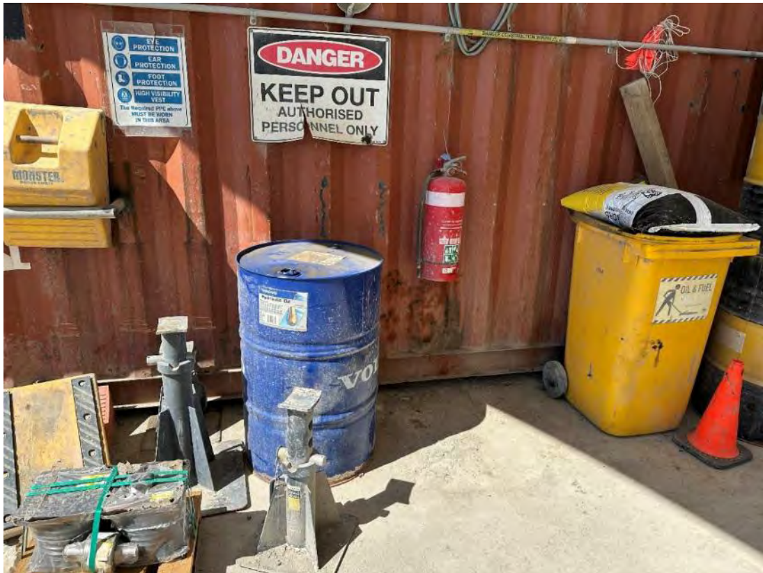
Photo 41 – Contractor yard (Main Yard) hydrocarbons incorrectly stored. See NC REC 14.
