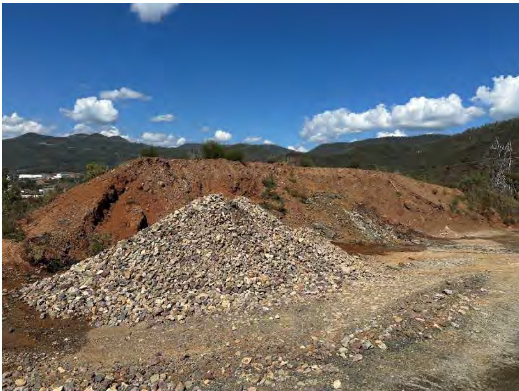
Photo 34 – Topsoil stockpile at GF01 Leachate basin. Topsoil mixed with non-topsoil material, weeds present and no signage. See NC REC 4.
