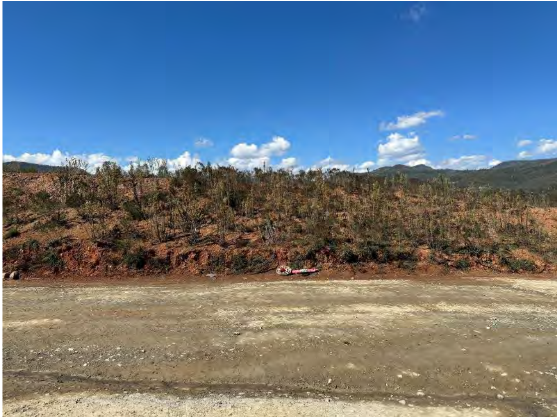
Photo 35 – Topsoil stockpile dominated by weeds at GF01. See NC REC 4.
