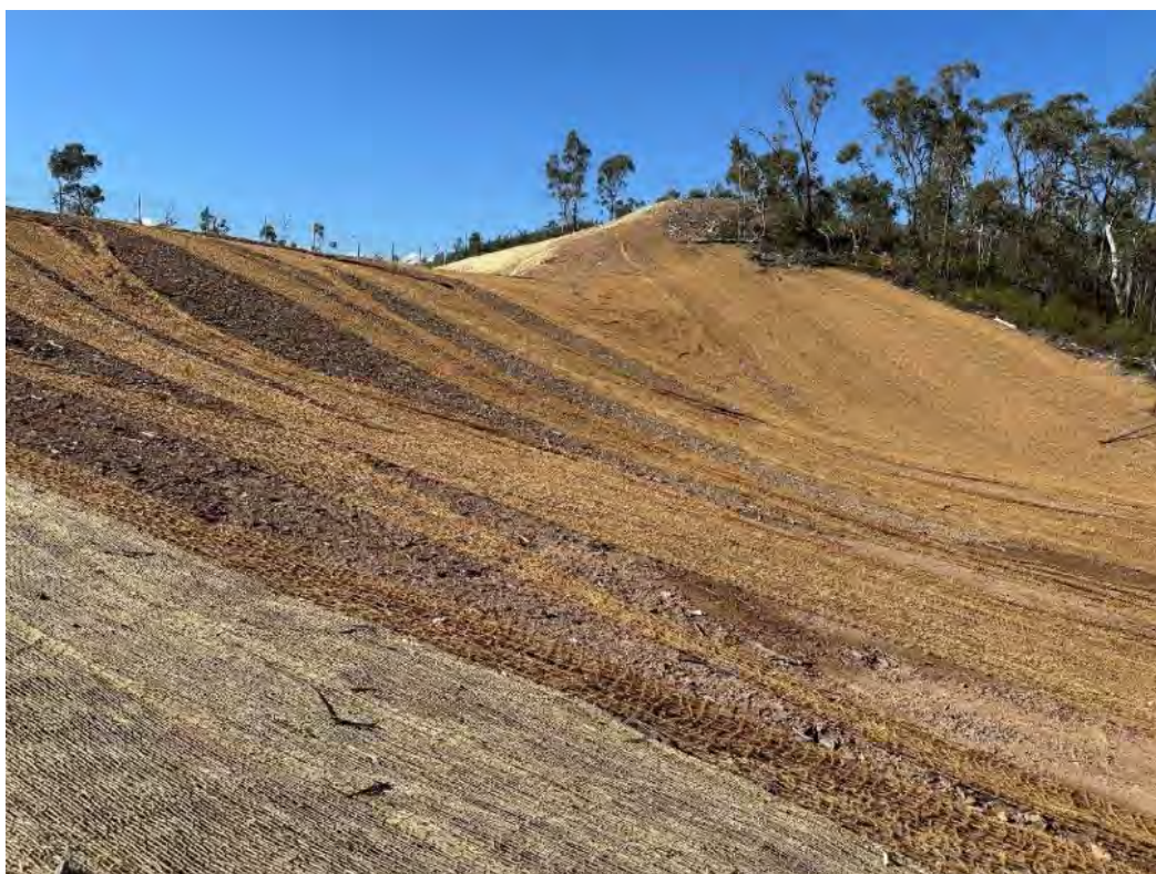
Photo 28 – Jute mesh used on batter between leachate basin (SB01) and Talbingo Reservoir. See IMP REC 13 about completion of the works.
