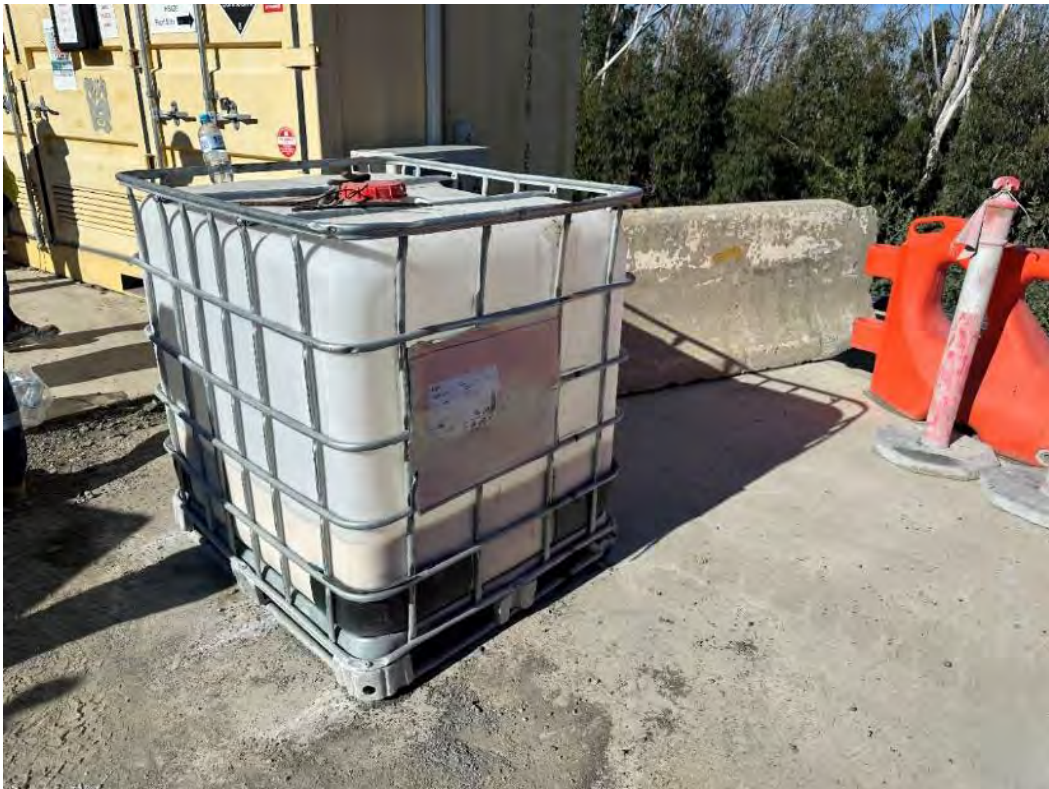
Photo 52 – Hydrocarbons incorrectly stored at Marica Surge Shaft.
