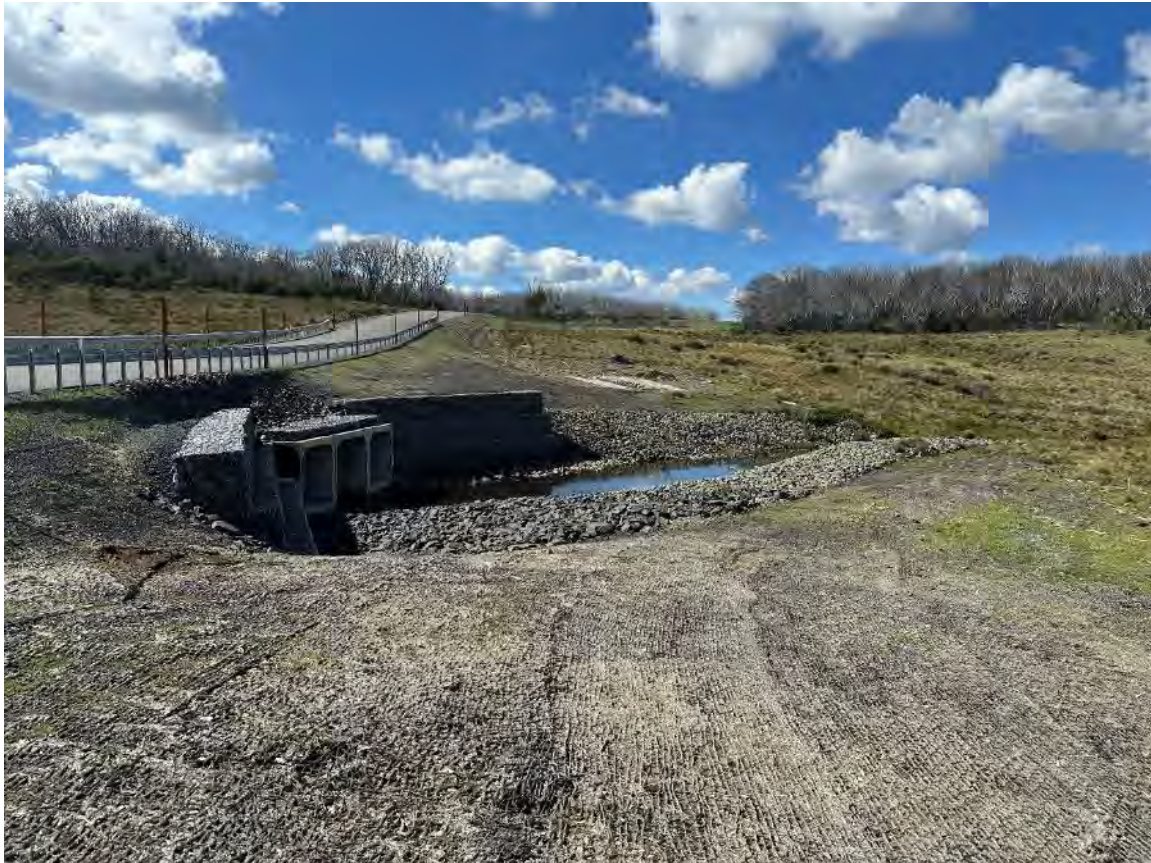
Photo 59 – Culvert along Marica Trail with jute mesh used for ground stabilisation.
