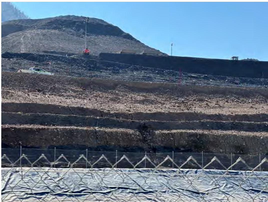
Photo 26 – Erosion on batter between Permanent Spoil Emplacement (Ravine Bay) and Leachate basin (SB01). See IMP REC 25.
