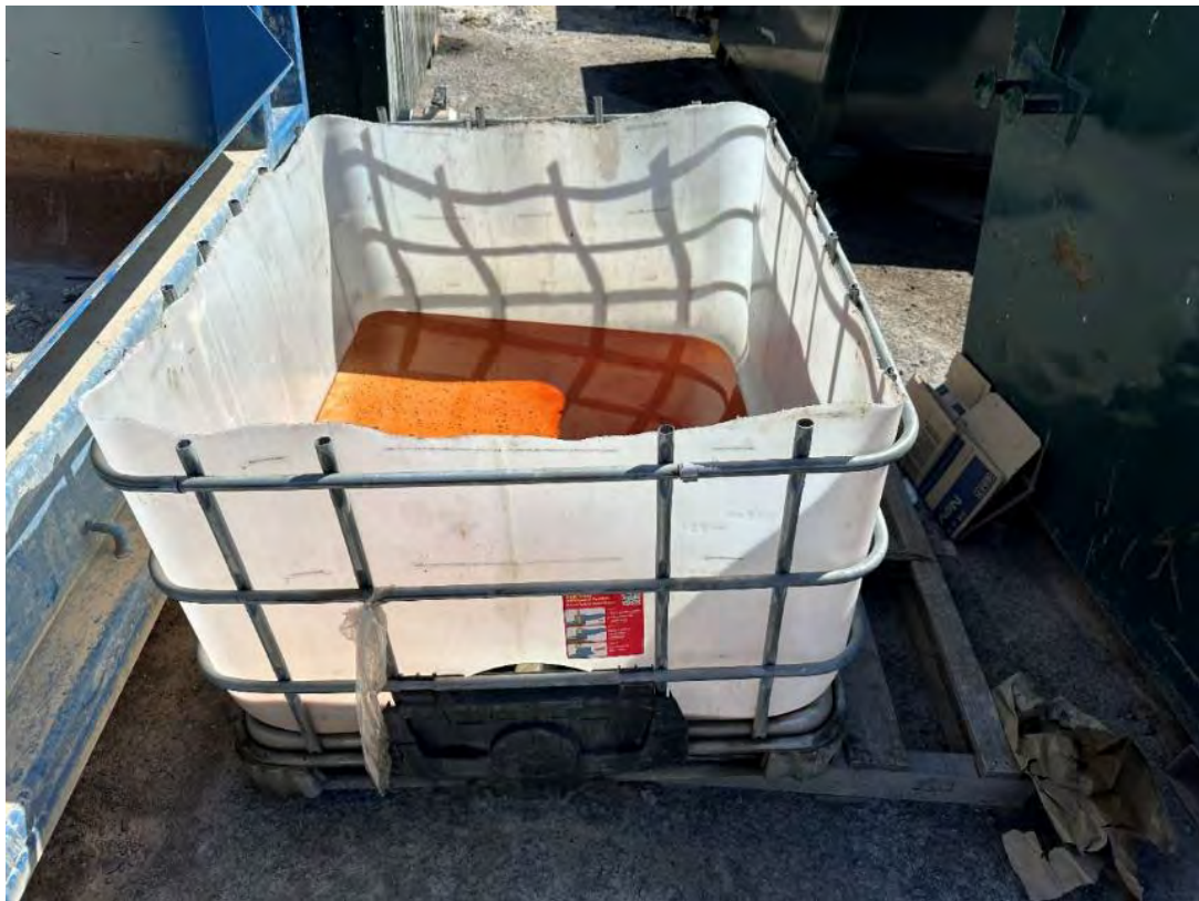
Photo 46 – Contractor yard (Main Yard) waste hydrocarbons incorrectly stored. See NC REC 14.
