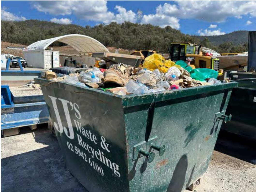
Photo 43 – General waste bin in contractor yard (Main Yard). Note no bin lid covering with loose waste material. See NC REC 15.
