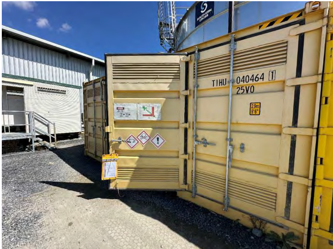
Photo 09 – Hydrocarbon storage at Dewatering/Reverse Osmosis area. Meeting AS 1940.
