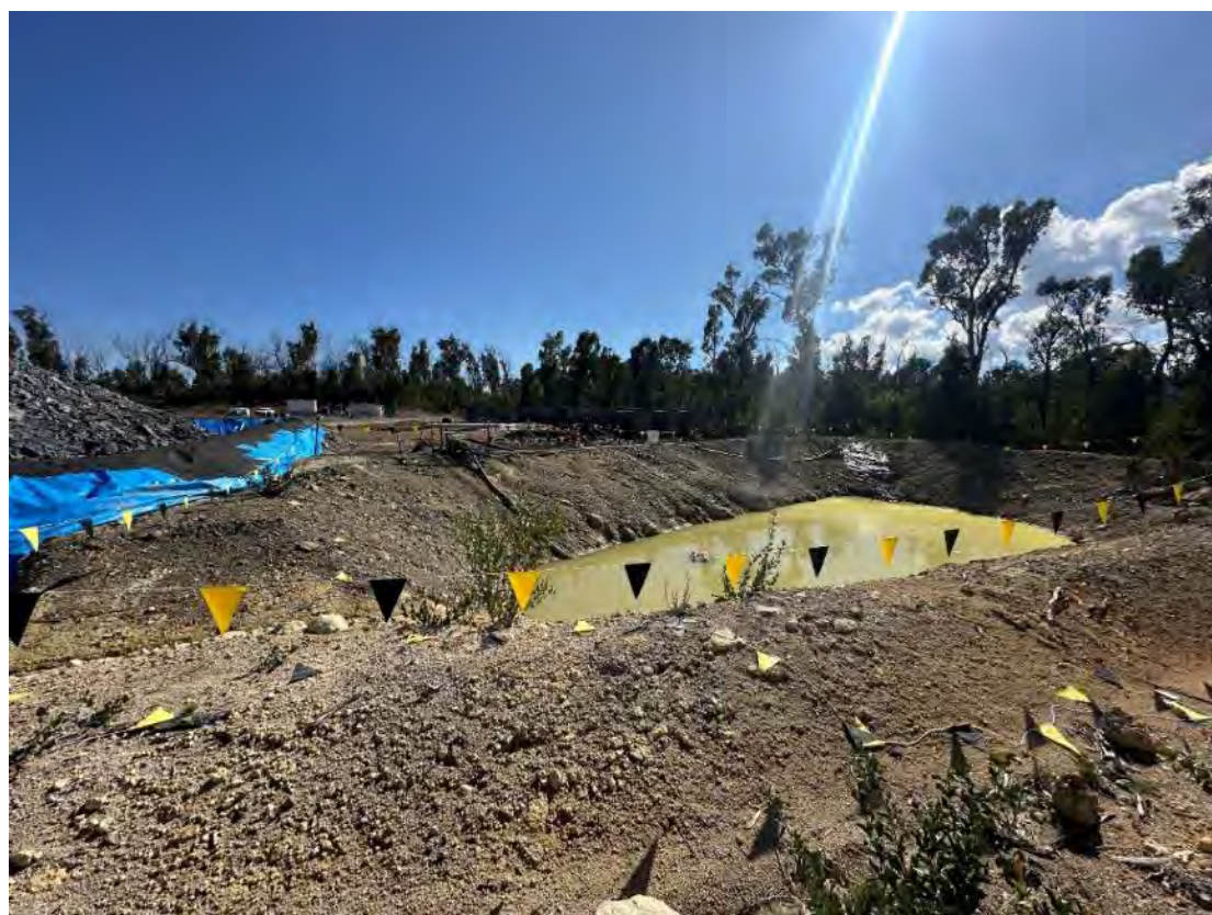
Photo 56 – Leachate basin at Marica West HDD Pad.
