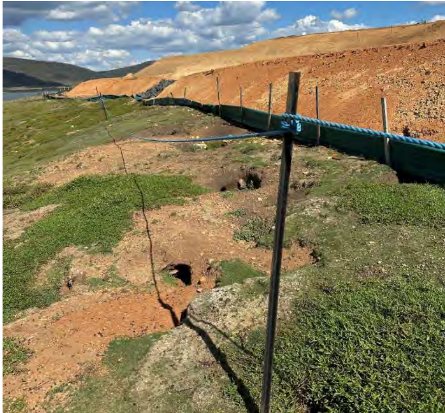
Photo 21 – Rabbit damage at permanent spoil laydown low point/project boundary. See IMP REC 17.
