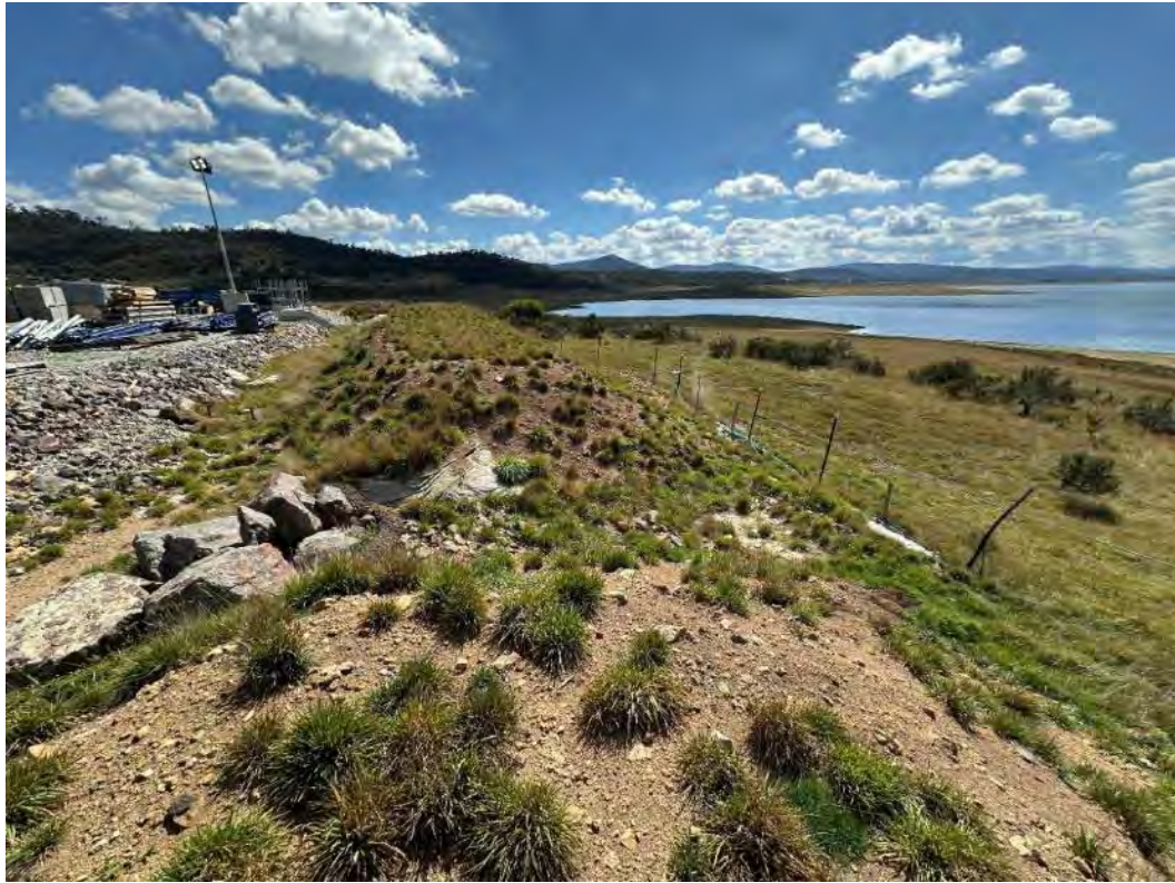
Photo 13 – Storage yard diversion drain flowing into sump. Sump was at capacity with sediment. Sediment fence behind sump is damaged.
