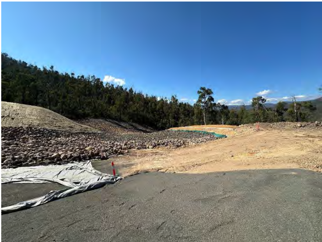
Photo 30 – Construction of Permanent Spoil Emplacement (Ravine Bay) diversion drain.
