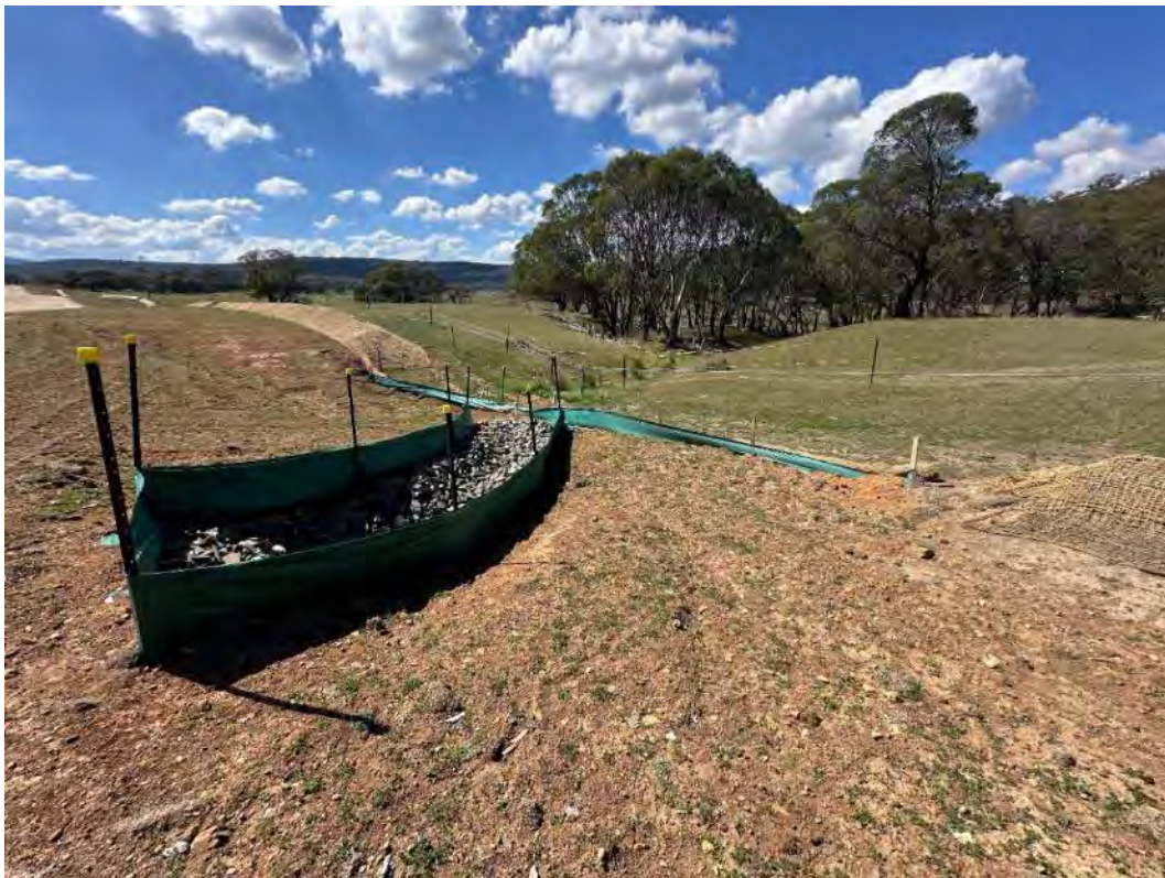
Photo 63 – Sediment controls along roadside at Rock Forest. See IMP REC 24 about considering other controls.
