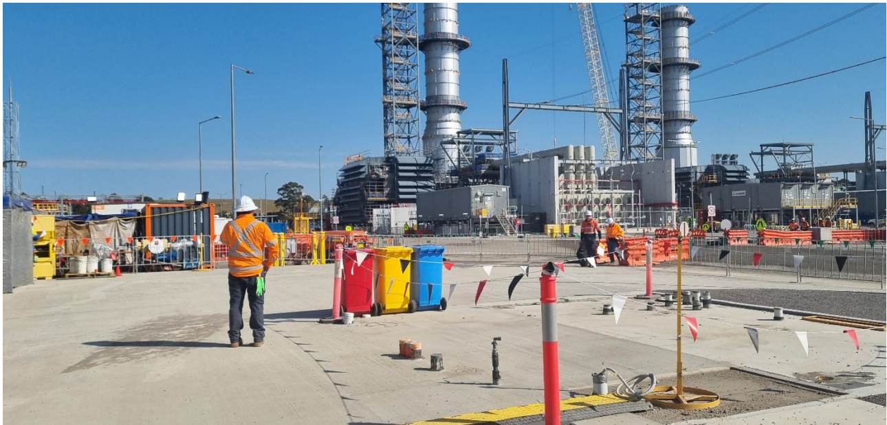
Photograph 1: Gas Turbine exhaust stacks under construction
