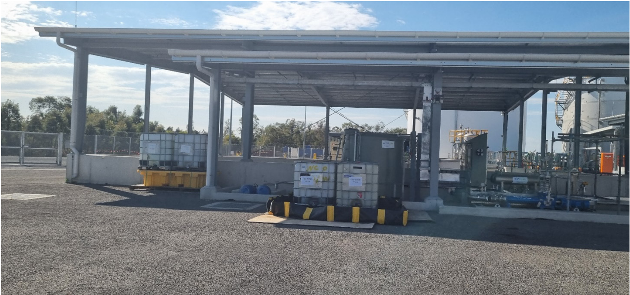
Photograph 3: Water Treatment Chemical Storage
