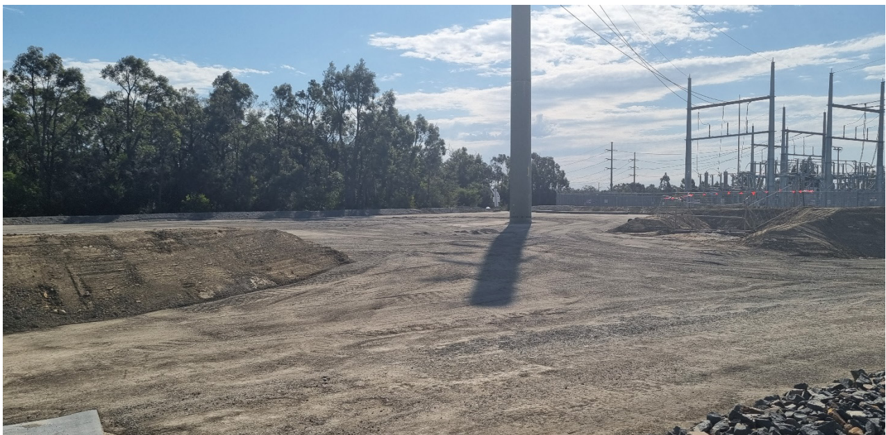
Photograph 8: Location of former construction sediment basin
