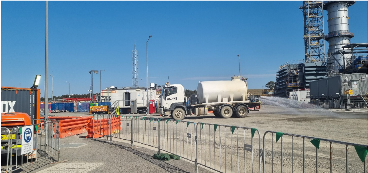
Photograph 5: Water Cart in operation
