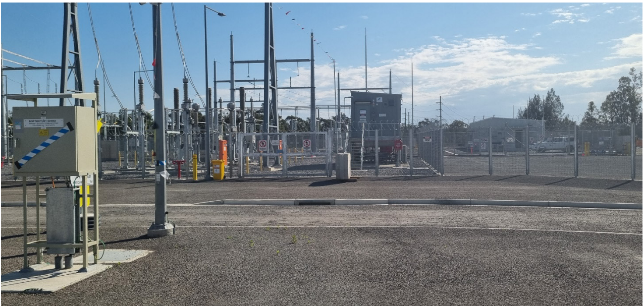
Photograph 4: Sealed hardsstand and power island
