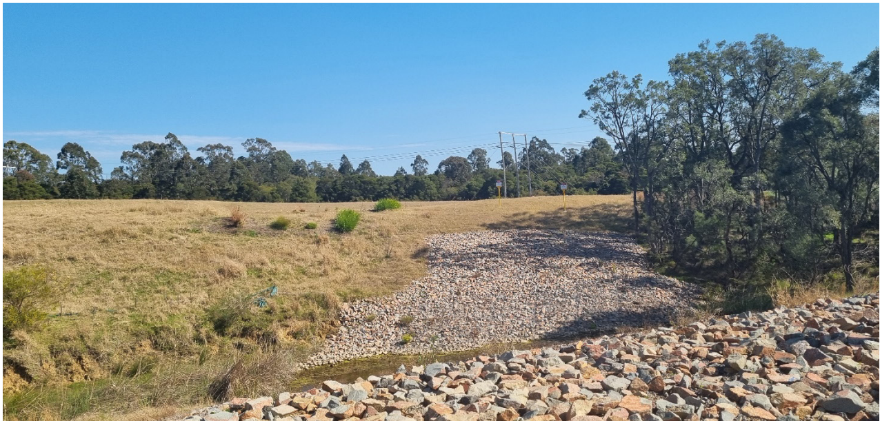
Photograph 6: Connecting gas pipeline rehabilitation and scour protection
