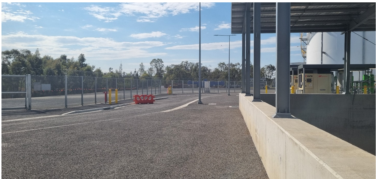
Photograph 2: Sealed internal roads
