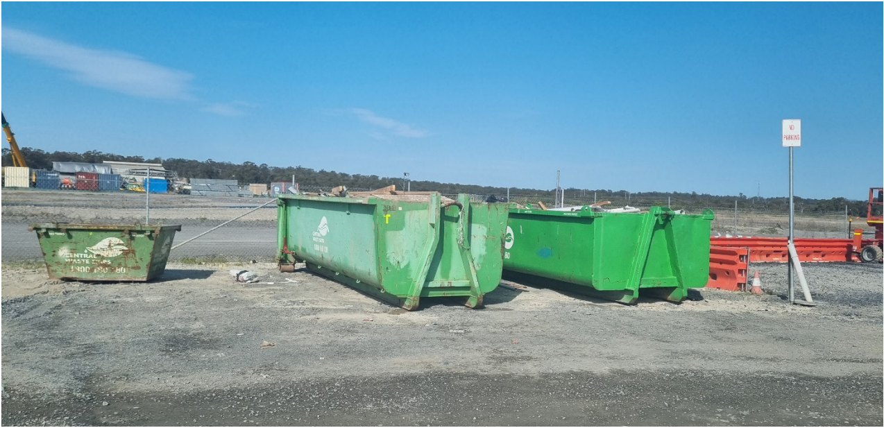
Photograph 11: Construction Waste Storage
