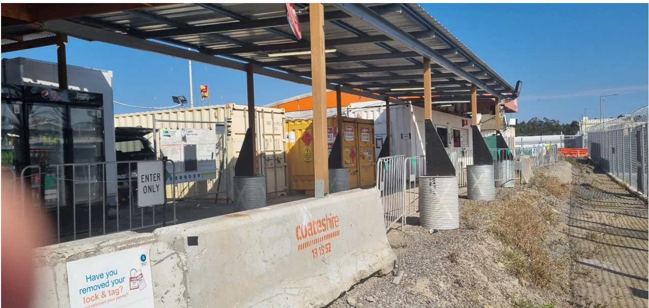
Photograph 10: Constuction Chemical Storage
