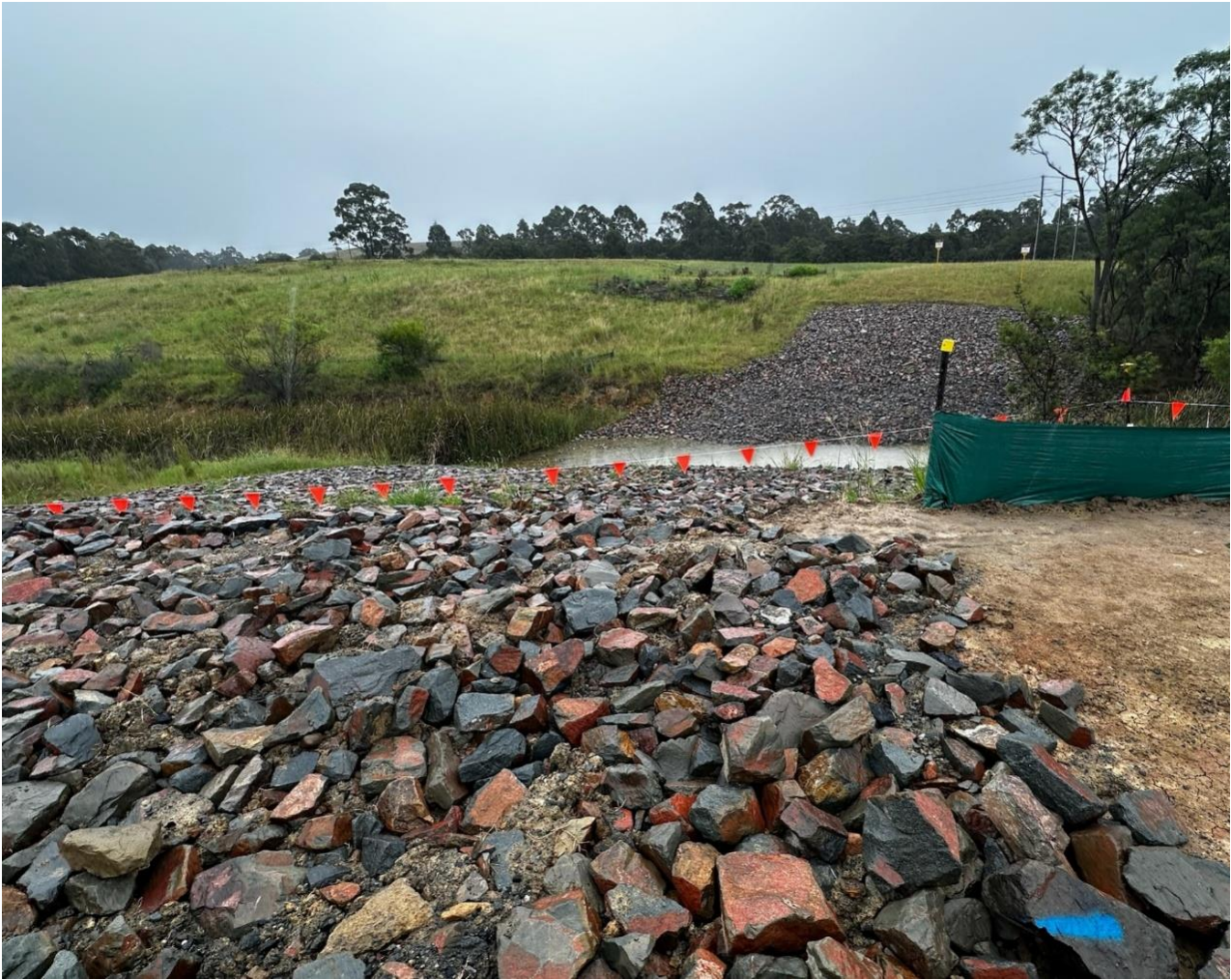
Photograph 6: Connecting gas pipeline rehabilitation and scour protection
