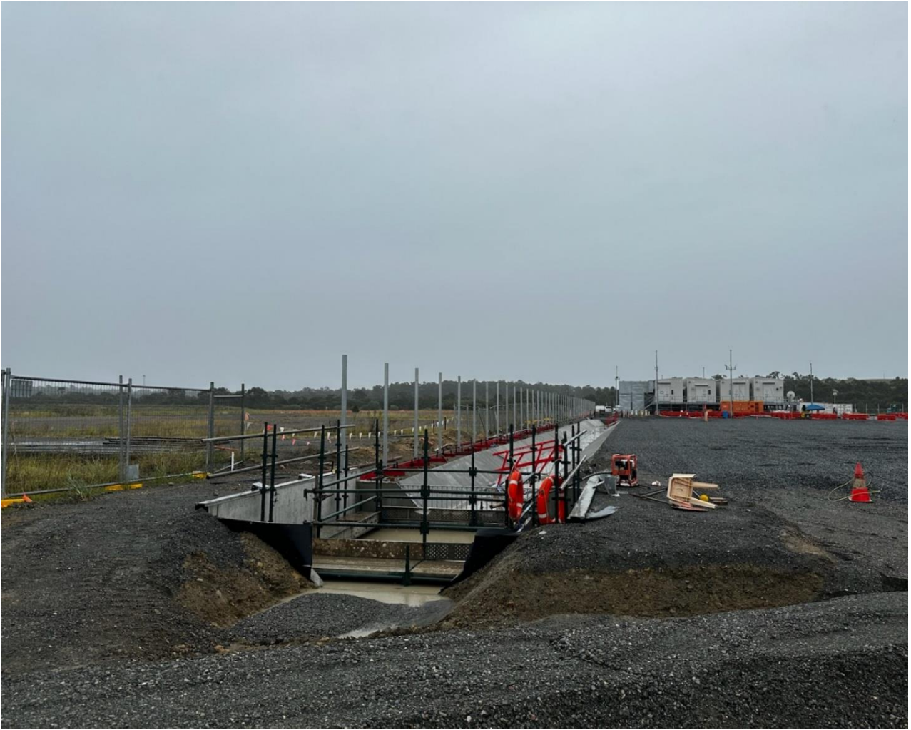
Photograph 15: Permanent perimeter drainage
