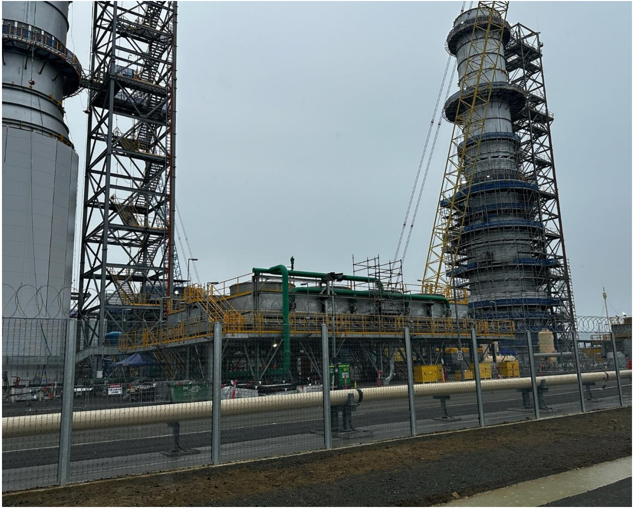
Photograph 1: Gas Turbine exhaust stacks under construction
