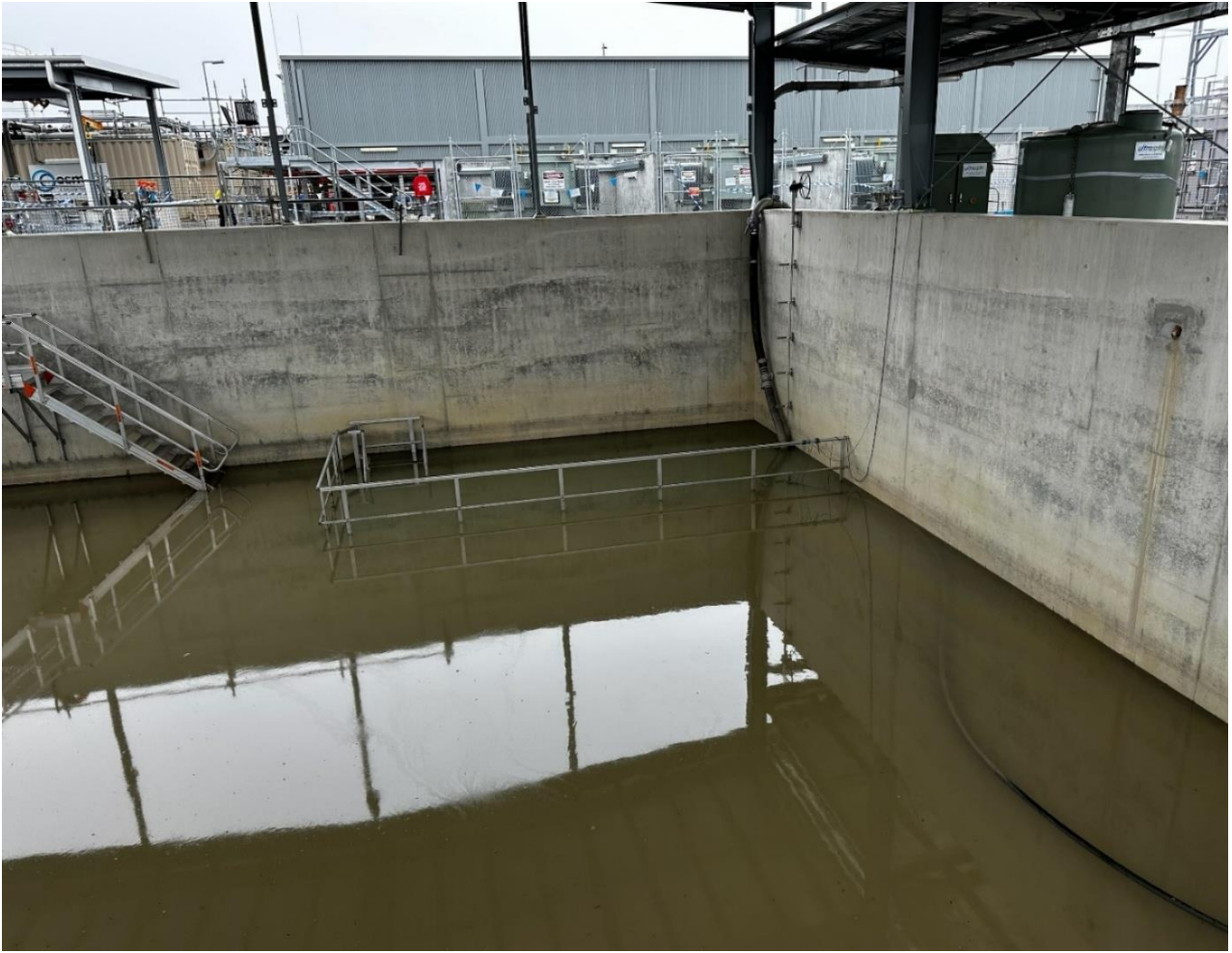
Photograph 8: Permanent oil pit interceptor utilised for site runoff
