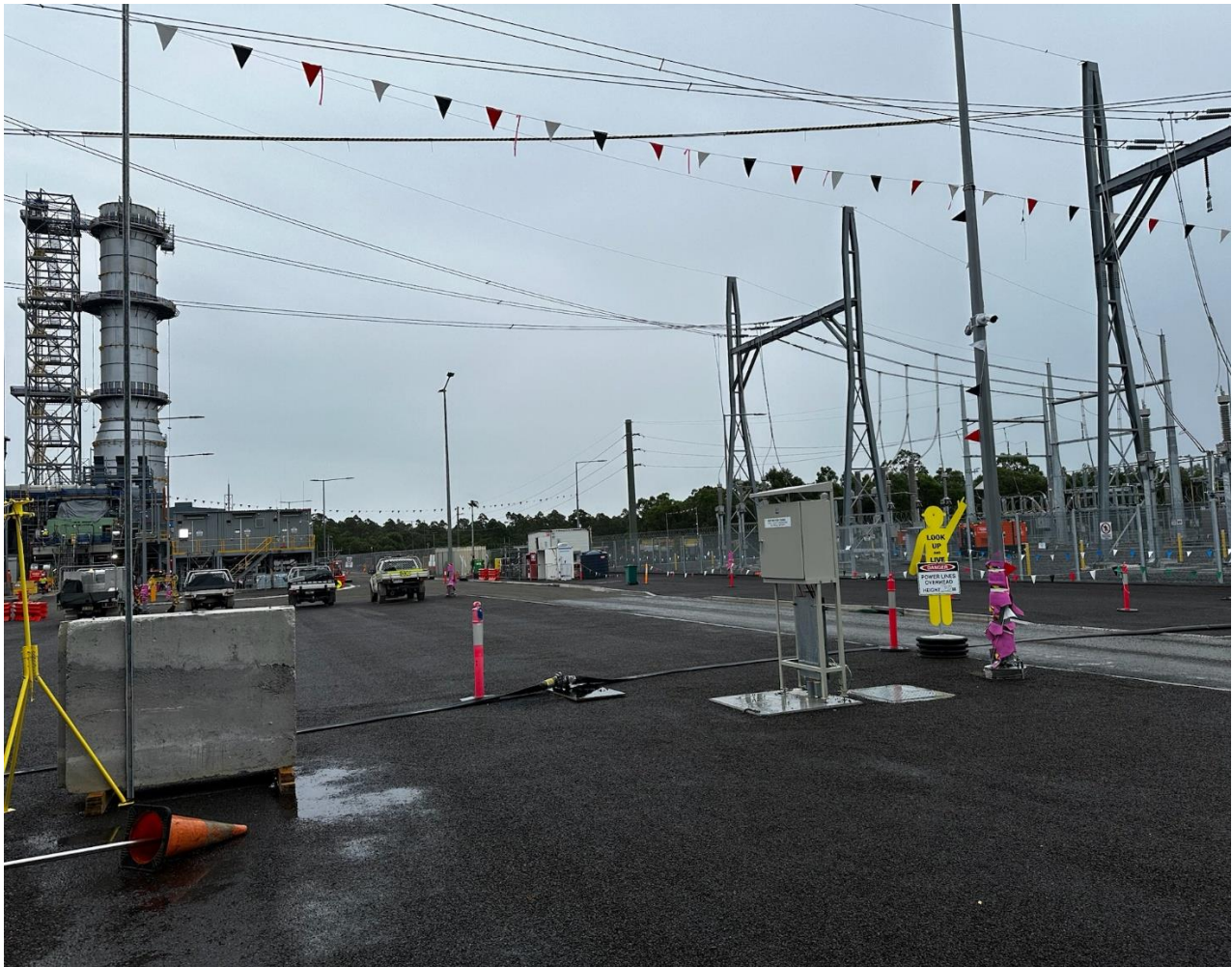
Photograph 2: Sealed hardstand, exhaust stack and power island
