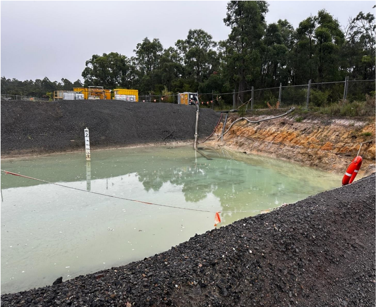
Photograph 9: Construction phase sediment basin (undergoing conversion to operational phase configuration)
