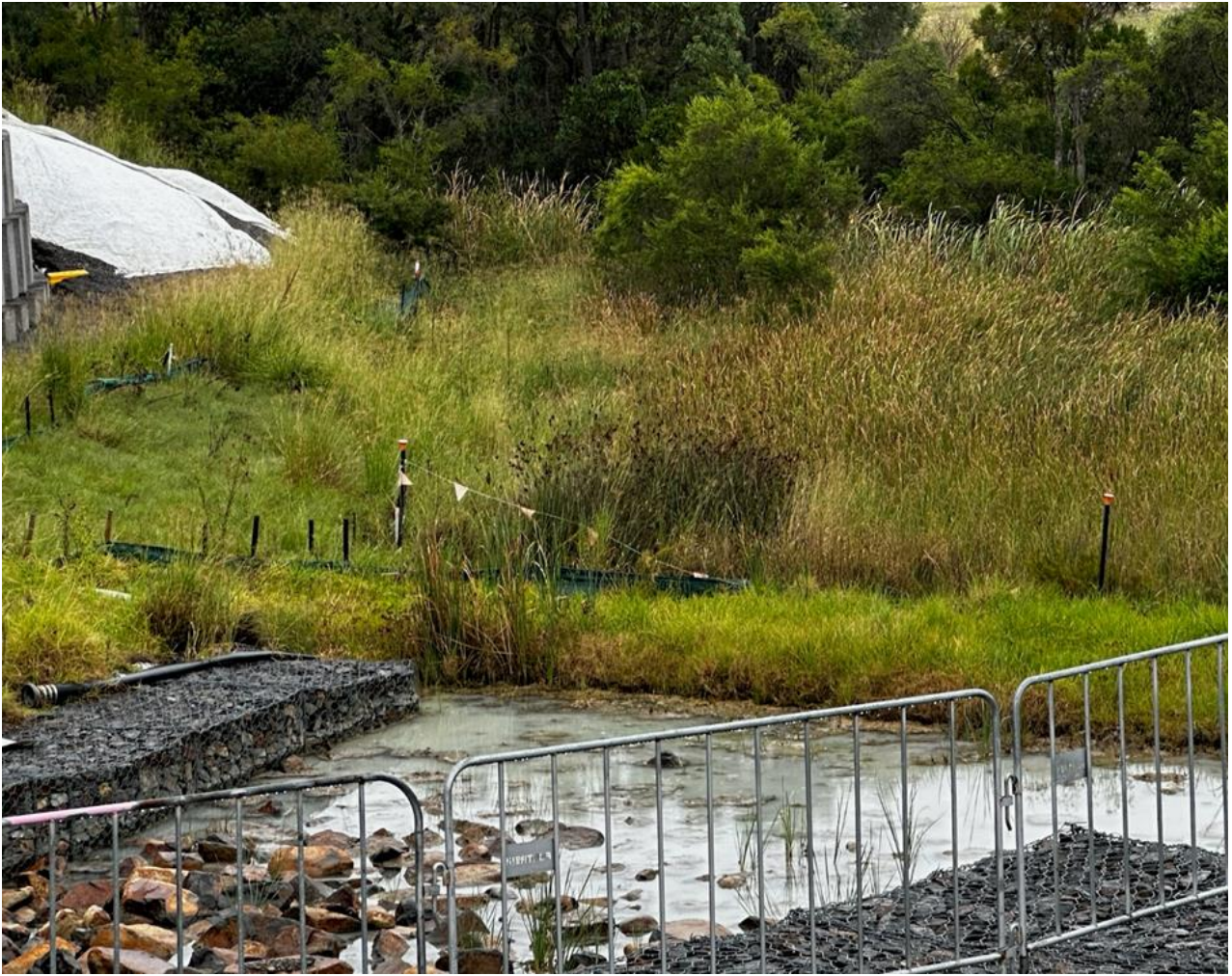
Photograph 11: Sediment basin outlet with operational features including rock scour protection installed
