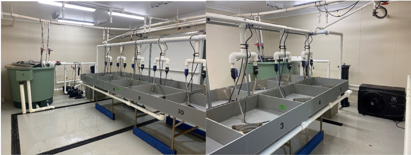
Figure 18. Incubation/larval rearing room at NFC including a heater/chiller unit that has been installed.
