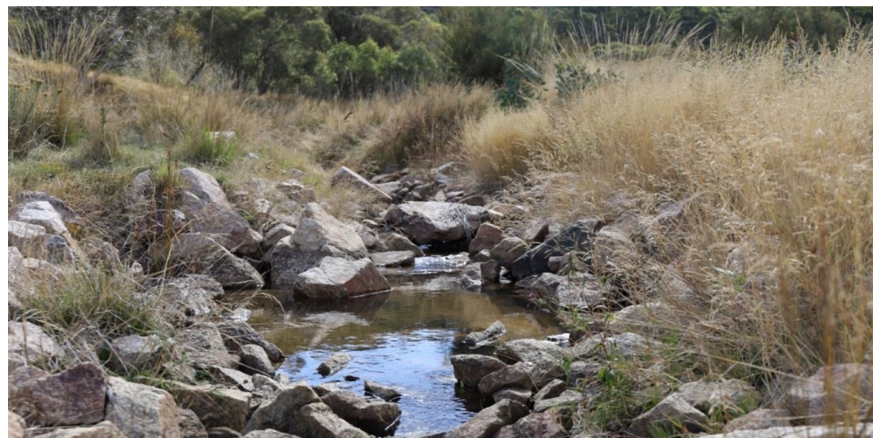
Figure 2 (d). Example of the constructed stream habitat at the Eucumbene Borrows (photo taken March 2023).
