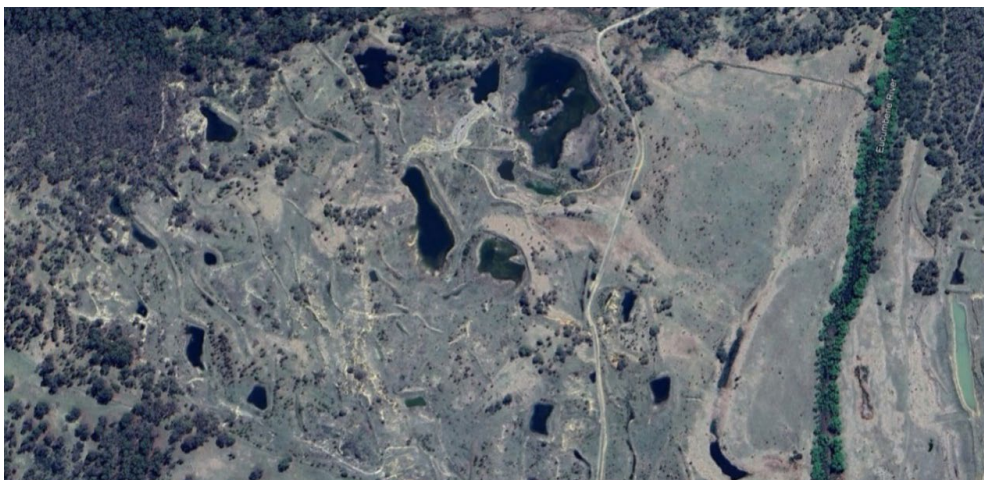
Figure 2 (a). Overview of the Eucumbene Borrows site (image taken October 2023).
