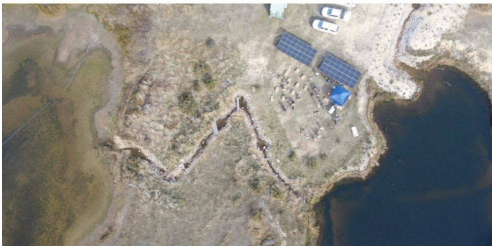
Figure 2 (c). Eucumbene Borrows lower constructed stream connecting the mid and lower ponds (photo taken March 2023).
