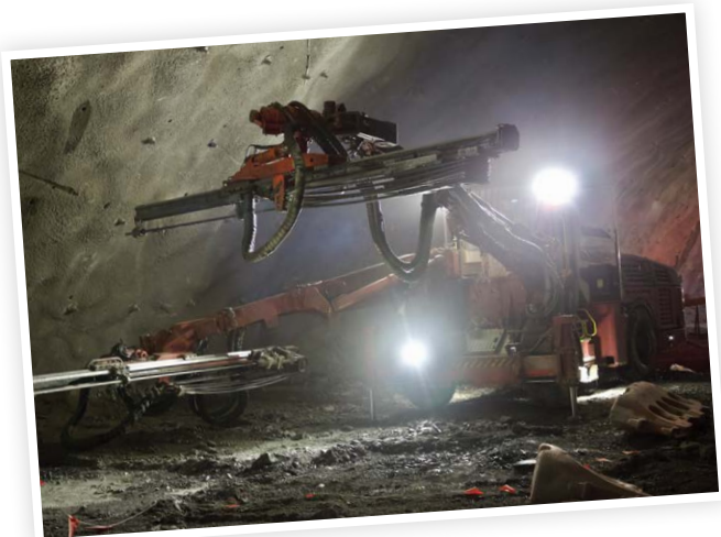
Drill and blast excavation in progress
