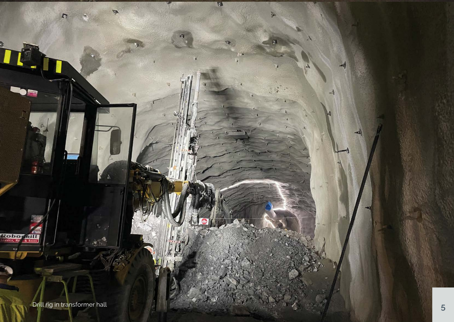
Workers at the Snowy 2.0 cavern excavation site
