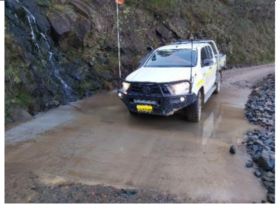
LH 45 and LH 46 Section of gravel road sealed with concrete and stabilised with rock on low side of LHRR North
