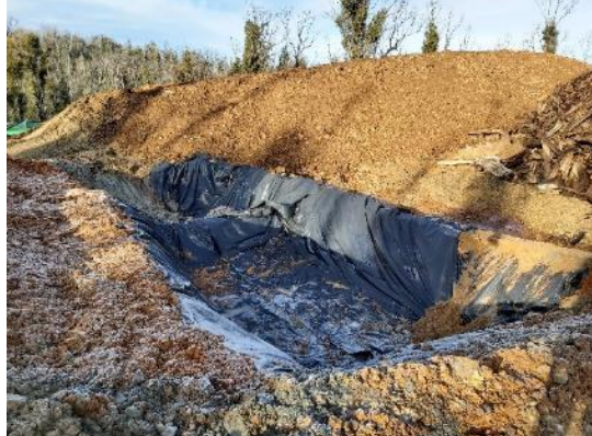
MC19: Concrete washout area – Marica West trail
