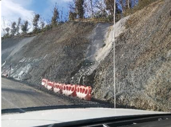
MC20: Marica Trail – “blind corner” stabilised batter
