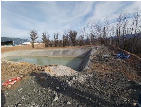
MC38: Leachate basin below temporary spoil area
