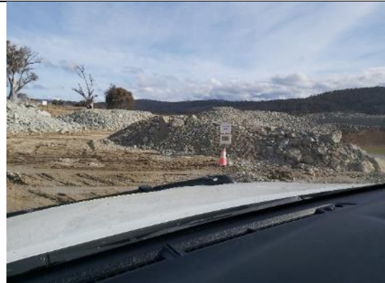
TT45: Concrete washout point in temp spoil area (with signage). Removed since inspection – not to go into the emplacement area.
