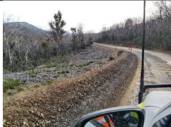
TT2: Tantangara – stabilised berm on road edge
