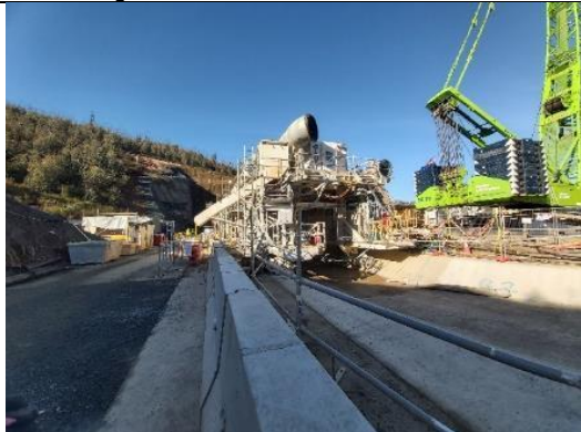
LH 37: TBM cradle and attaching gantries to the TBM Talbingo Adit
