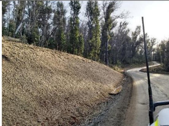
TT1: Tantangara road – Hydromulched batter
