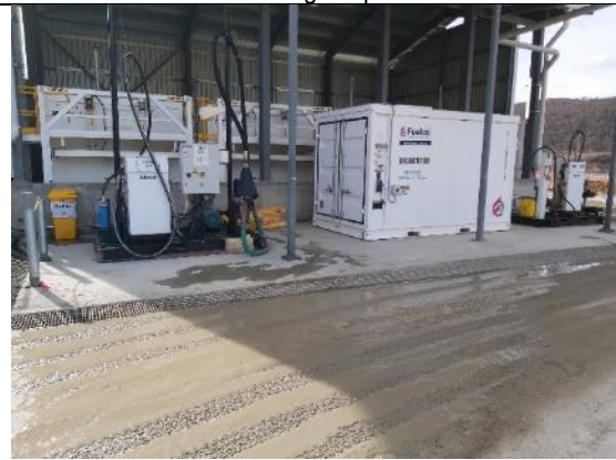
TT29: Fuel Farm. Sumps around storage and filling area
