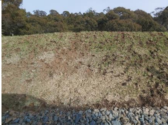
TT11: Hydromulched stabilised batter – damage by brumbies
