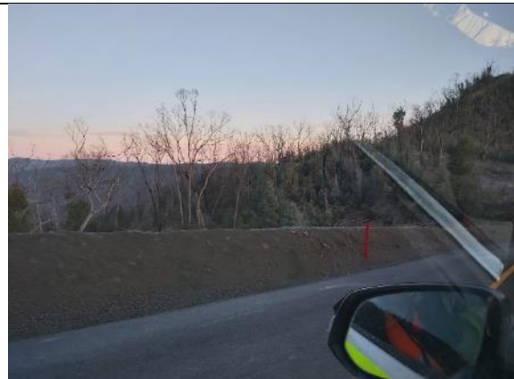
LRR 12: Roadside berm treated with "Stonewall" to stabilise
