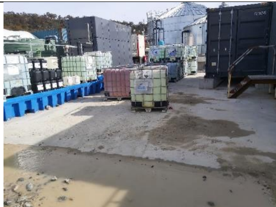
TT30: Water treatment Plant chemical storage – not fully bunded – one side open.
