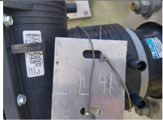
LH 42: EPL point correctly labelled on apparatus
