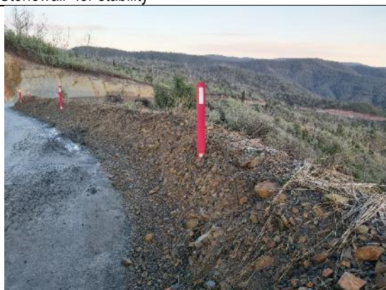
LRR 15: Roadside berms – treated with Stonewall
