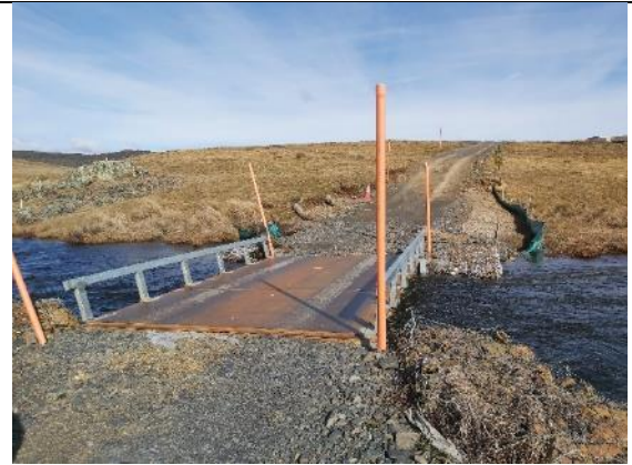
GTS16: Tantangara Creek – Gabion baskets installed to limit scour on the creek banks, stabilised road verges with jute mesh, coir logs and sediment fencing
