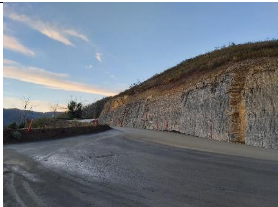
LRR 13: Lay-bye with stabilised berms – treated with "Stonewall" for stability
