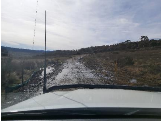
GTS11: Sediment controls on track edge – controlling water from natural springs. Further sediment controls may be required in areas inundated with natural spring water.
