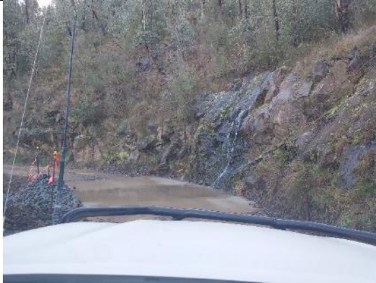
LH 45 and LH 46 Section of gravel road sealed with concrete and stabilised with rock on low side of LHRR North
