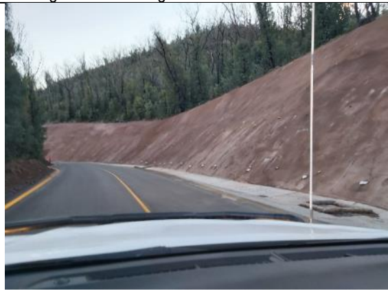
LRR 11: Stabilised / shotcreted rock face. Road pavement fully sealed (from gatehouse to site).
