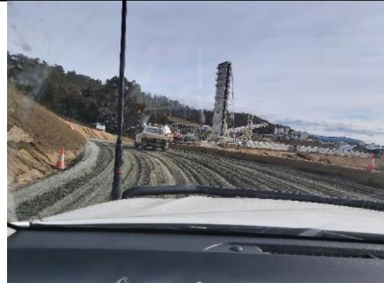
TT23: Quarry Trail Road – Tantangara Adit. Road sheeted with crushed rock
