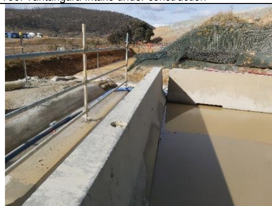
TT35: Water collection system around the gate shaft
