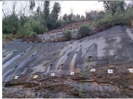
LRR 10: Stabilised / shotcreted rock face
