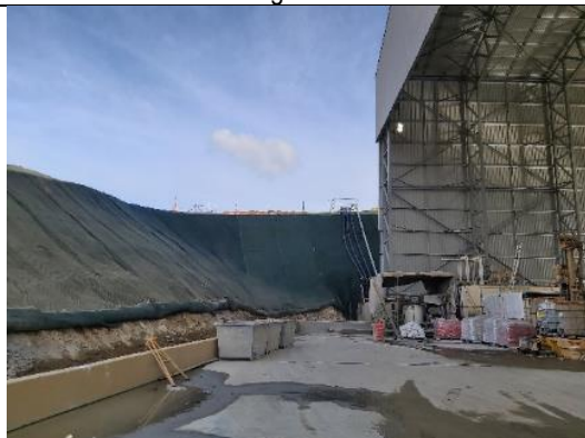
TT36: Plastic mesh used to stabilise embankment around the gate shaft
