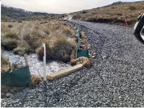
GTS9: Gooandra Creek crossing – sheeted with DGB
