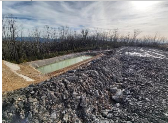
MC37: Temporary spoil area – material from the surge shaft stored for later use for land forming around the surge shaft when completed.
