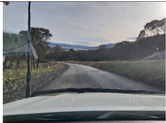
TT10: Hydromulched berms – germinated seeds. Road surface has been sheeted with crushed rock
