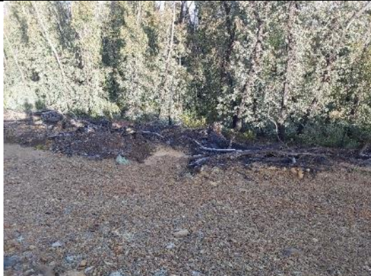
MC16: As previous photo – washout at base of batter.
