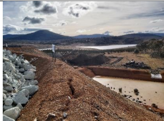
TT49: S1 spoil area – sediment basin
