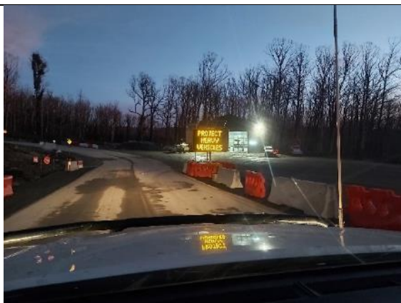
LRR 17 & LRR 18: Lobs Hole Ravine Road entry / exit – signage says Project Heavy Vehicles must maintain 500m between heavy vehicles (to prevent convoying – previously 250m)
