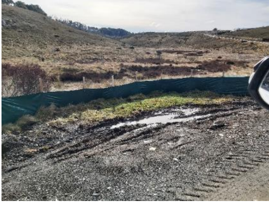
GTS7: Sediment fencing installed to capture surface water runoff
