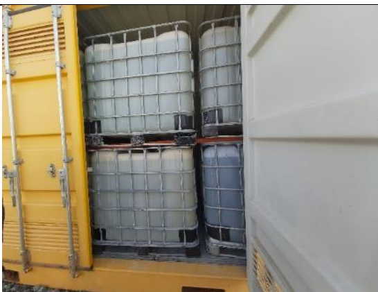
TT32: Chlorine storage inside container
