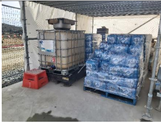
TT20: Pallet load of drinking water for the Camp. Waste cooking oil tank (valve positioned outside bund – ineffective for spill containment)
