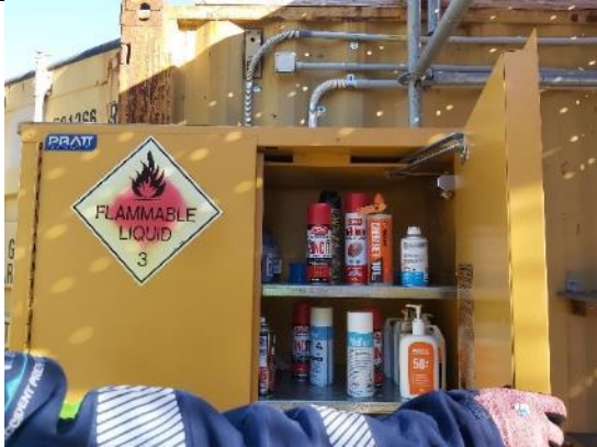
LH 39: Minor DG and Hazardous substances storage at Talbingo Adit. Incompatible storage (class 2 gas and class 3 liquids, signage incorrect), see NC on general chemical management
