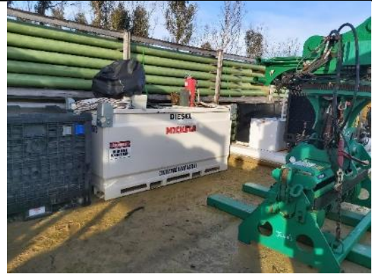
MC17: Diesel storage at HDD pad – double skinned tank
