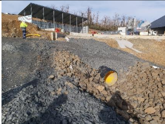
MC36: Part of upgrade of surface water controls below the surge shaft
