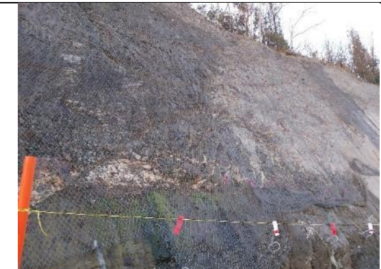
MC9: Batter stabilisation – wire mesh
