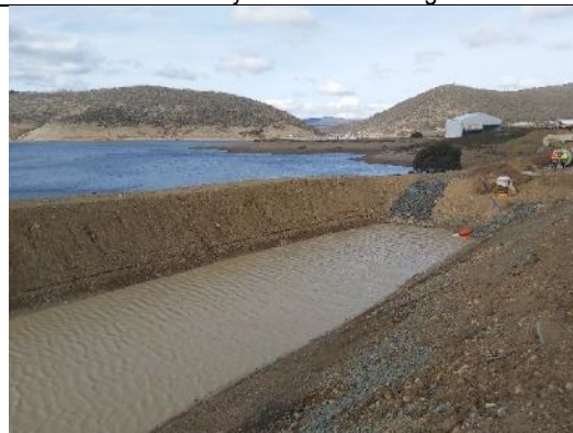
TT37: Upgraded sediment basins (S2) along Spoil Road.
