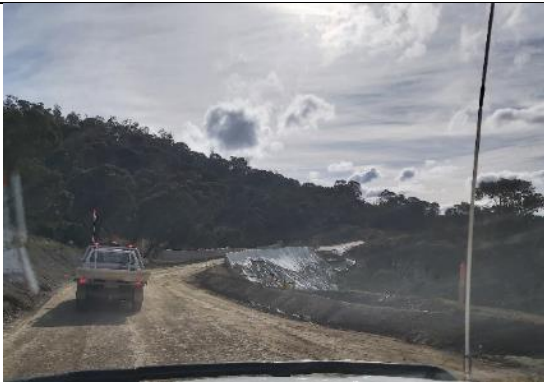
TT40: Additional erosion and sediment controls installed along Spoil Road to prevent splash of sediment to the creek line
