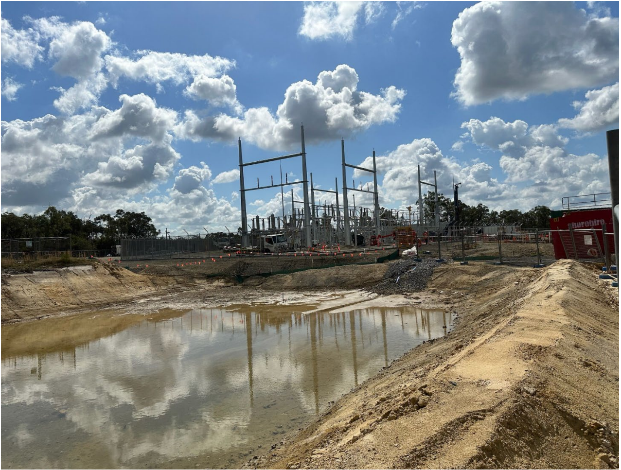
Photograph 4 – Sediment basin and switchyard
