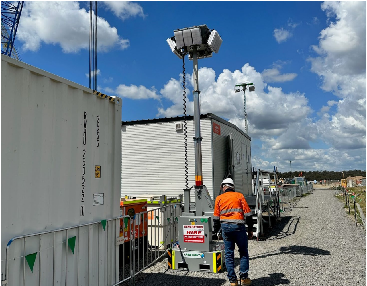
Photograph 12 – Temporary mobile lighting utilised for night works
