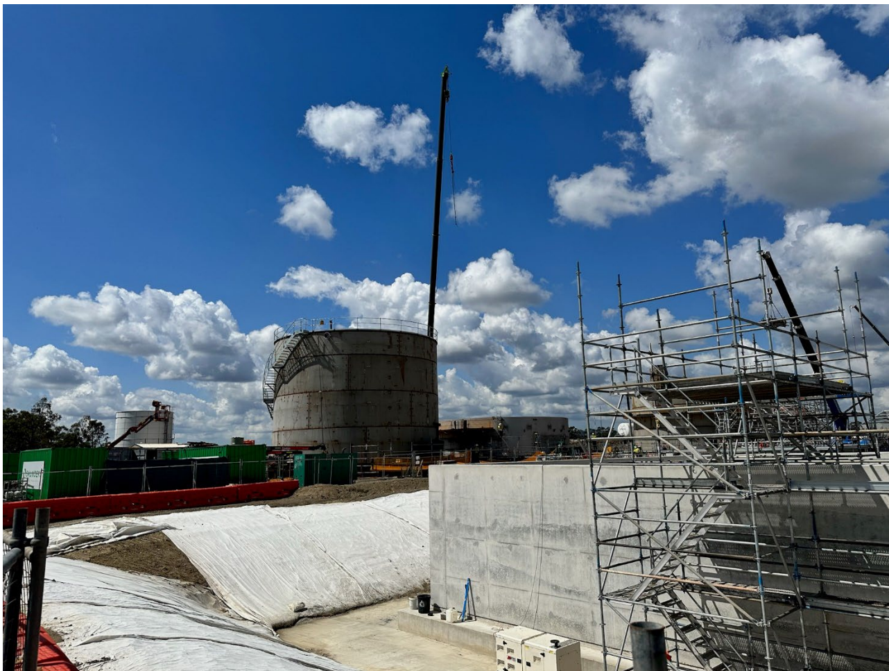
Photograph 1 – Construction of amenities building and tank farm
