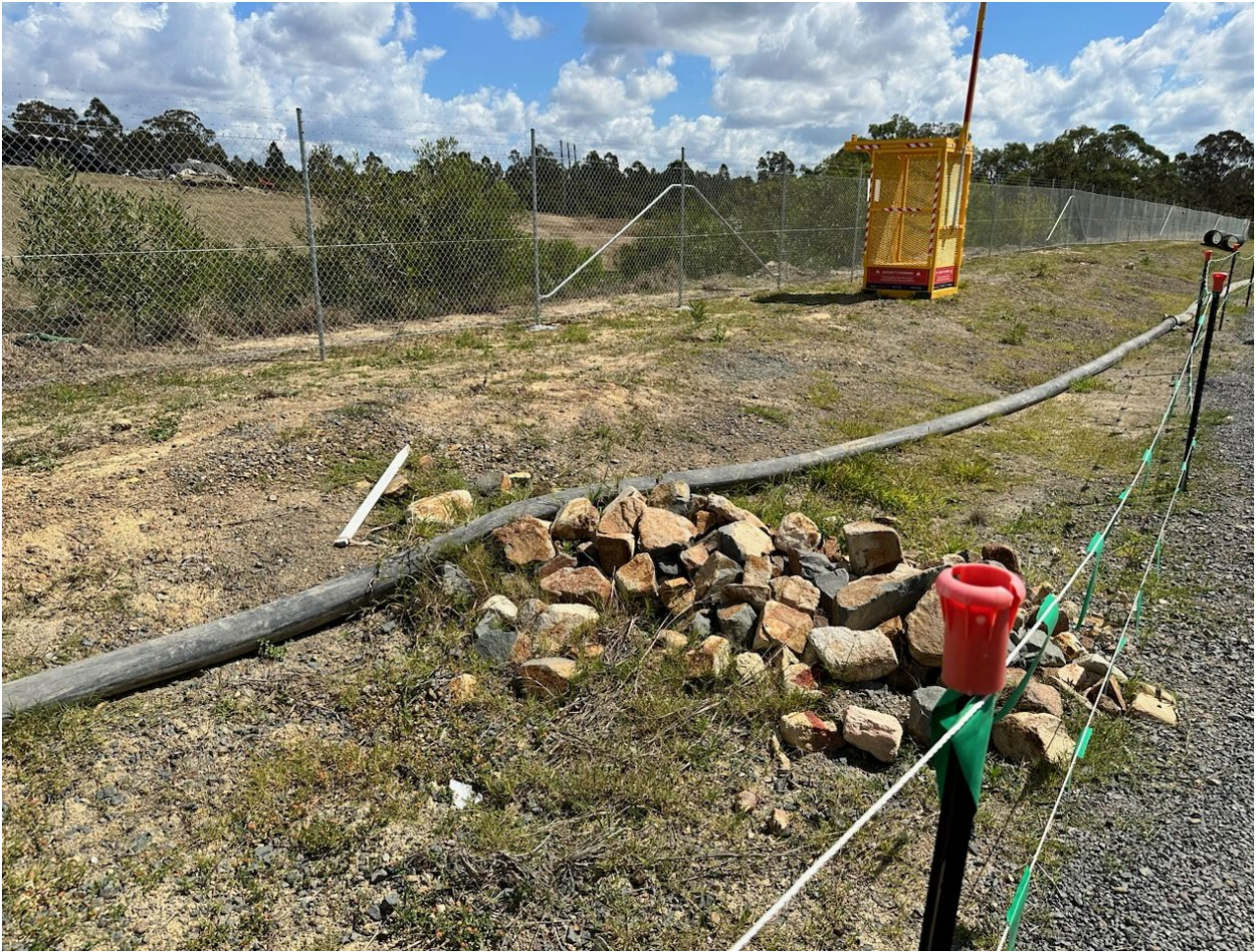
Photograph 10 –Perimeter bund and rock check
