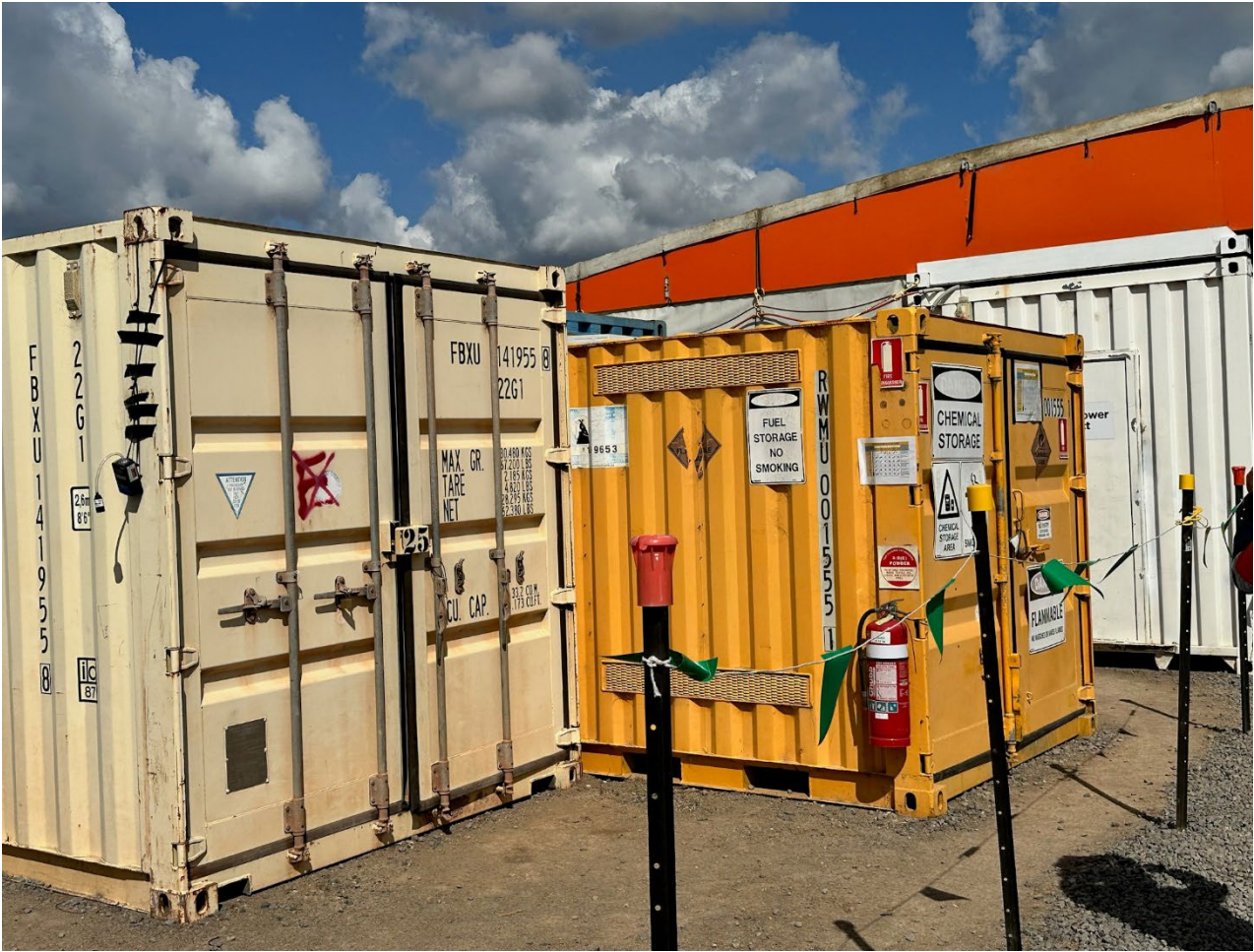
Photograph 2 – Ventilated and banded chemical storage container
