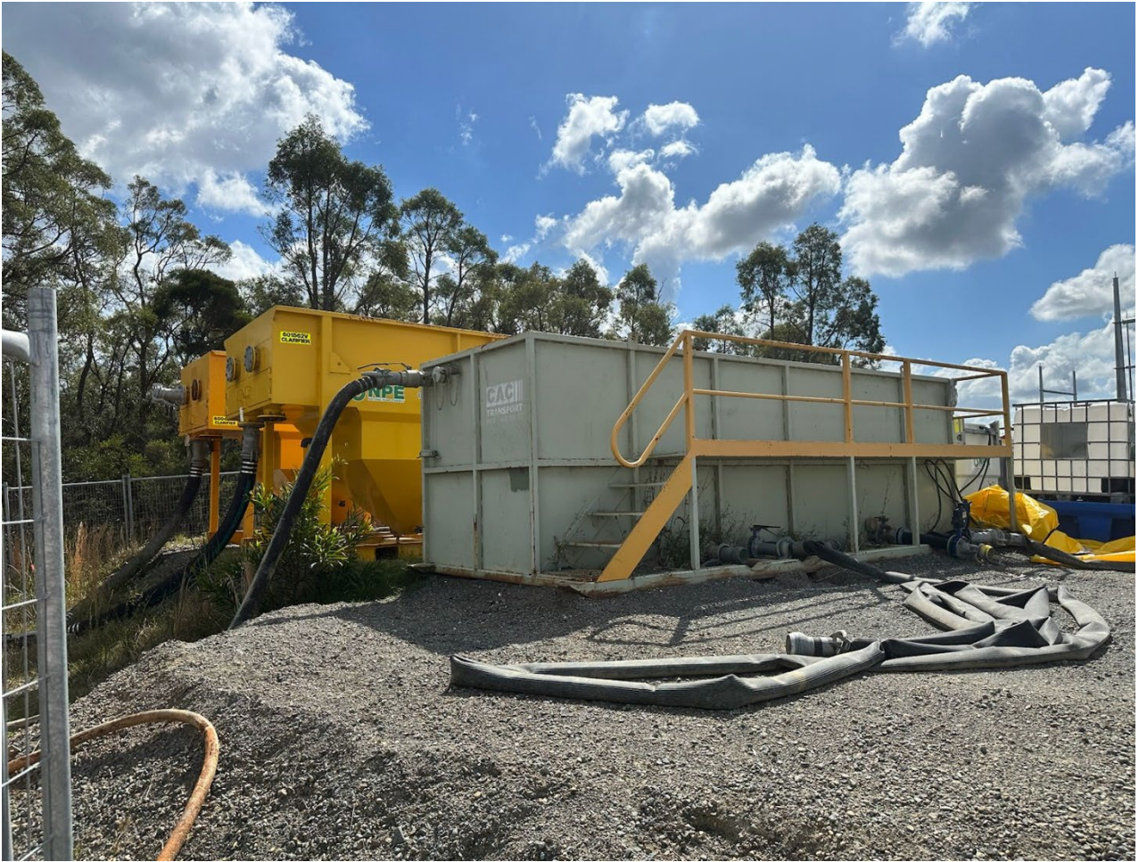
Photograph 9 – Site water settlement container
