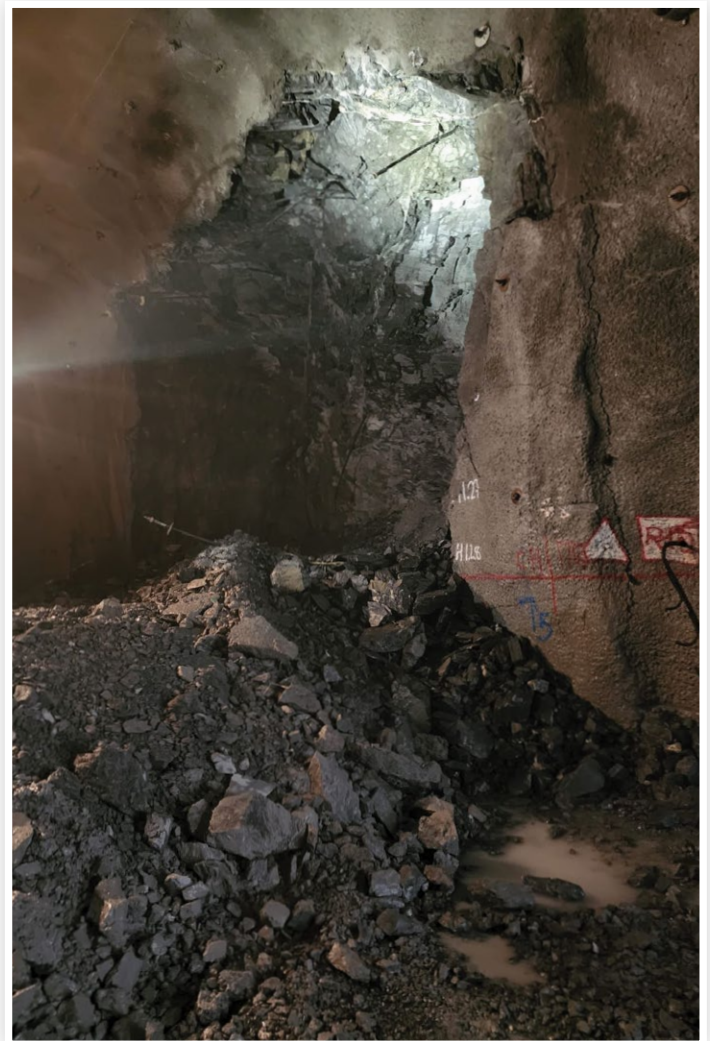
First opening of the transformer hall cavern crown
