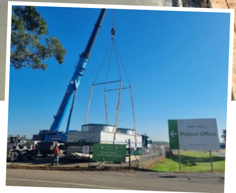
Giant fin fan coolers arriving on site
