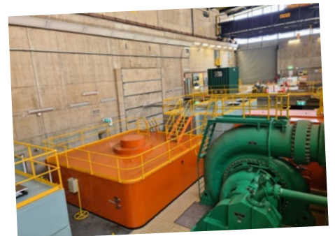
Above and below: Permanent edge barriers help protect workers from falls
