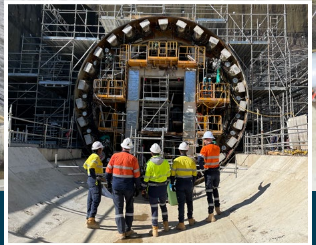
TBM Lady Eileen assembly at Talbingo adit
