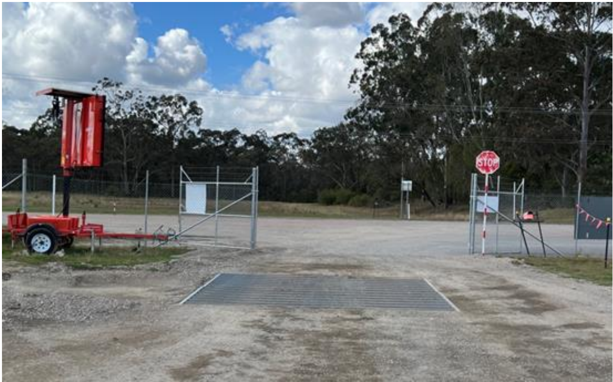
Photograph 3 - Rumble Grid at site entrance
