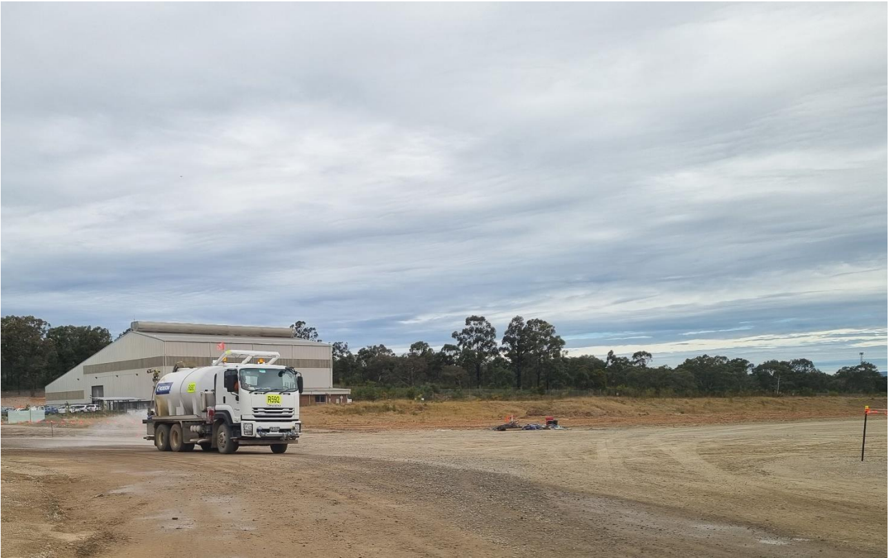
Photograph 1 - Water cart in operation
