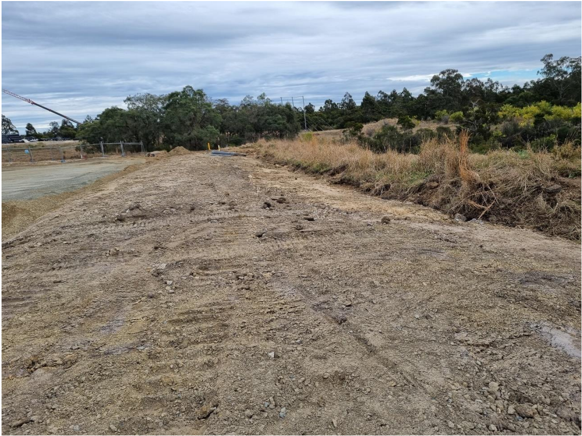
Photograph 6 - Site boundary contouring to divert run off into sediment pond.
