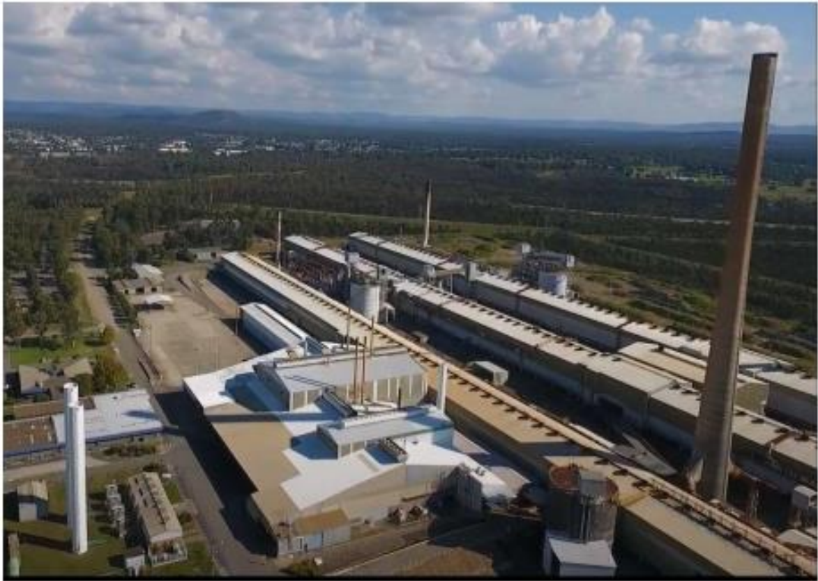
Figure 1.4: Precinct 3B prior to demolition in 2019
