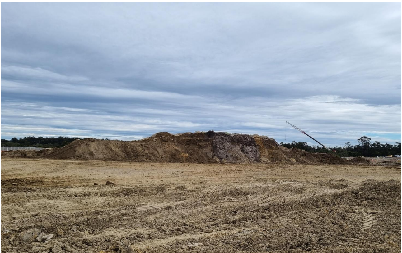
Photograph 2 - Excavated Material Stockpile
