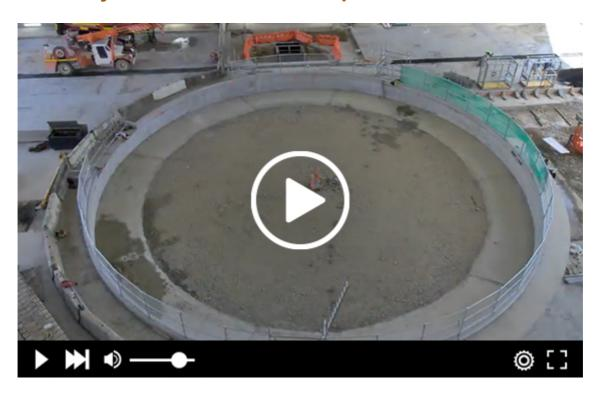
We're full speed ahead with construction of the upstream surge shaft at Marica.In this time lapse video taken from our 28 metre-high shed, you can see preparation works for the construction of the shaft and the start of excavation. The yellow structure at the end of the video will be used to transfer rock from the kibble into the 30-tonne articulated dump trucks for removal.
