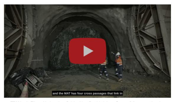
TBM Lady Eileen Hudson has finished her first big job on Snowy 2.0, excavating the 2.85 kilometre main access tunnel. The MAT, as it's known, gives us access to the site where we'll excavate the 2 enormous caverns about 800m underground that will house our power station. This tunnel is 10 metres in diameter and it's lined with almost 13,000 concrete segments manufactured locally at our precast plant in Cooma. This is a great tunnelling achievement for our Snowy 2.0 teams!
