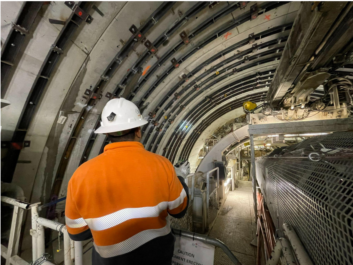
On TBM Florence
