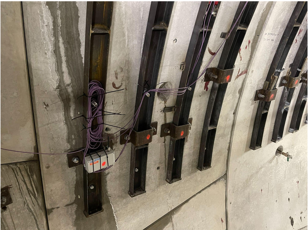
Instrumentation to monitor ground performance
