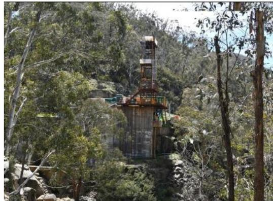
In a remote part of the Snowy Mountains, Snowy Hydro and its contractors have been carrying out complex and important improvements to a 125-metre deep intake shaft. The Burrungubugge intake shaft is a critical part of the Snowy Scheme, diverting water from the Gungarlin and Burrungubugge rivers into the Snowy-Eucumbene tunnel directly below.
