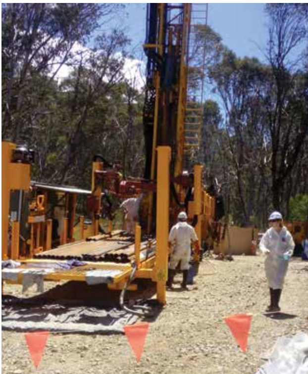
Drilling as part of the geotechnical investigation
