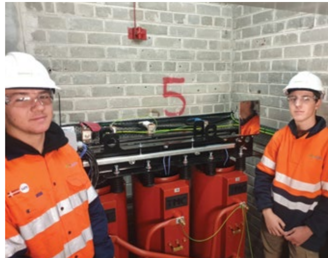
Blair Tracey and Nick Holloway standing with a new dry-type transformer after it was fitted into place in readiness for electrical connection to Tumut 2 Unit 5 Generator
