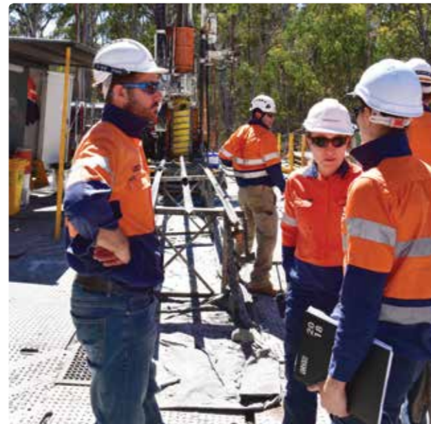
Staff at a Snowy 2.0 investigative drill site
