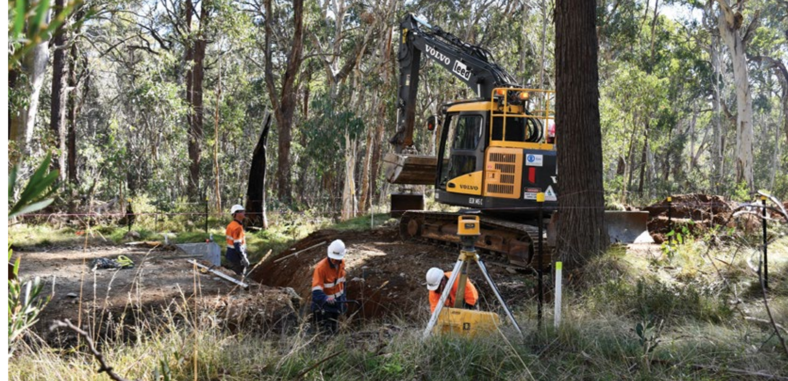
Lobs Hole Ravine Road drainage work
