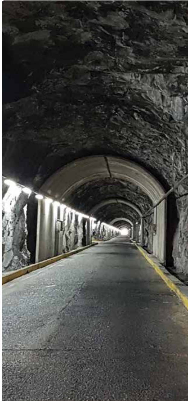
Tumut 2 Power Station access tunnel
