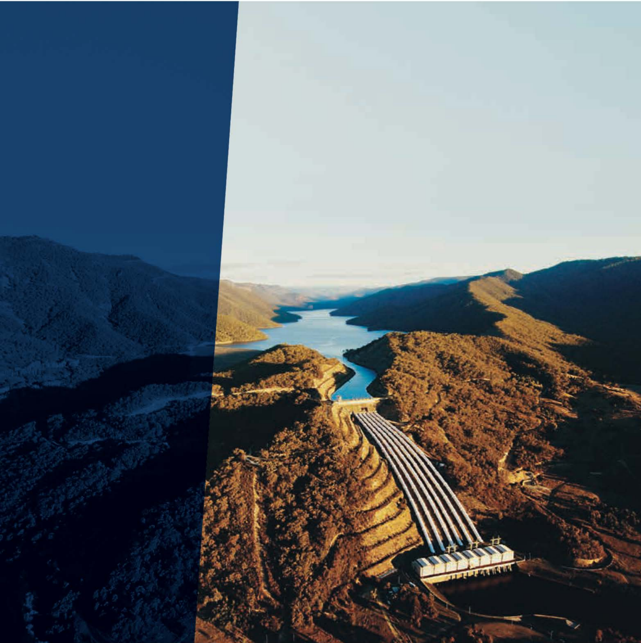
Tumut 3 Power Station
