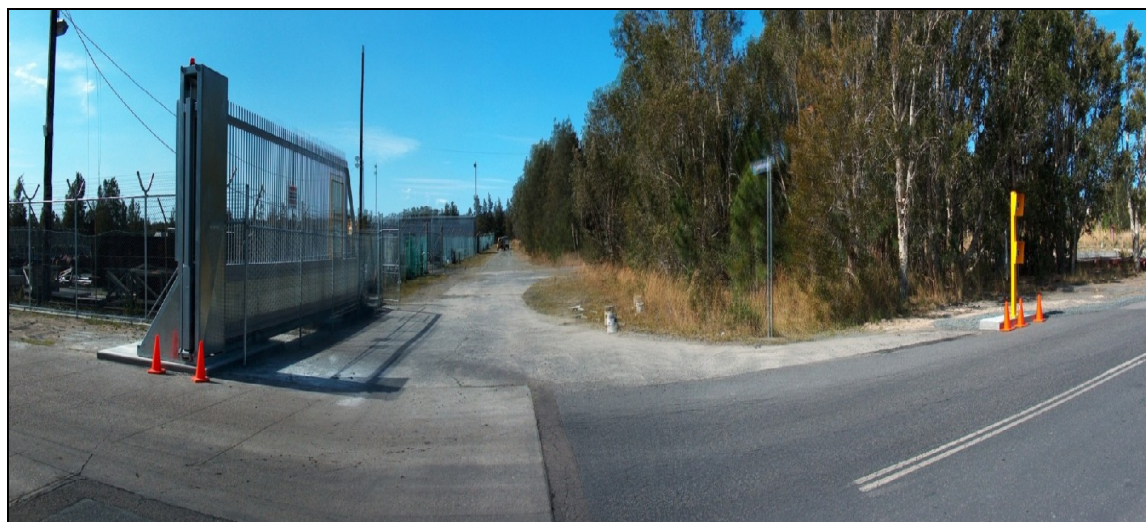
Photograph 5.1: OCGT peaking plant, facing NE
