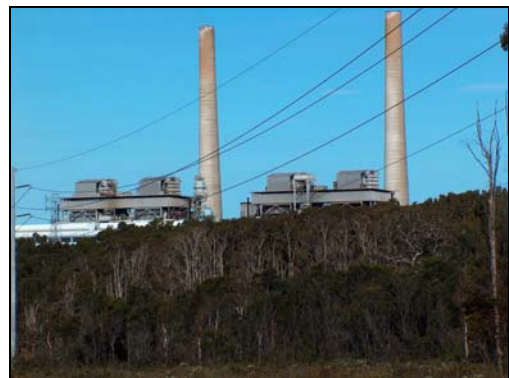
Proposed Gas Turbine Facility Munmorah Power Station
