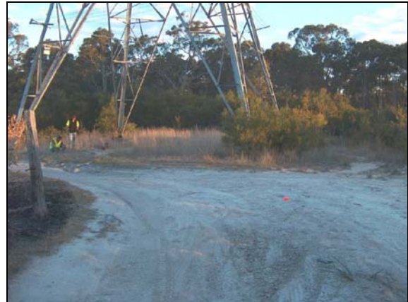
Photograph 5.14: 21TL15, the location of AS2, looking South
