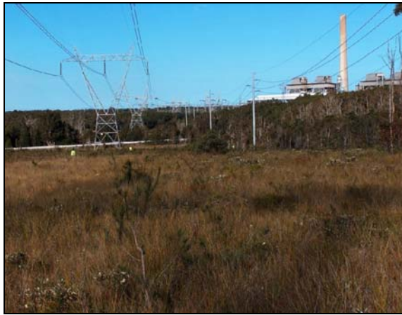
Photograph 5.3: Area B, looking towards the power station, facing East
