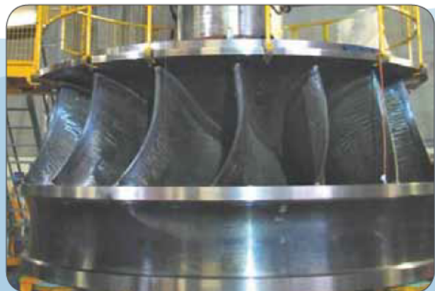
The new runner being installed at Tumut 3, the increased curve provides better efficiencies.
