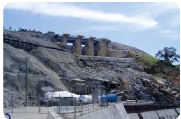
A concrete apron and training walls will connect the existing spillway to the new outlet works.
