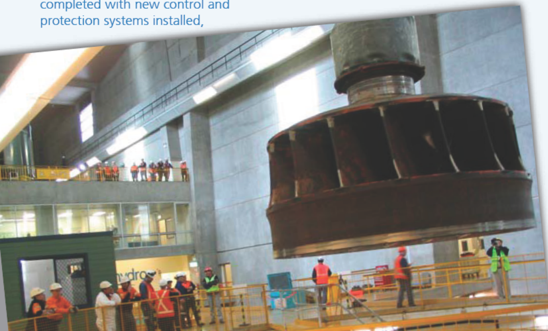
Left: The removal of a runner at Tumut 3.
