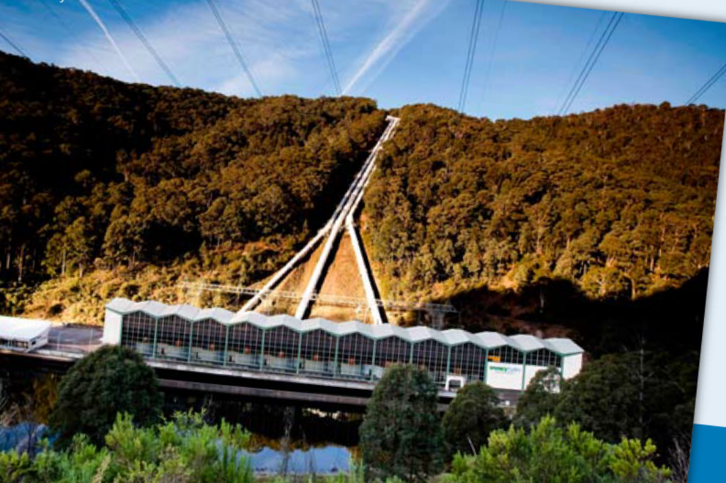
Murray 1 Power Station
