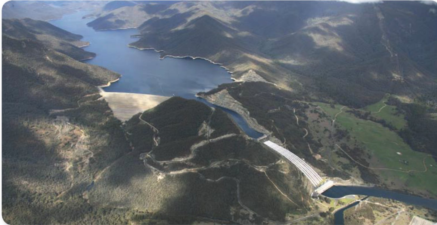
Talbingo Dam, Reservoir and Tumut 3 Power Station
