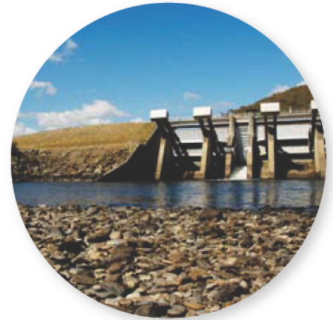
Khancoban Dam Release Gates
