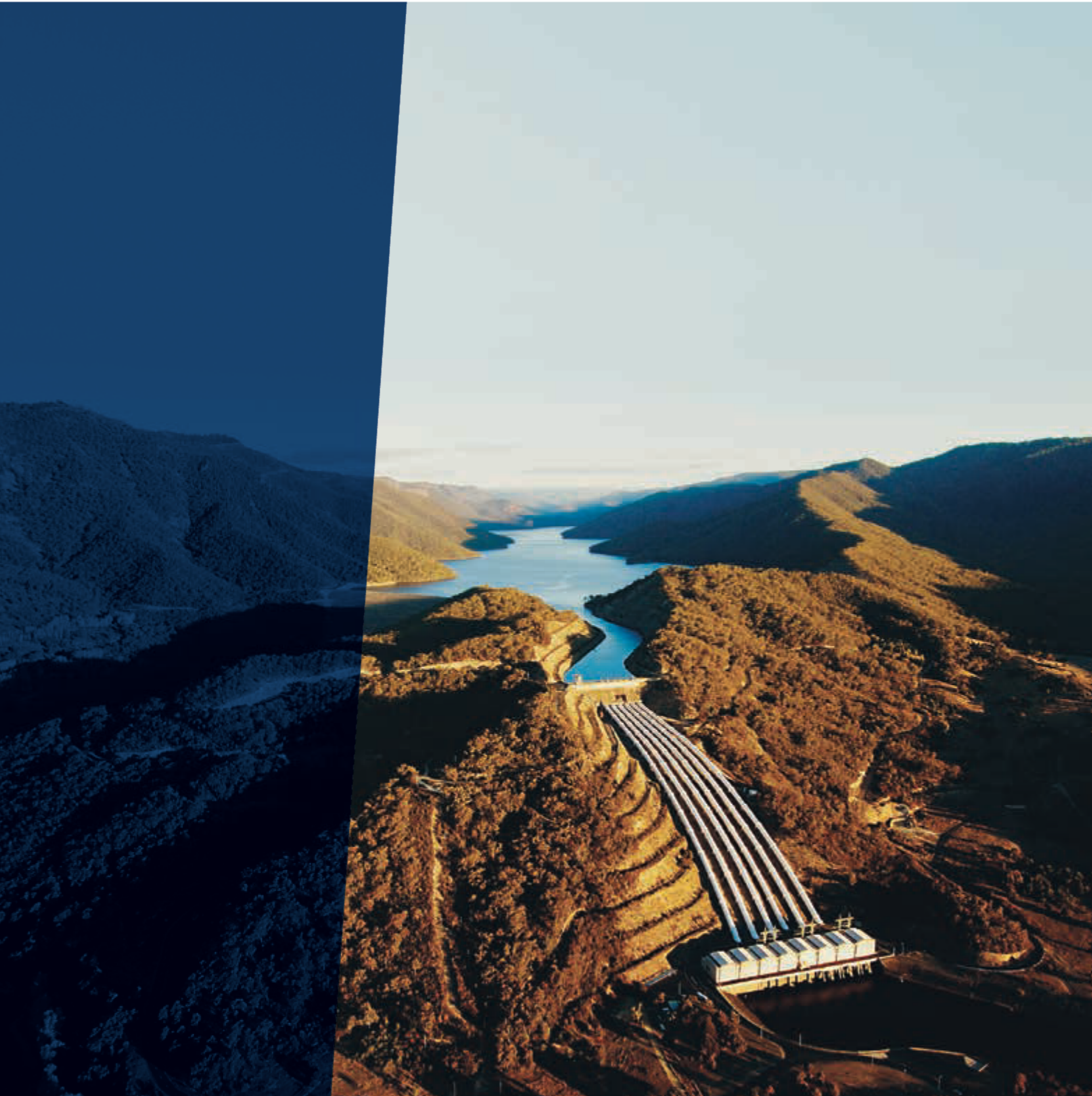
Tumut 3 Power Station
